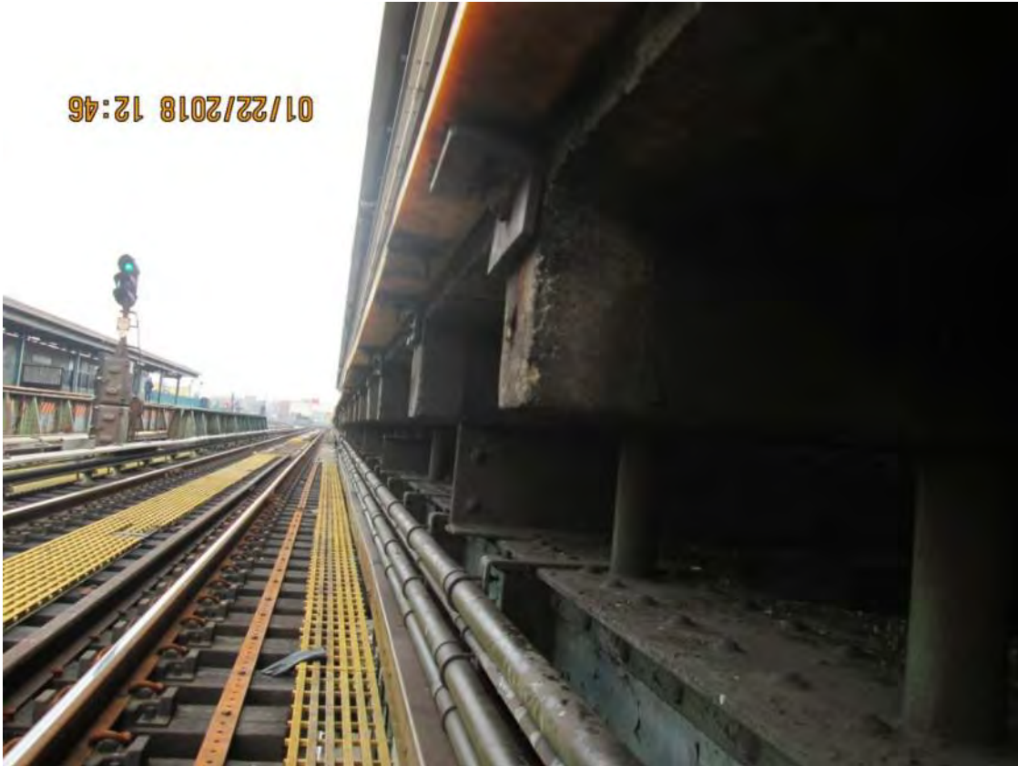
Figure 2 – Precast T-Beam platform – 103rd Street-Corona Plaza Station
