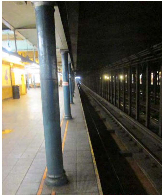
Figure 1 – Column 18” from the edge 50 th Street Station
