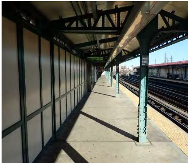
Figure 1 – General Station Condition Whitlock Avenue Station
