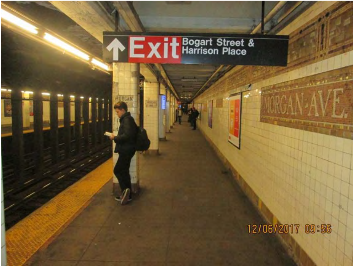
Figure 3– Typical Platform View – Morgan Avenue Station
