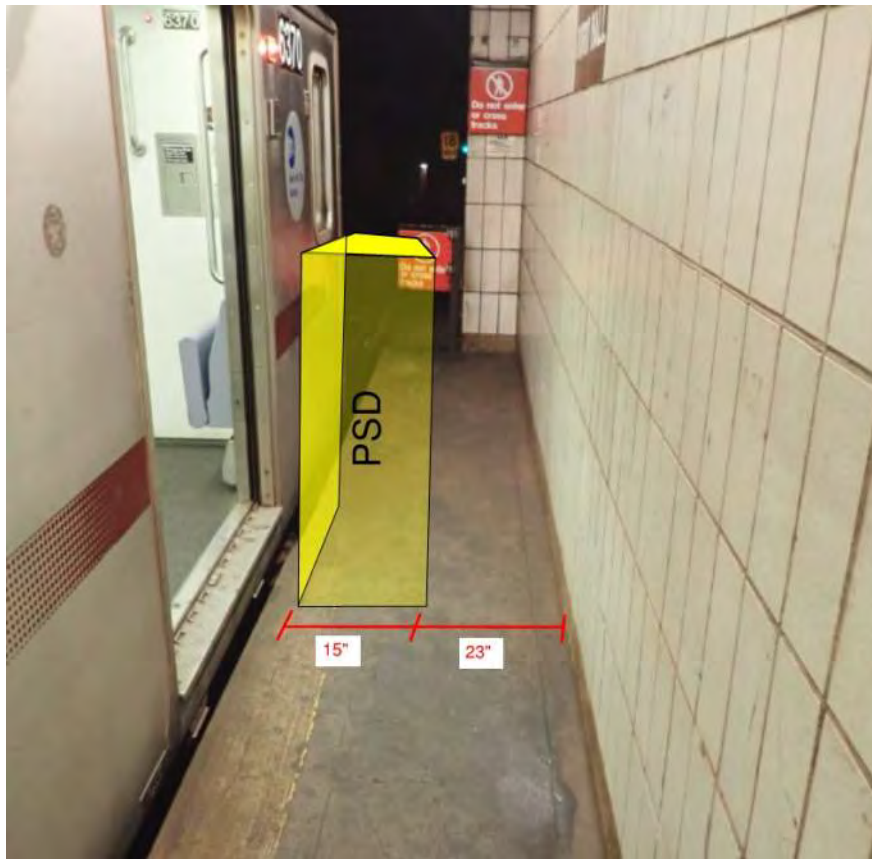
Figure 1 – Non-compliant ADA condition Borough Hall Station
