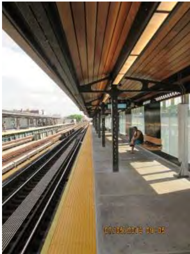
Figure 1 – Overall view 36 th Avenue Station
