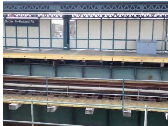
Figure 2 – Precast Slab Sutter Avenue Station
