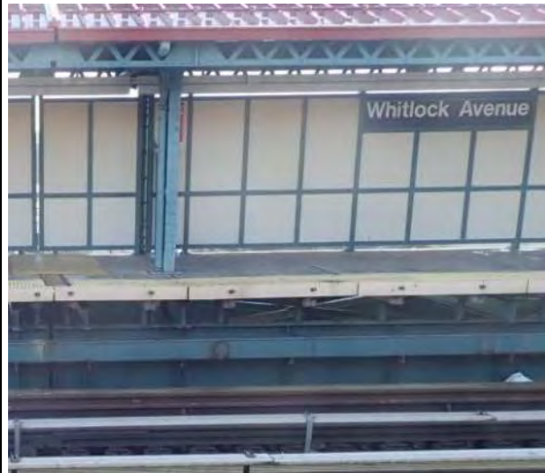
Figure 2 – Precast Slab Whitlock Avenue Station
