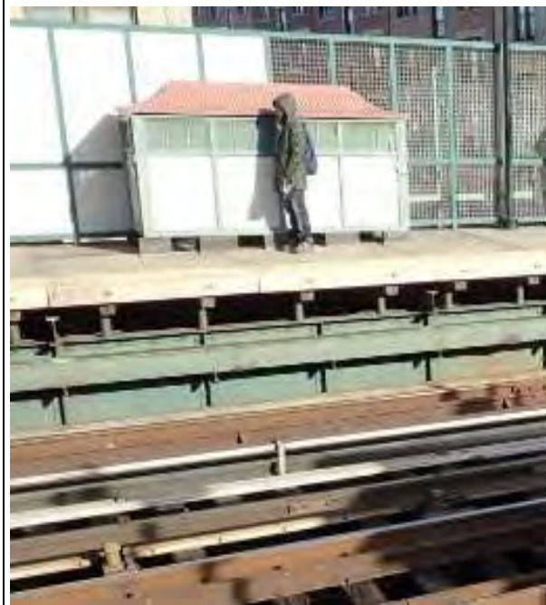
Figure 2 – Precast Slab Elder Avenue Station
