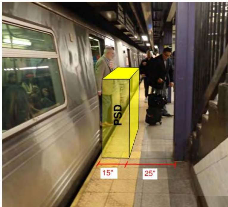
Figure 1 – Non-compliant ADA dimension Chambers Street Station
