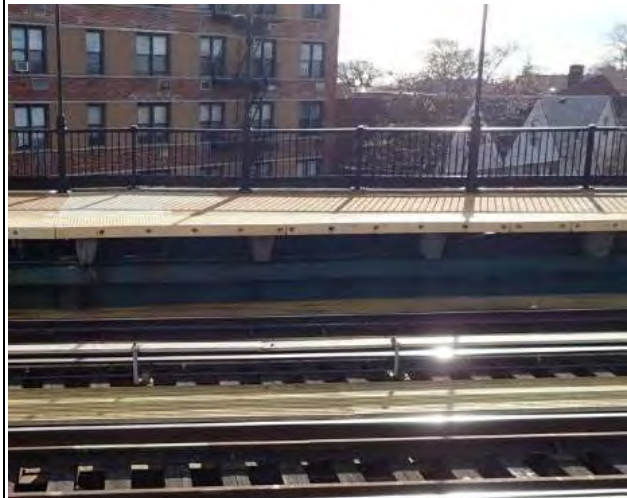
Figure 2 – Precast Slab Buhre Avenue Westchester Avenue Station
