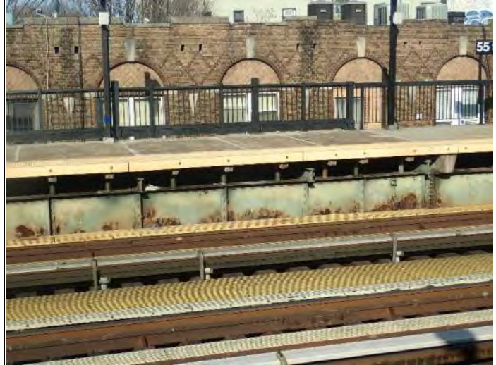
Figure 2 – Precast Slab 55 th Street Station
