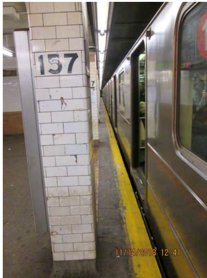
Figure 1 – Column 1'-2" from the edge 157 th Street Station
