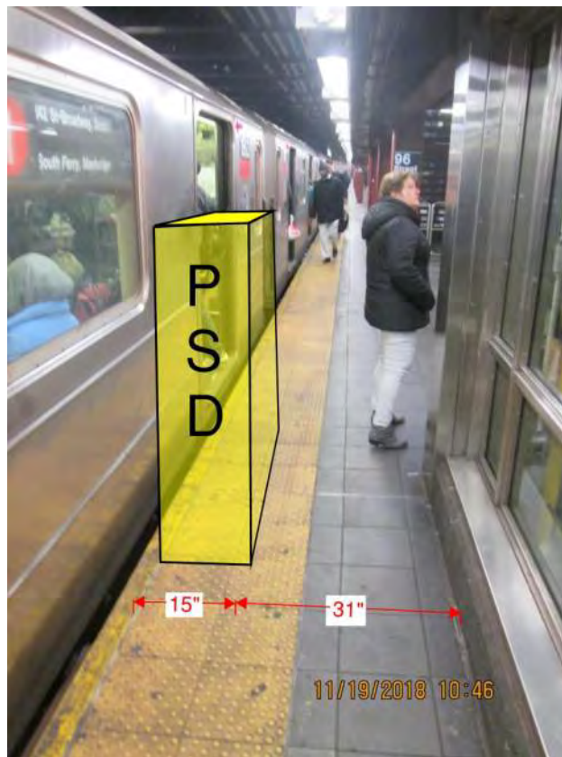
Figure 1 – Non-compliant ADA condition 96 th Street Station
