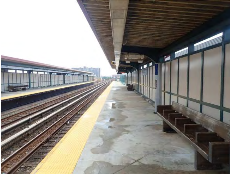
Figure 3 – General platform view Beach 105th Street Station
