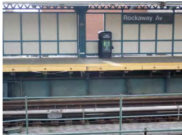
Figure 2 – Precast Slab Rockaway Avenue Station
