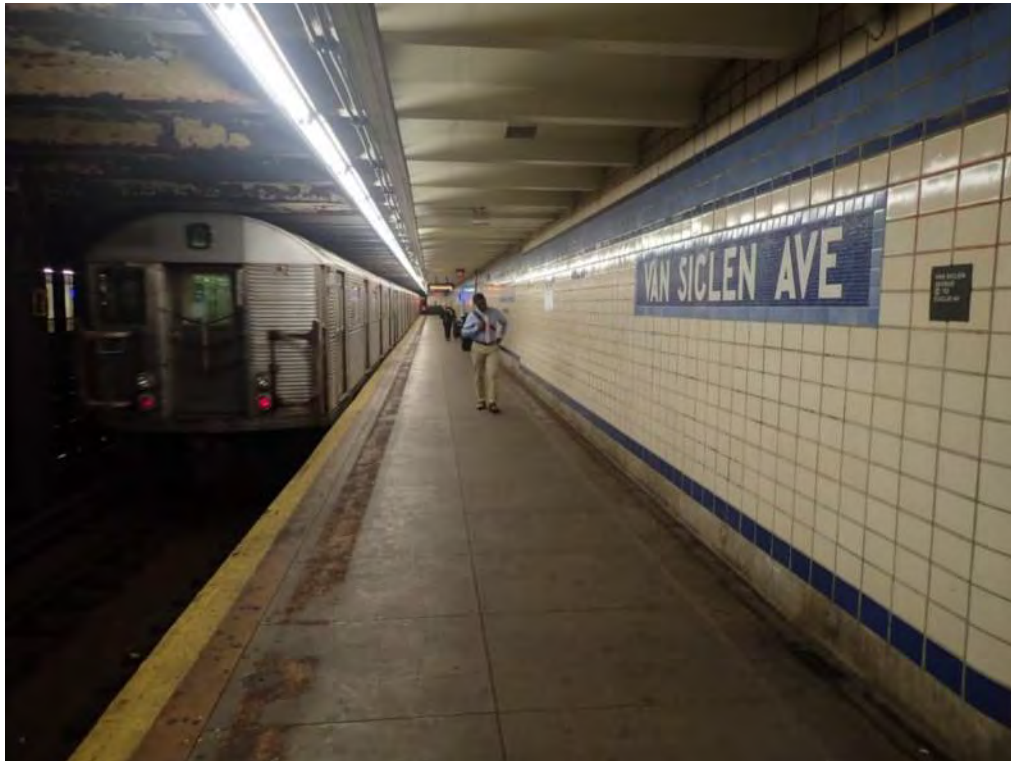
Figure 3 – General platform view Van Siclen Avenue Station
