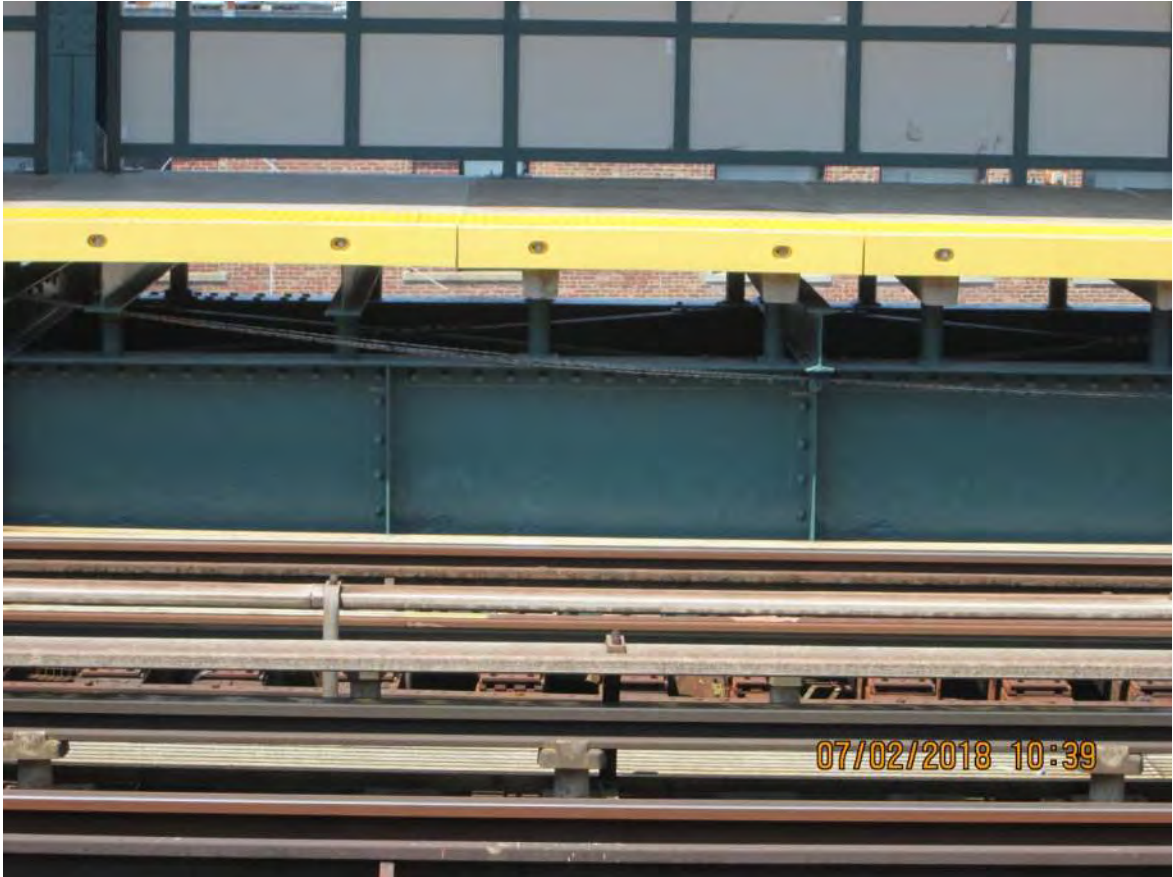
Figure 2– Precast T-Beam platform – Avenue X Station
