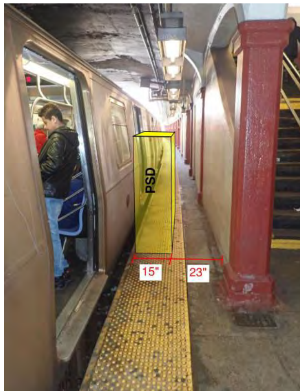
Figure 1 – Area of ADA non-compliance Parkside Avenue Station
