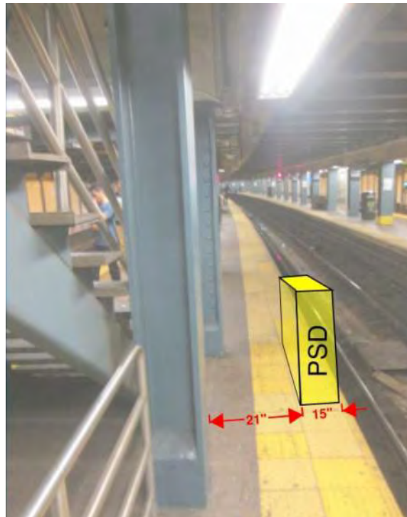
Figure 1 – Non-Compliant ADA condition Whitehall Street Station
