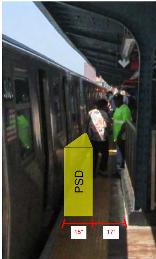
Figure 1 – Non-Compliant ADA condition Knickerbocker Avenue Station
