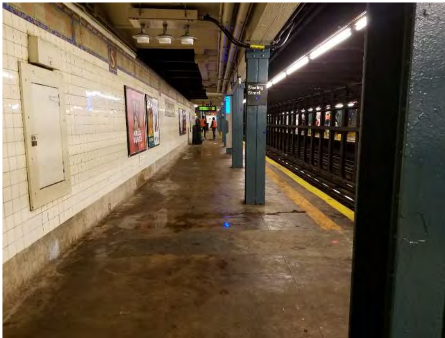
Figure 3 – Typical platform view Sterling Street Station
