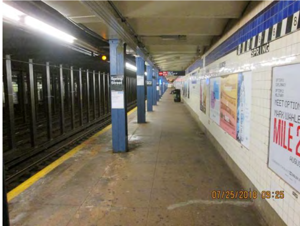
Figure 3 – Typical platform view with signal light Spring Street Station
