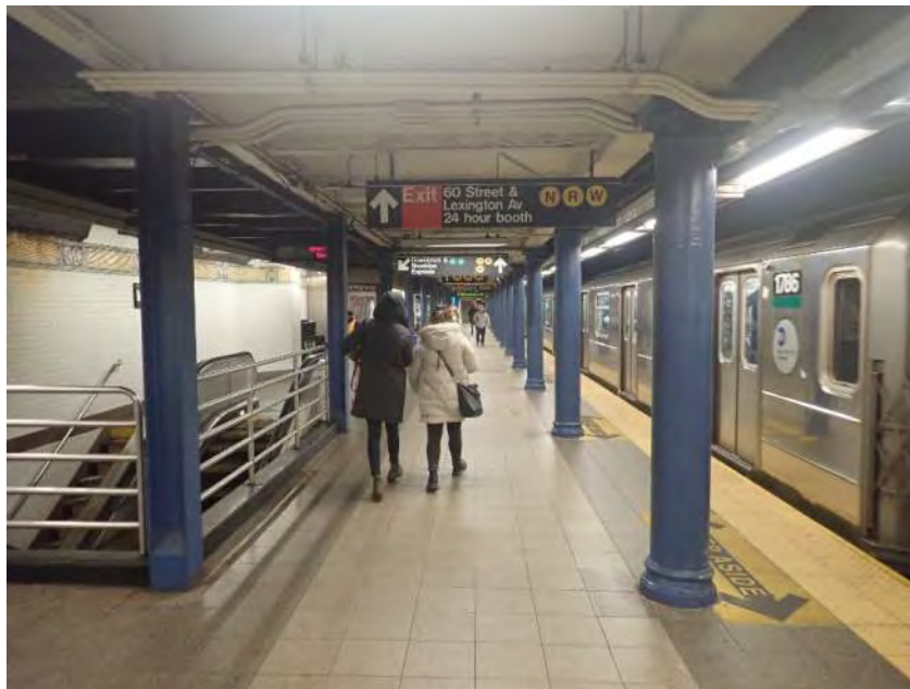
Figure 3 – Typical platform view 59th Street Station
