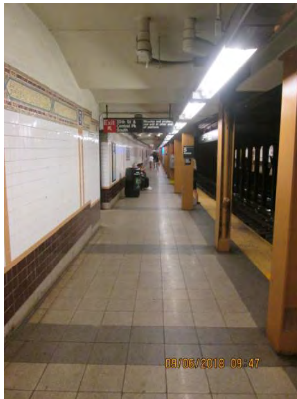
Figure 4 – Typical Platform View Fifth Avenue Station
