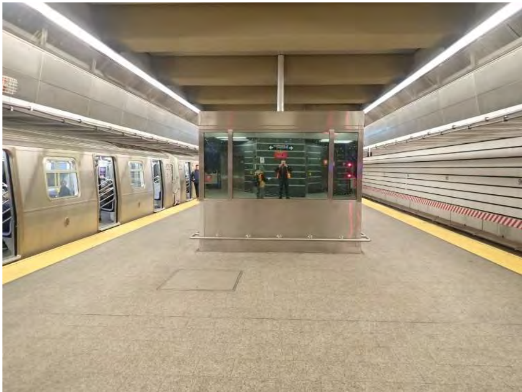
Figure 3 – Typical platform view 96 th Street Station
