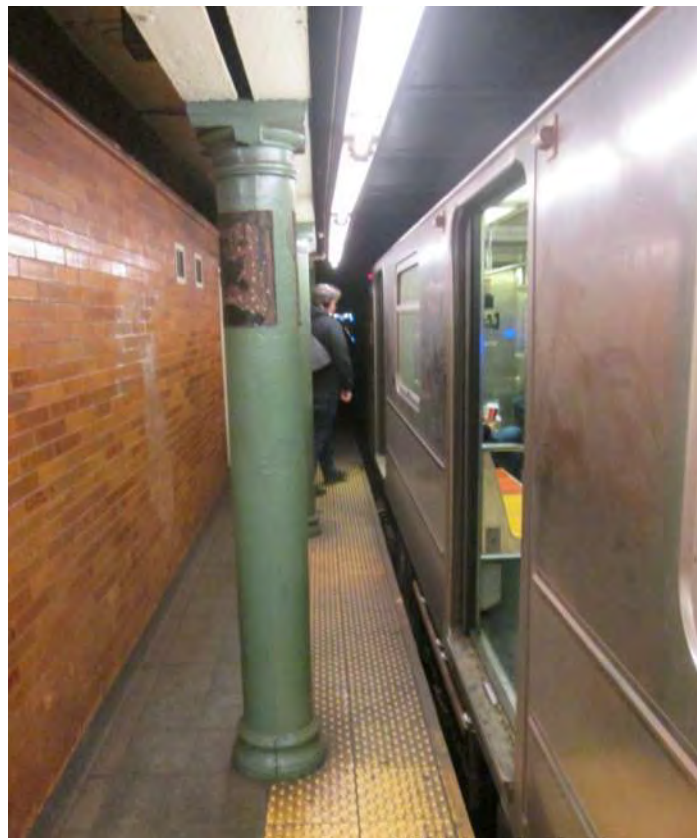
Figure 1 – Column 18” from the edge 66 th Street Station
