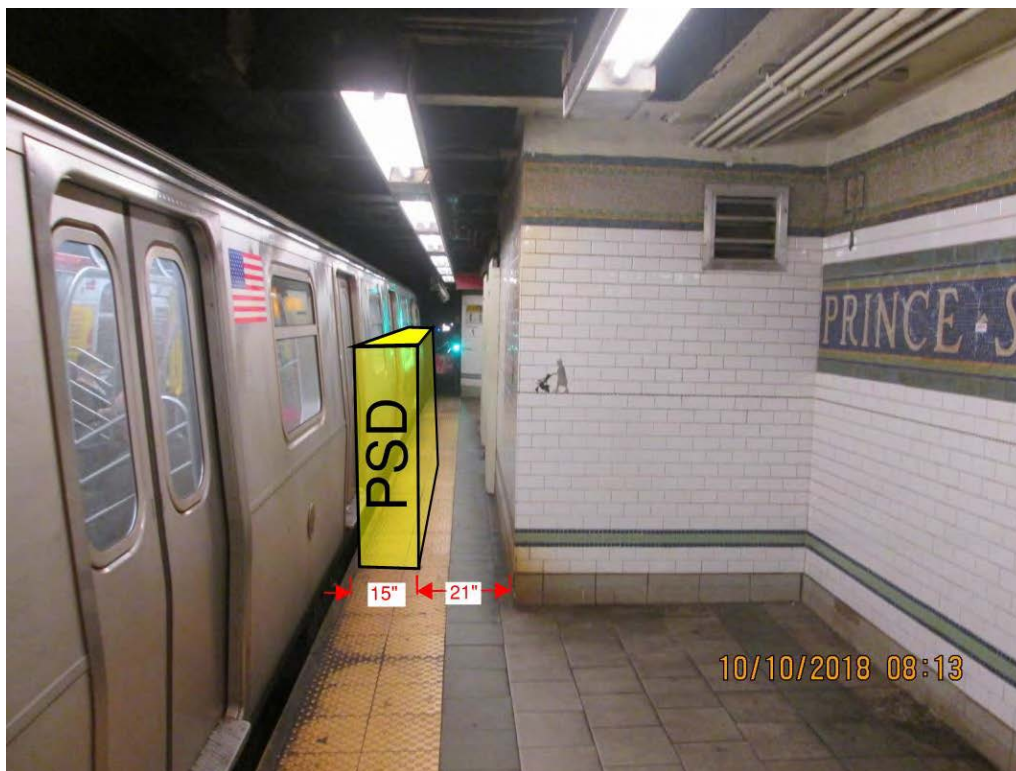
Figure 1 – Non-Compliant ADA condition Prince Street
