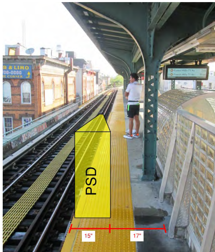
Figure 1 – Non-Compliant ADA condition Seneca Avenue Station
