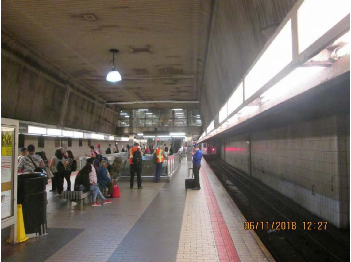
Figure 3 – Typical platform view with back of signal light Sutphin Boulevard Station
