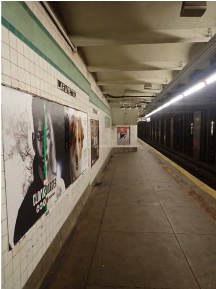
Figure 3 – General platform view Lafayette Avenue Station
