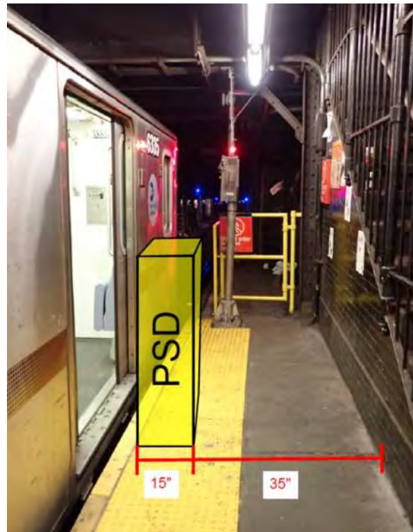
Figure 1 – Non-Compliant ADA condition 149 th Street Station
