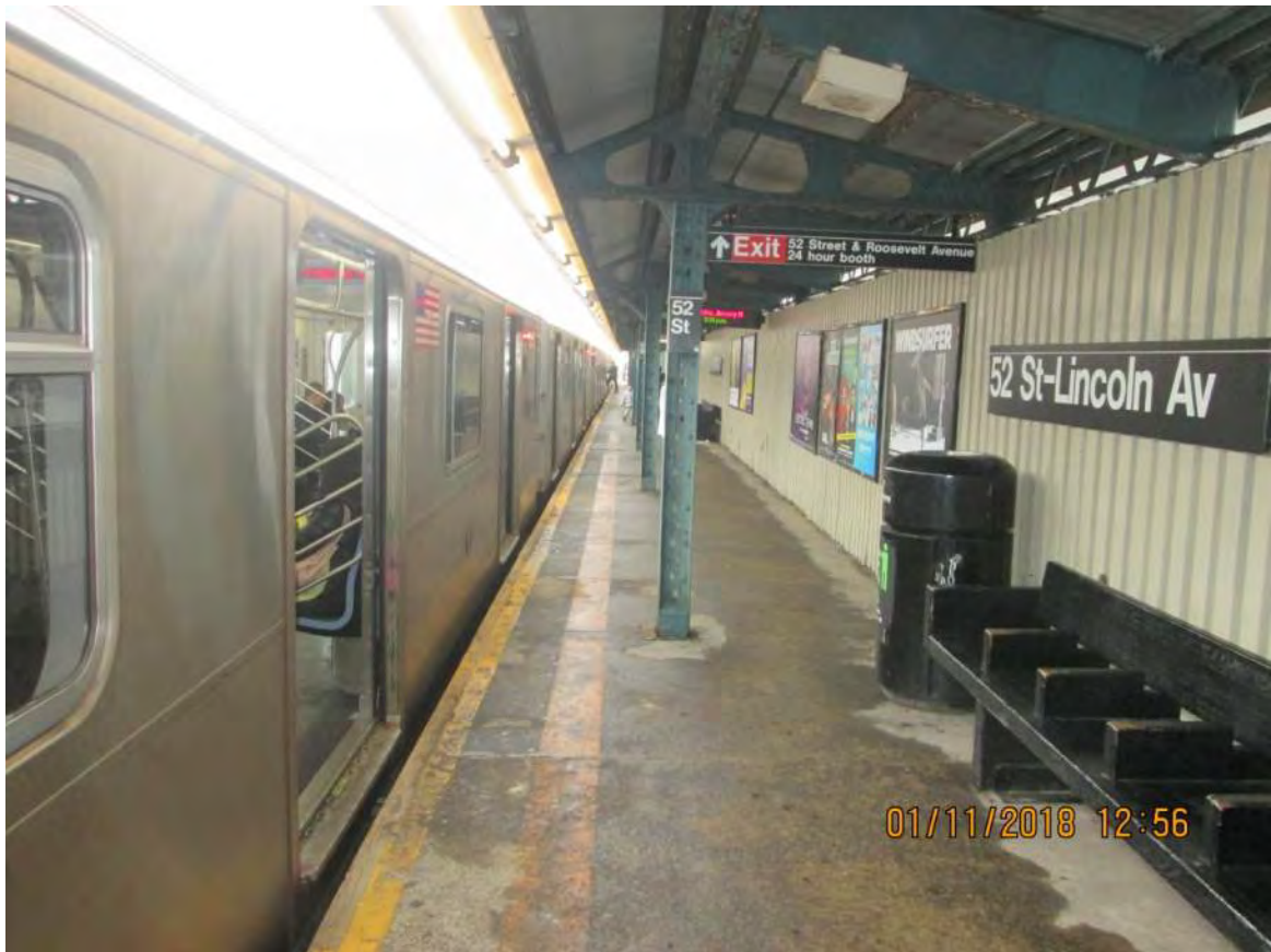
Figure 1 – Typical platform condition – 52 nd Street-Lincoln Avenue Station
