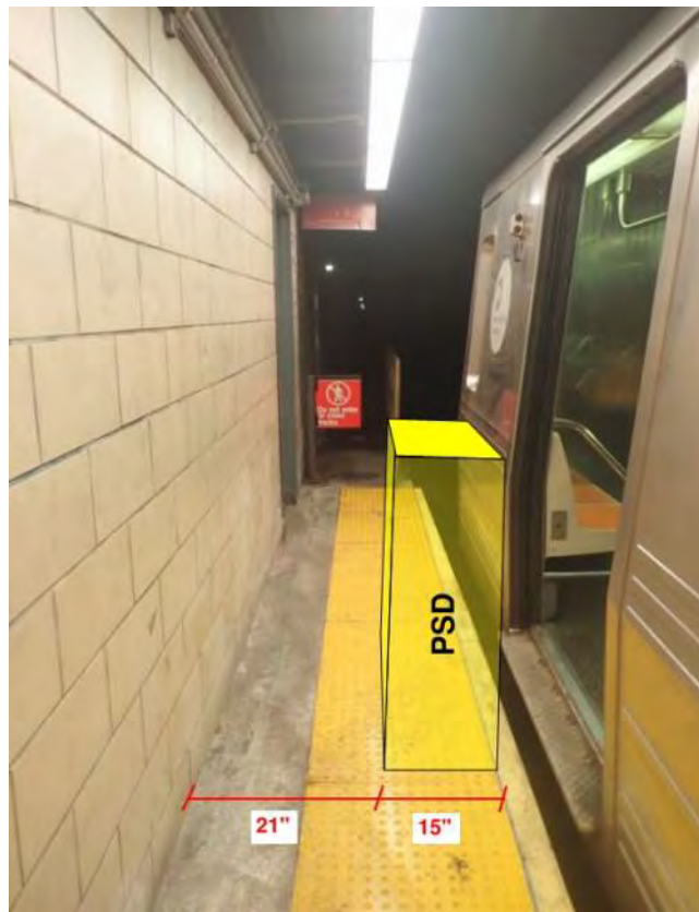
Figure 1 – Non-Compliant ADA condition 86th St Station
