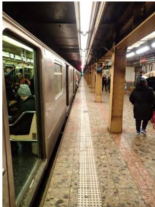
Figure 3 – Typical platform view Franklin Street Station
