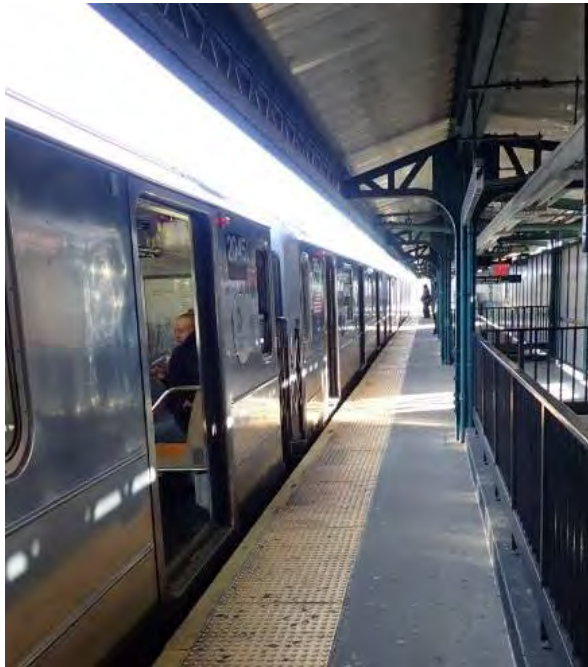
Figure 1 – General Station Condition Elder Avenue Station
