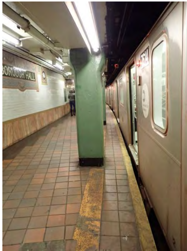
Figure 1 – Column 16” from the edge Borough Hall Station
