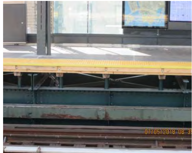
Figure 2 – Precast concrete platforms 30 th Avenue Station
