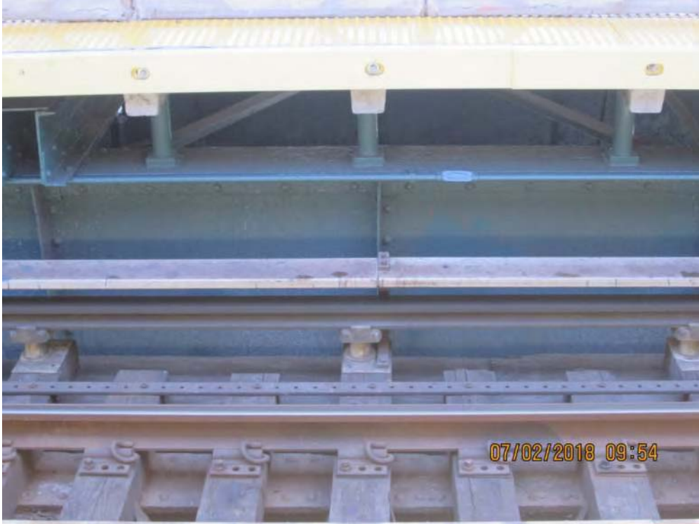
Figure 2– Precast T-Beam platform – Kings Highway Station
