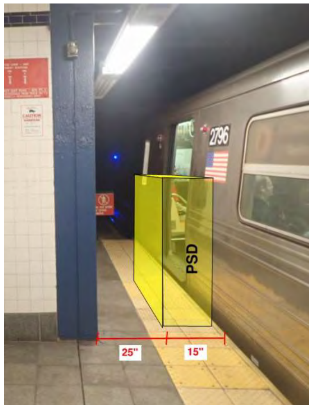
Figure 1 – Non-Compliant ADA condition 81st St. Station
