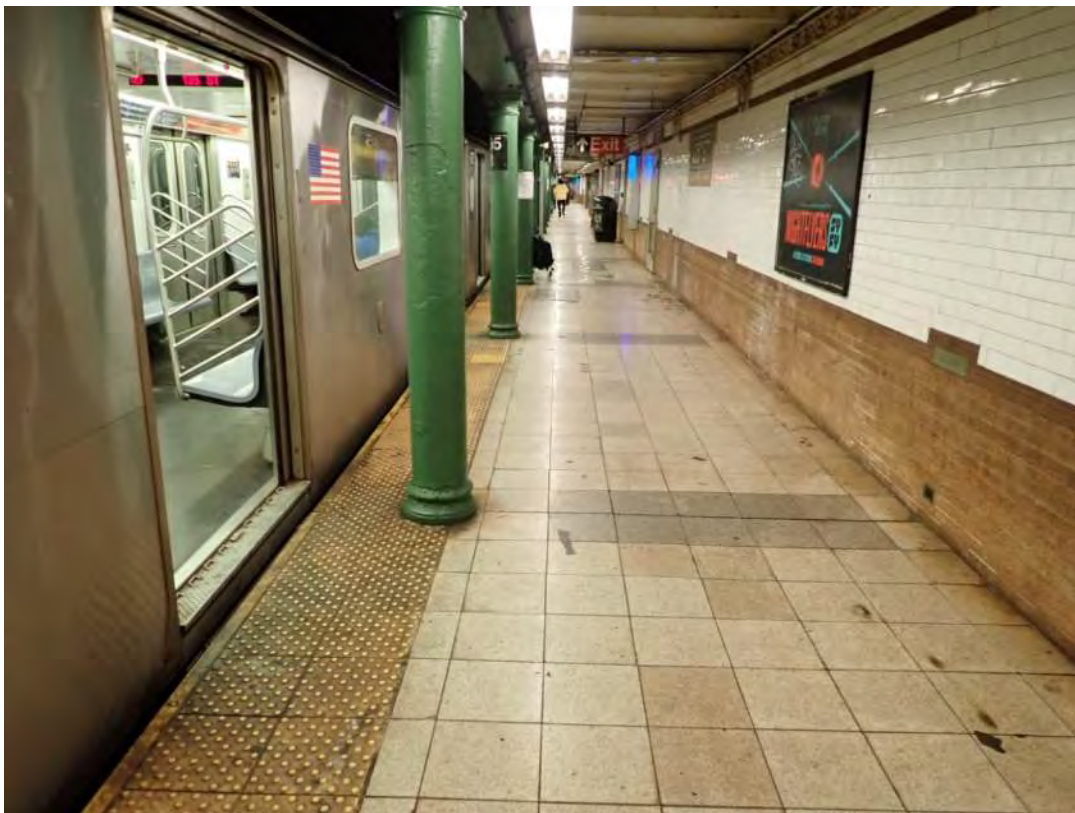
Figure 1 – Column 16” from the edge 135 th Street Station
