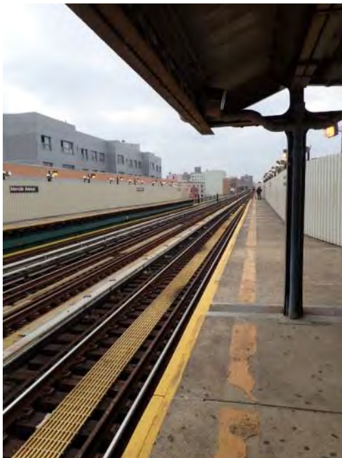
Figure 1 – General Station Condition Intervale Avenue Station
