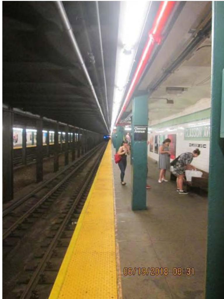
Figure 3 – Typical platform view with standpipe MRN 290 – Classon Avenue Station
