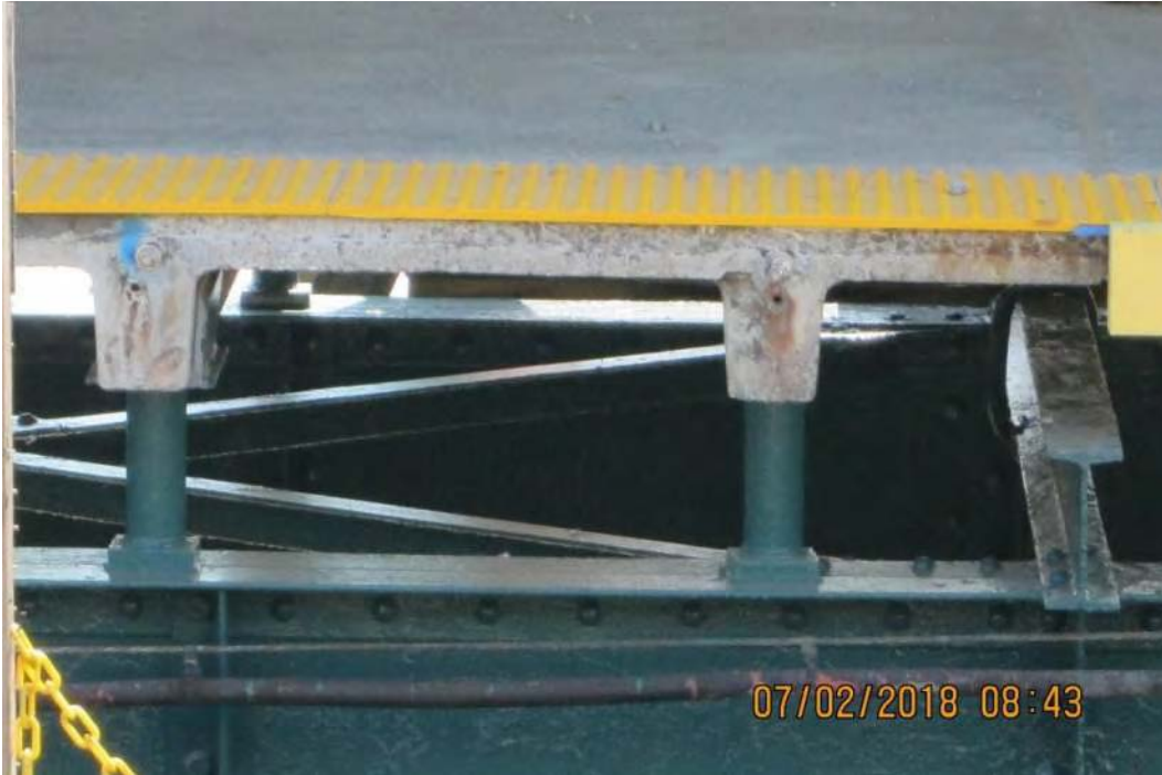
Figure 2– Precast T-Beam platform – Avenue I Station
