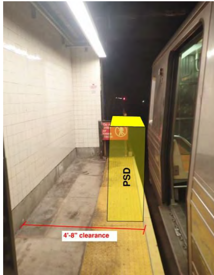
Figure 1 – Non-Compliant ADA condition 72 nd Street Station
