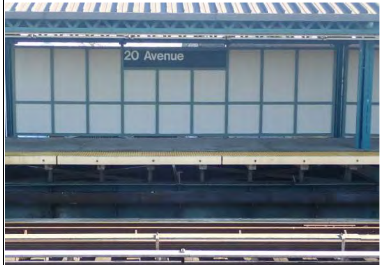
Figure 2 – Precast Slab 20 th Avenue Station
