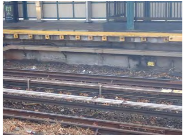
Figure 2 – Precast Slab Bedford Park Boulevard Station
