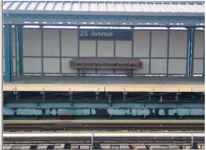
Figure 2 – Precast Slab 25 th Avenue Station
