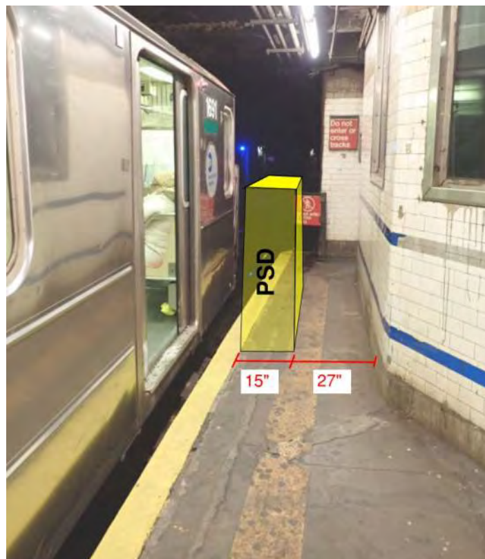
Figure 1 – Non-compliant ADA condition 3rd Avenue -138th Street Station
