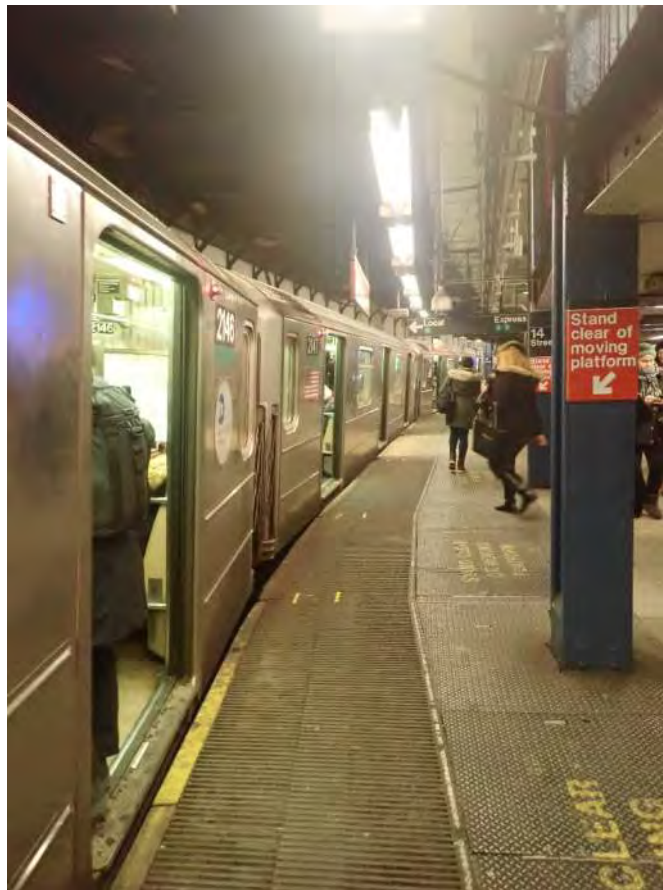
Figure 1 –Platform Edge Gap Fillers 14 th Street Union Square Station
