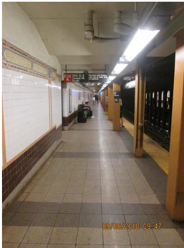
Figure 4 – Typical Platform View Fifth Avenue Station
