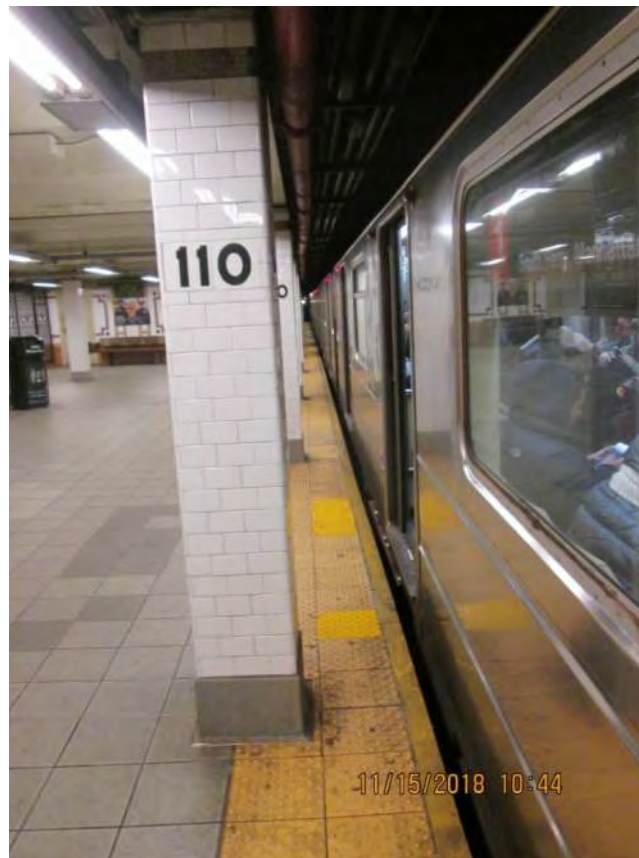
Figure 1 – Column 16” from the edge 110 th Street Station
