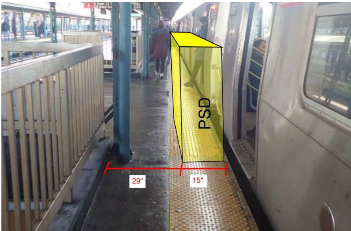
Figure 1 – Area of ADA non-compliance Sheepshead Bay Station
