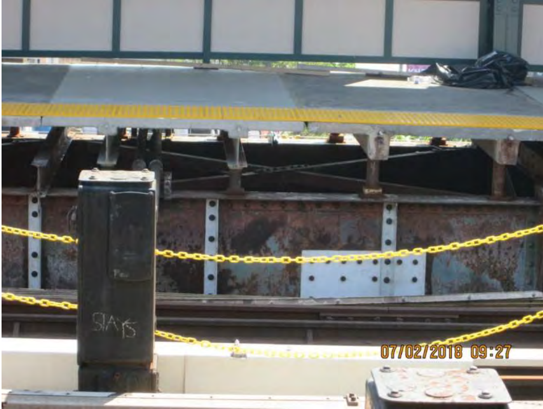
Figure 2– Precast T-Beam platform – Avenue P Station
