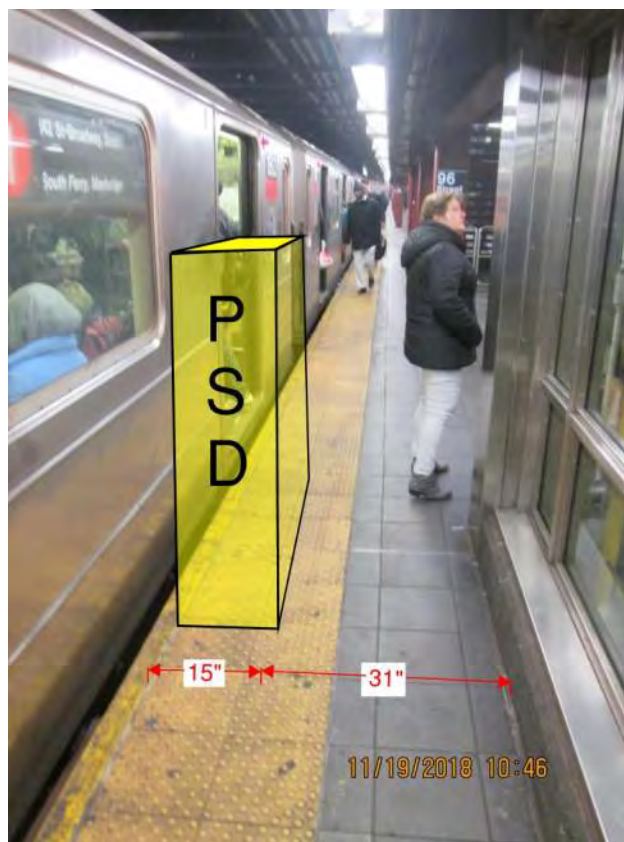
Figure 1 – Non-compliant ADA condition 96 th Street Station
