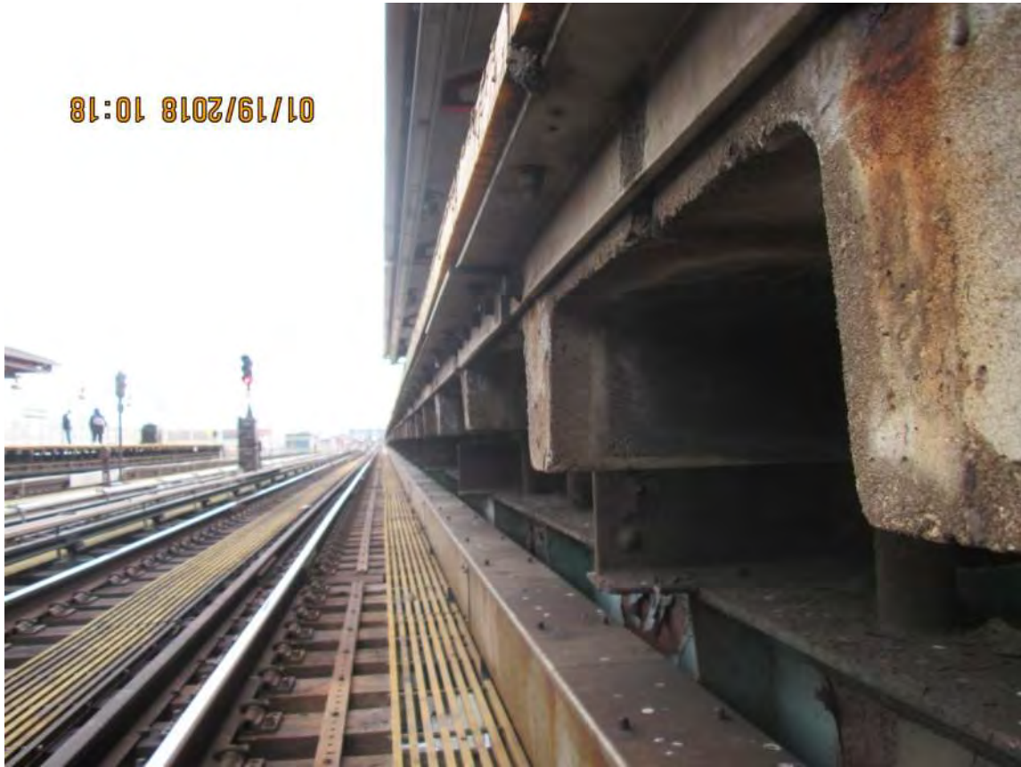
Figure 2 – Precast T-Beam platform – 90th Street-Elmhurst Street Station
