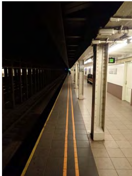
Figure 3 – Typical platform view Canal Street Station
