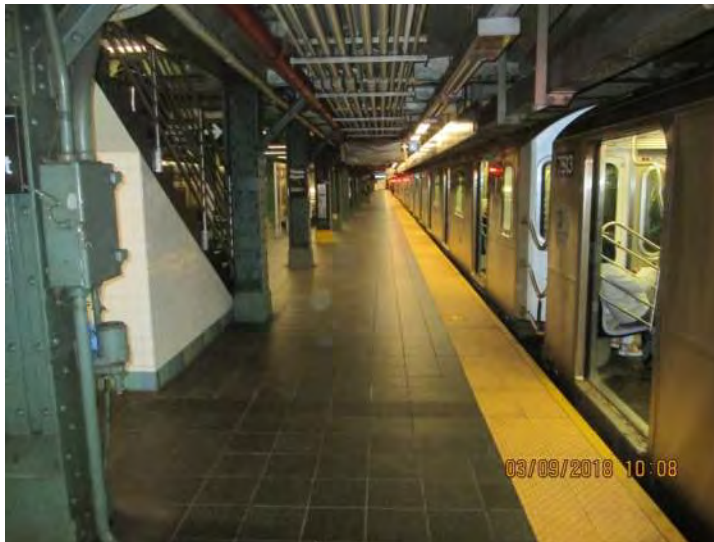
Figure 3 – Typical platform edge condition- 42nd Street-Times Square Station
