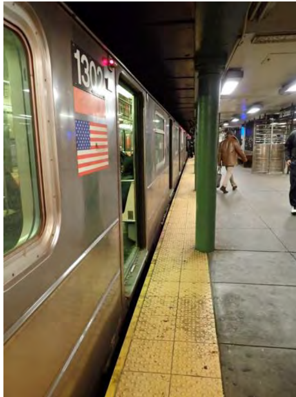
Figure 1 – Column 16” from the edge 116 th Street Station
