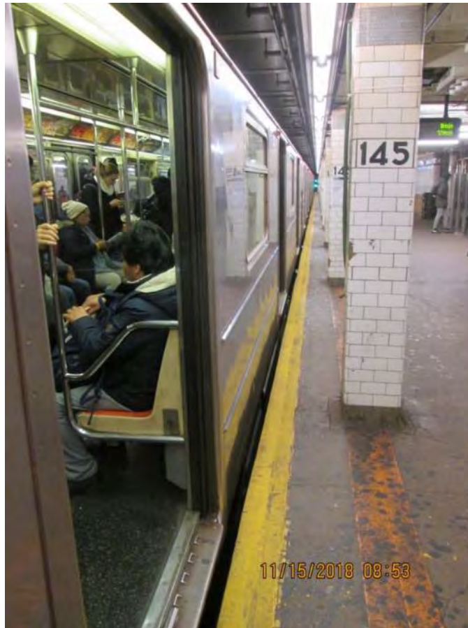
Figure 1 – Column 1'-2" from the edge 145 th Street Station
