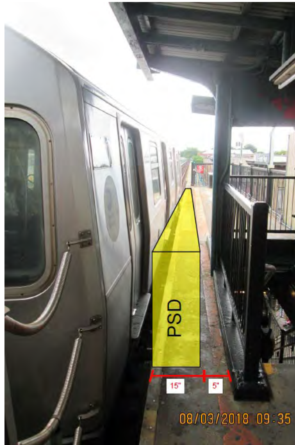
Figure 1 – Non-Compliant ADA condition 85th Street-Forest Parkway Station
