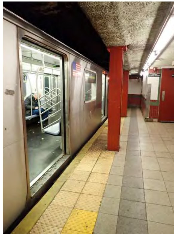
Figure 1 – Column 18” from the edge 3 rd Avenue 149 th Street Station
