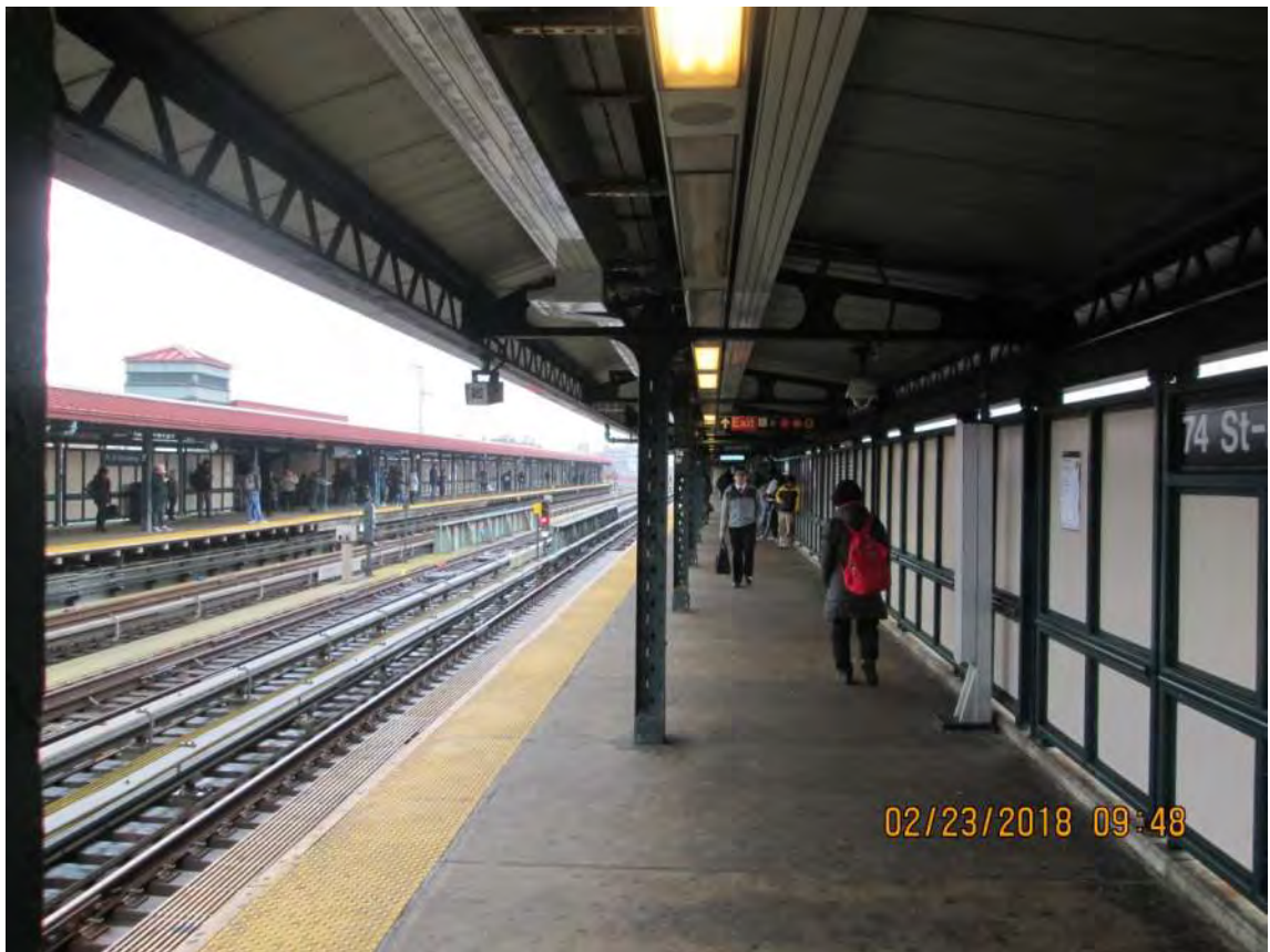
Figure 1–Typical Platform Condition – 74 th Street- Broadway Station
