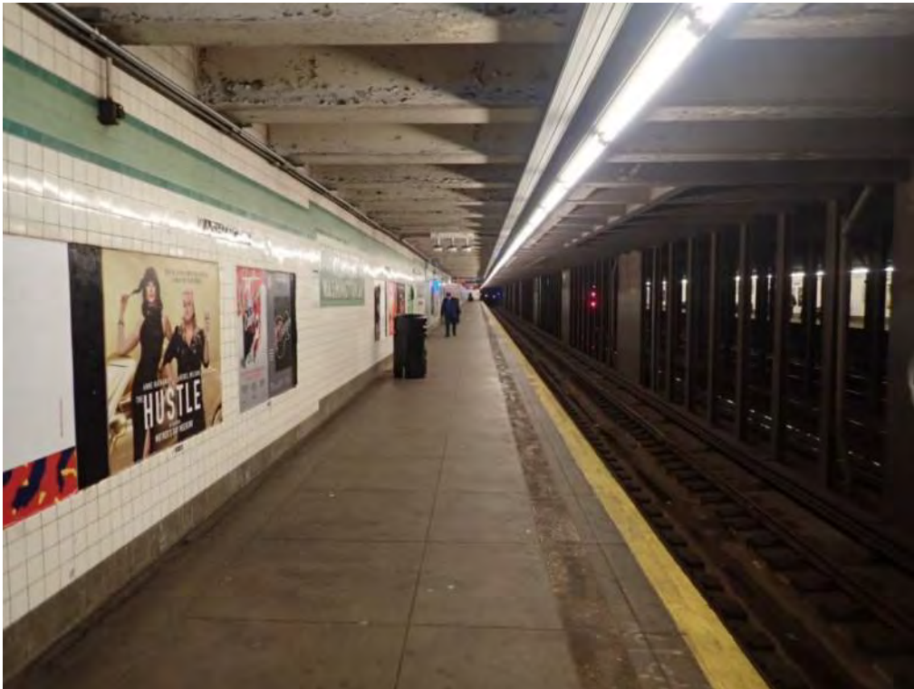
Figure 3 – General platform view Clinton Washington Avenue Station
