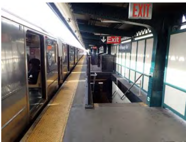
Figure 1 – General Station Condition Rockaway Avenue Station
