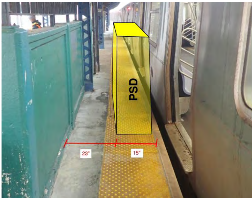
Figure 1 – Area of ADA non-compliance Ocean Parkway Station
