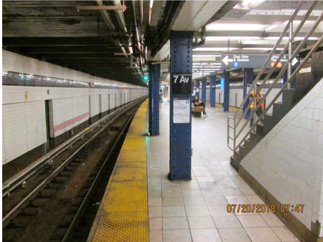
Figure 4 – Typical platform view with back of signal light 7 th Avenue Station
