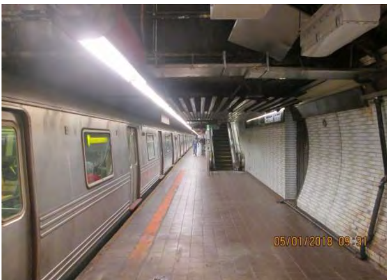
Figure 4 – Platform view featuring low planar ceiling with curved and straight walls- Roosevelt Island Station
