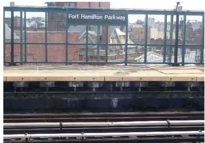
Figure 2 – Precast Slab Fort Hamilton Station
