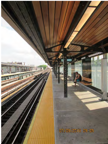
Figure 1 – Overall view 36 th Avenue Station
