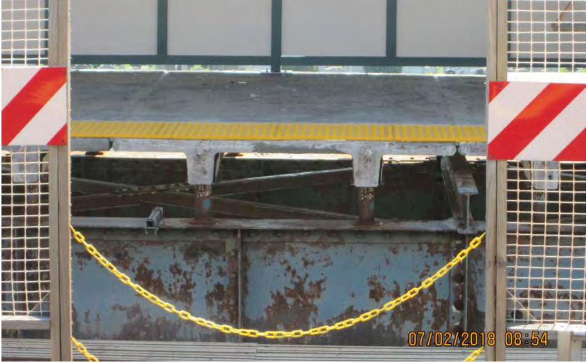
Figure 2– Precast T-Beam platform – Bay Parkway Station
