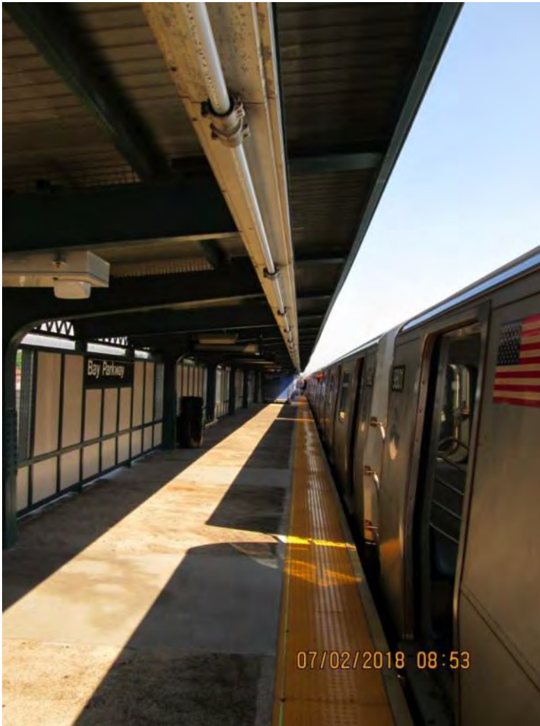
Figure 1– General Platform Condition – Bay Parkway Station
