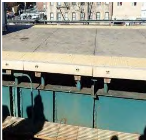
Figure 2 – Precast Slab Parkchester Station
