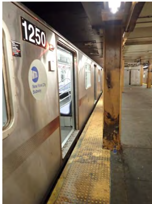
Figure 1 – Column 16” from the edge Franklin Avenue Station
