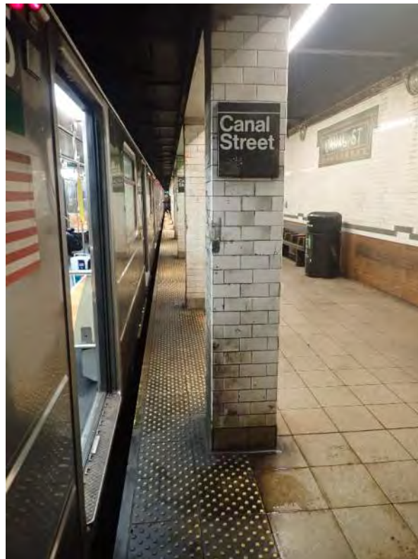
Figure 1 – Column 16” from the edge Canal Street Station
