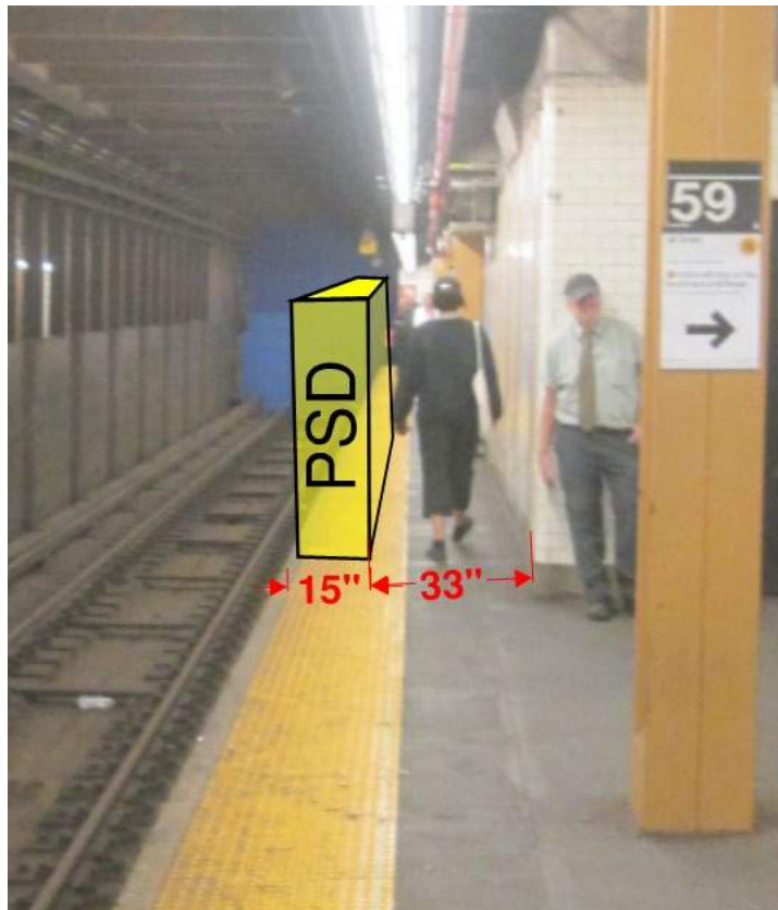
Figure 1 – Non-Compliant ADA condition 59 th Street Station
