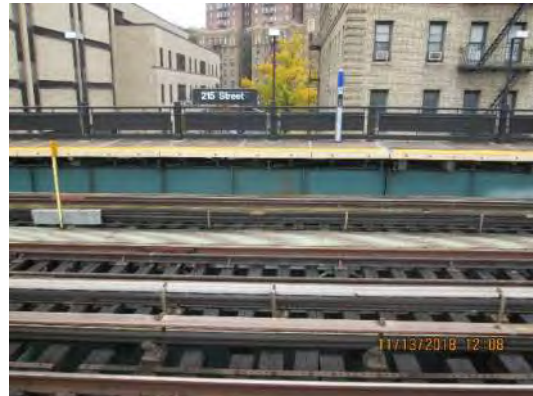
Figure 2 – Precast concrete platforms 215 th Street Station
