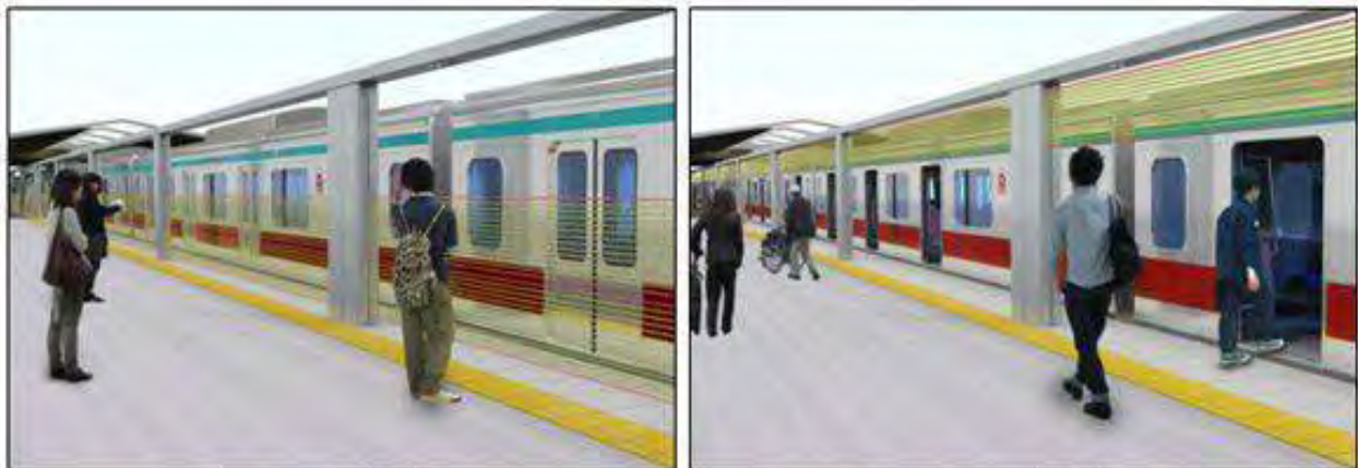
Photo 3 – Roped Platform Screen Doors, (closed in left image, open in right image)
