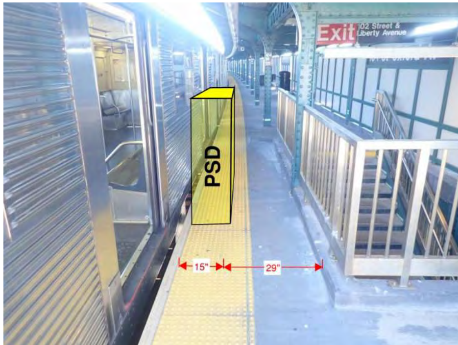
Figure 1 – Non-Compliant ADA condition 104 th Street
