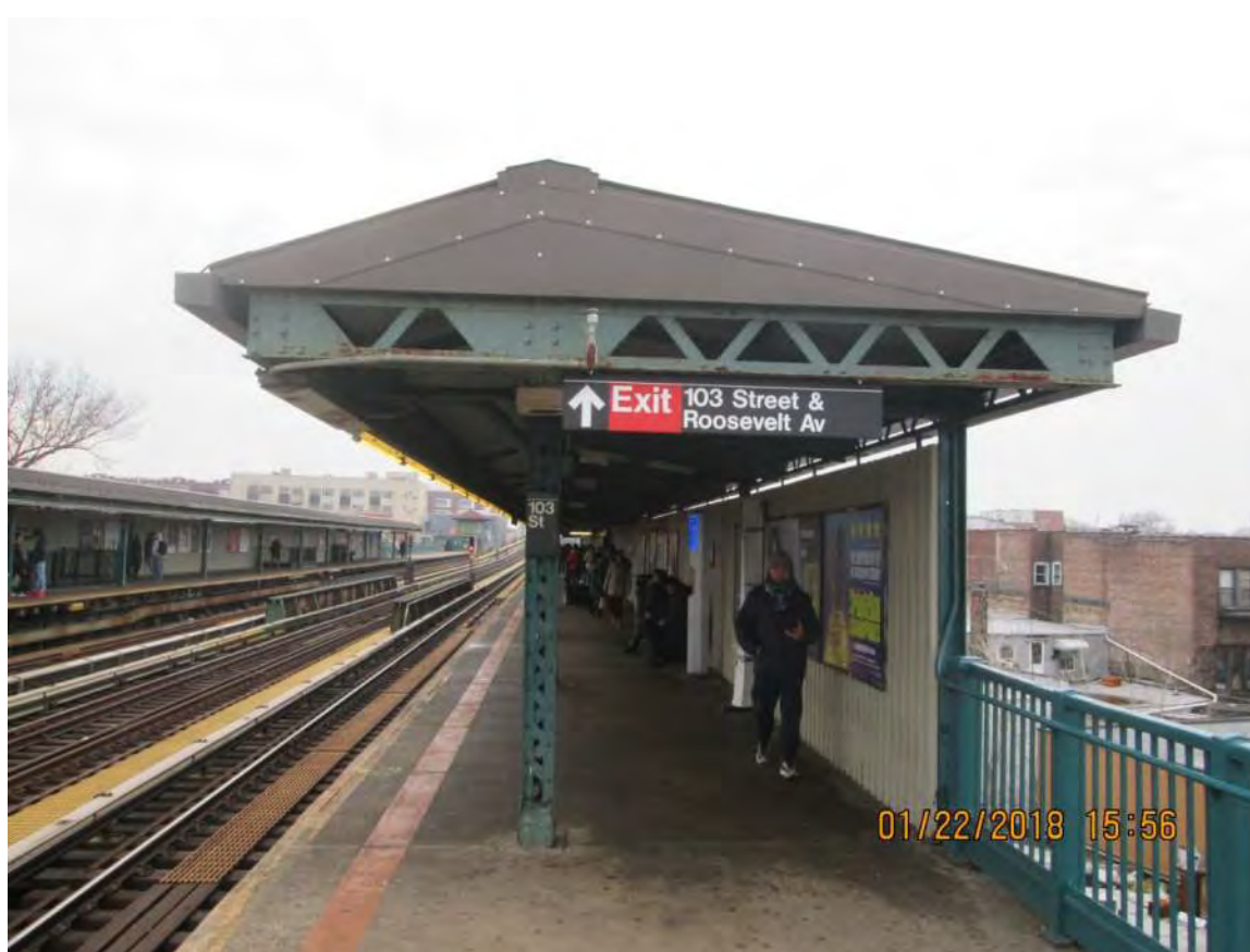
Figure 1 – Typical platform condition – 103rd Street-Corona Plaza Station
