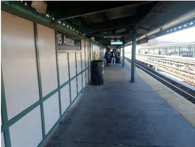
Figure 1 – General Station Condition 18 th Avenue Station
