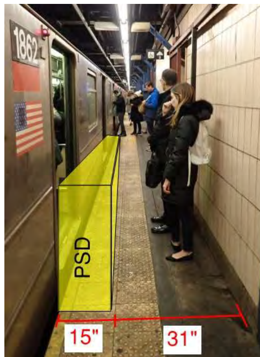
Figure 1 – Non-compliant ADA condition Chambers Street Station
