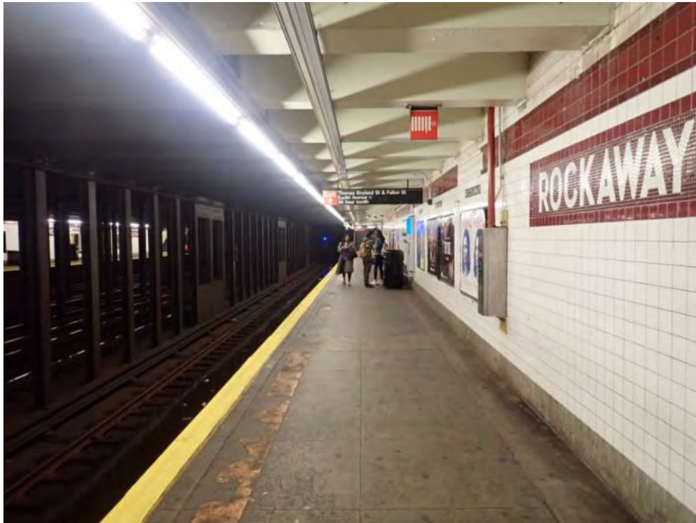
Figure 3 – General platform view Rockaway Avenue Station
