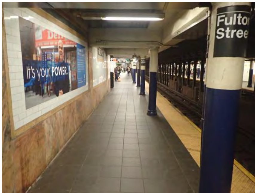
Figure 3 – Typical platform view Fulton Street Station
