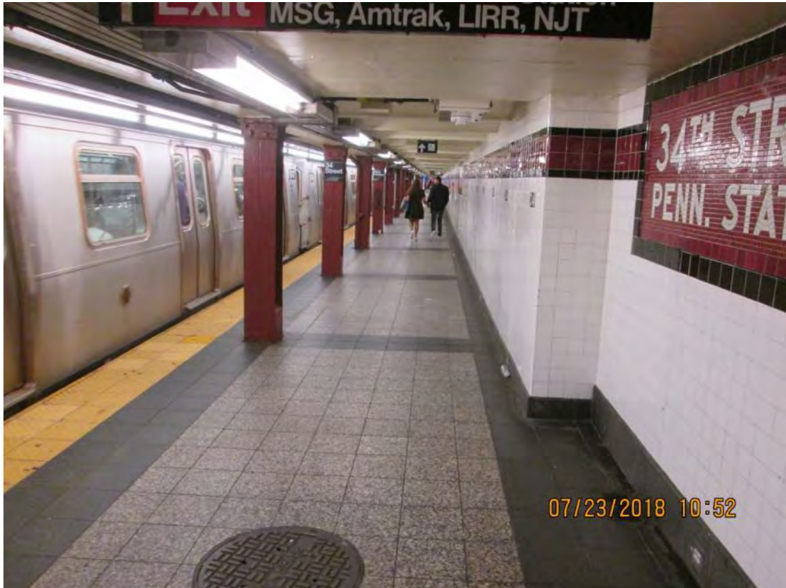
Figure 3 – Typical platform view (C-train platform) 34 th Street Station
