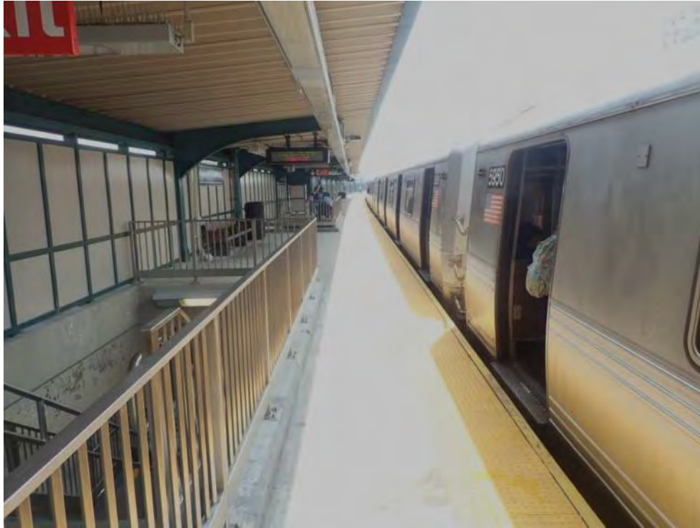
Figure 3 – General platform view Beach 60 th Street Station
