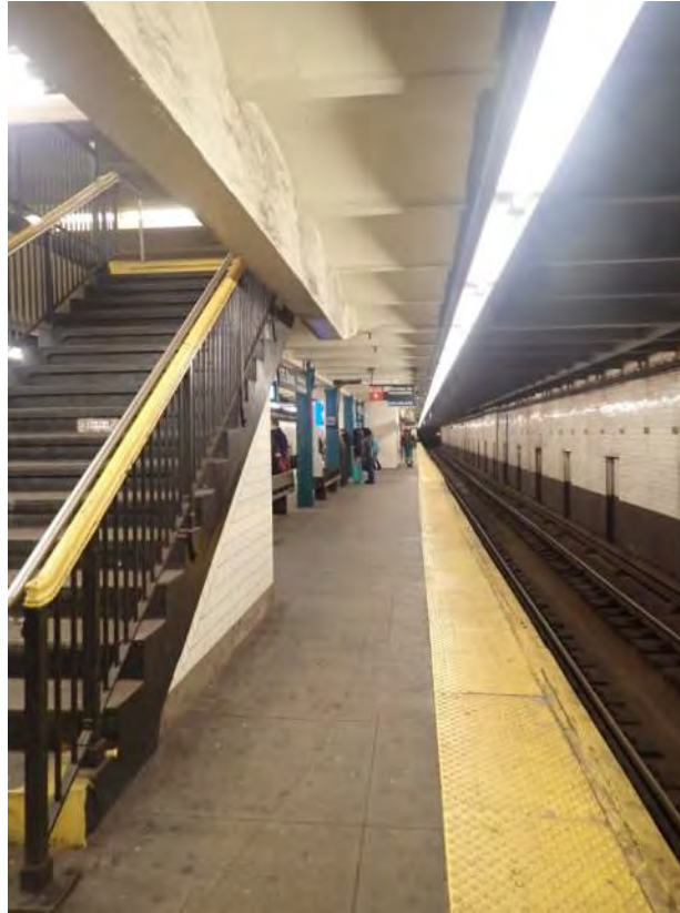
Figure 3 – Typical platform view 175 th Street Station
