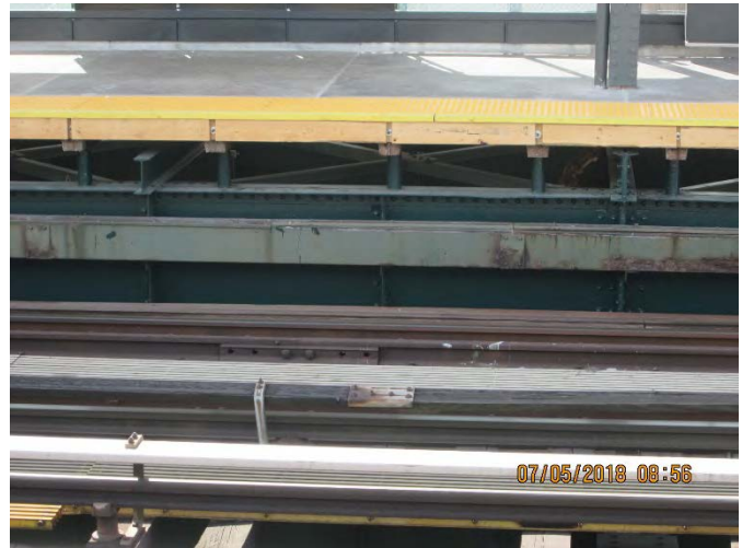
Figure 2 – Precast concrete platforms 36 th Avenue Station
