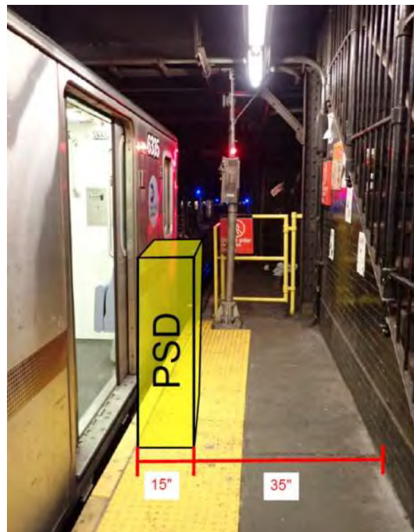
Figure 1 – Non-Compliant ADA condition 149 th Street Station
