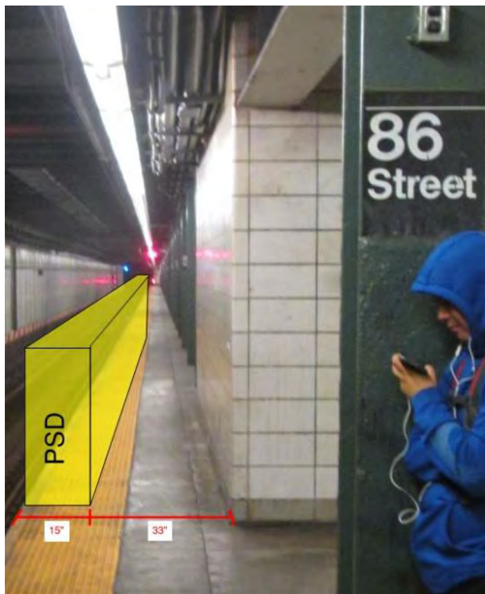
Figure 1 – Non compliant ADA Condition 86 th Street Station
