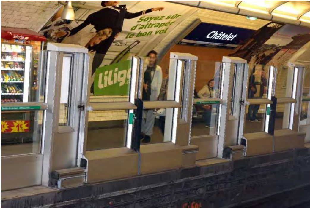
Photo 2 – Automatic Platform Gates at Châtelet Station, Paris, France
