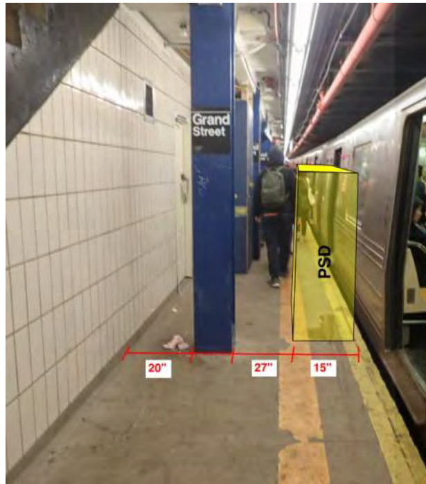
Figure 1 – Area of ADA non-compliance Grand Street Station
