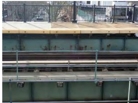
Figure 2 – Precast Slab Van Siclen Avenue Station
