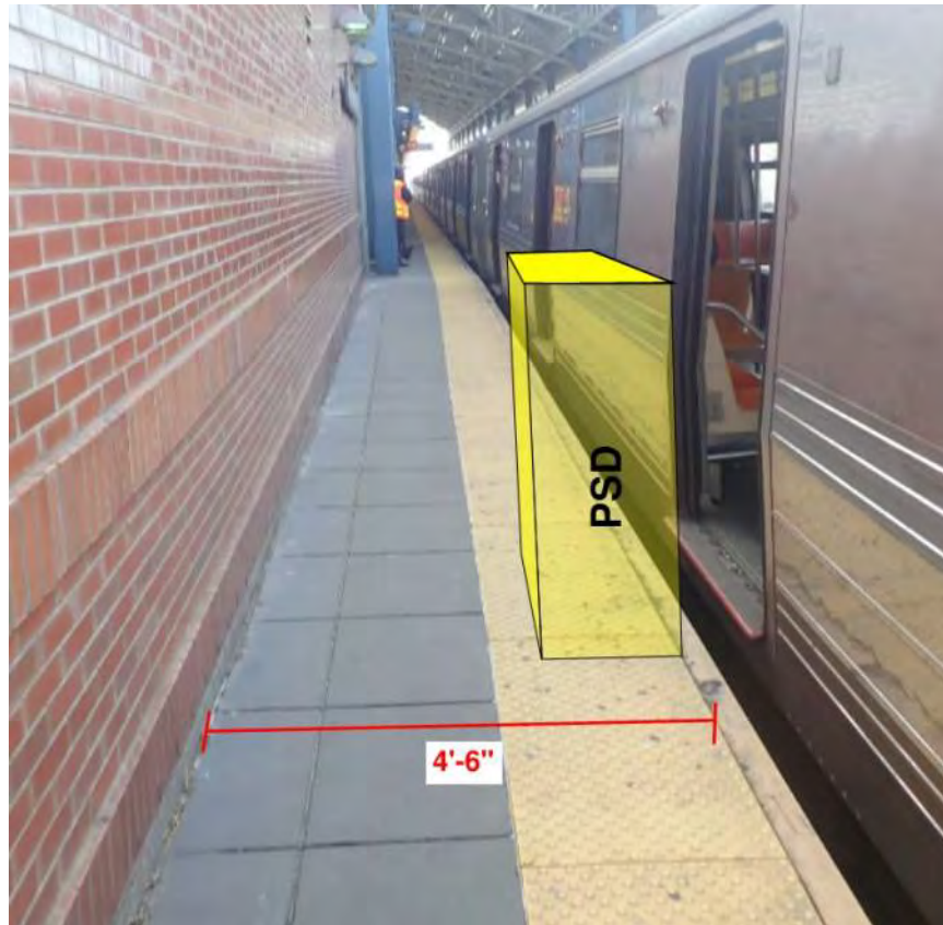
Figure 1 – Non-Compliant egress condition Coney Island Stillwell Avenue Station
