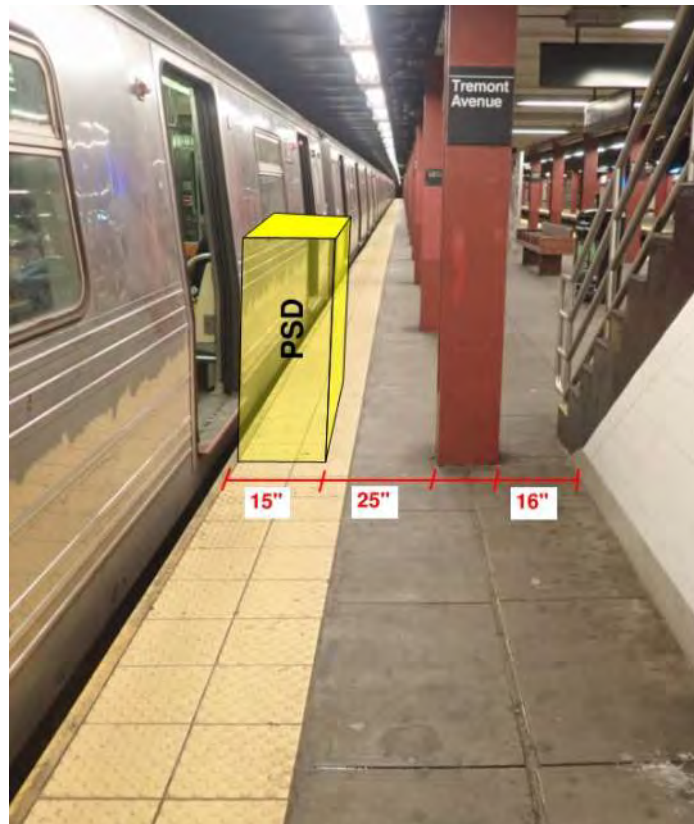
Figure 1 – Non-Compliant ADA condition Tremont Avenue
