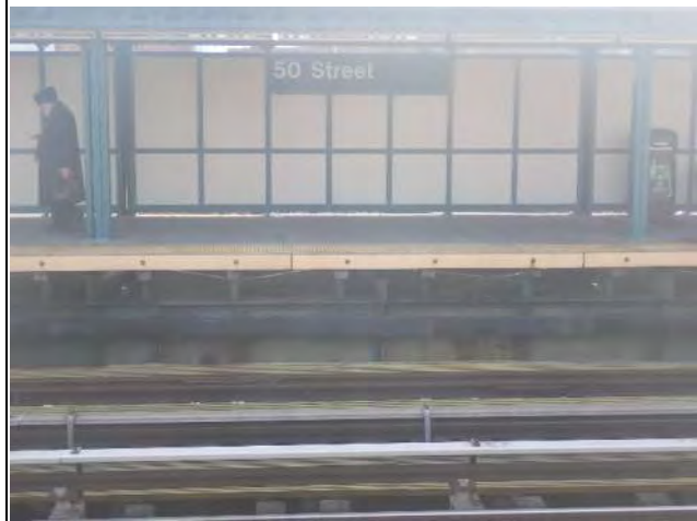
Figure 2 – Precast Slab 50 th Street Station
