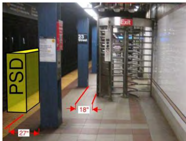
Figure 2 – Non-Compliant ADA condition - 23 rd Street
