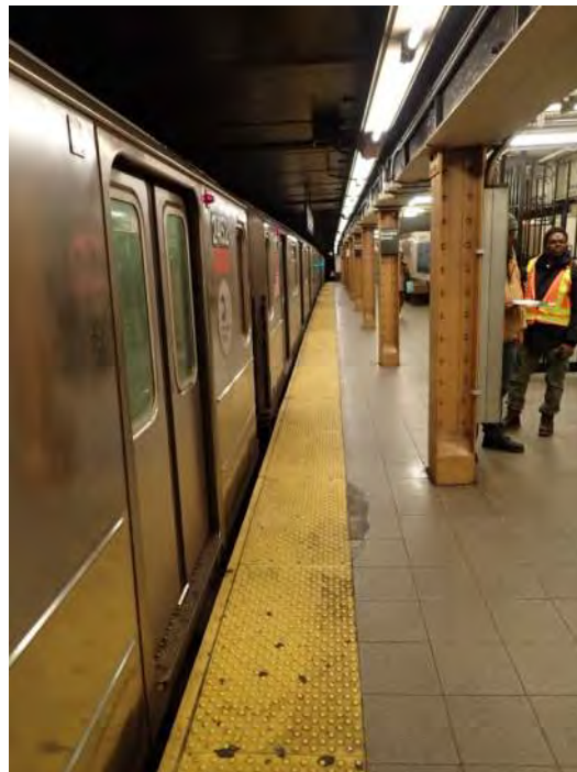
Figure 3 – Typical platform view Houston Street Station
