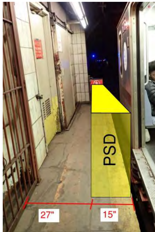
Figure 1 – Non-compliant ADA condition President Street Station
