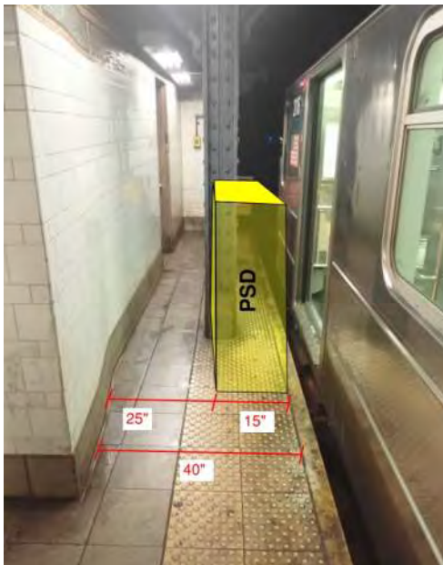
Figure 1 – Non-Compliant ADA clearance North end of lower platform; 125 th Street Station
