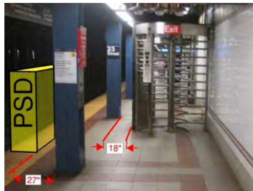
Figure 2 – Non-Compliant ADA condition - 23 rd Street
