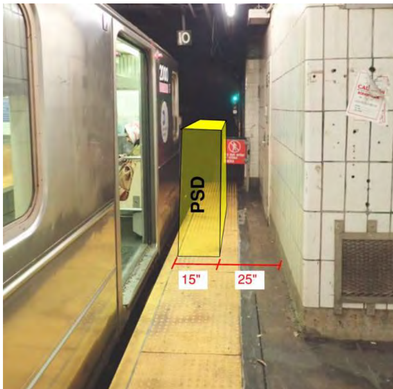
Figure 1 – Area of ADA non-compliance Longwood Avenue Station
