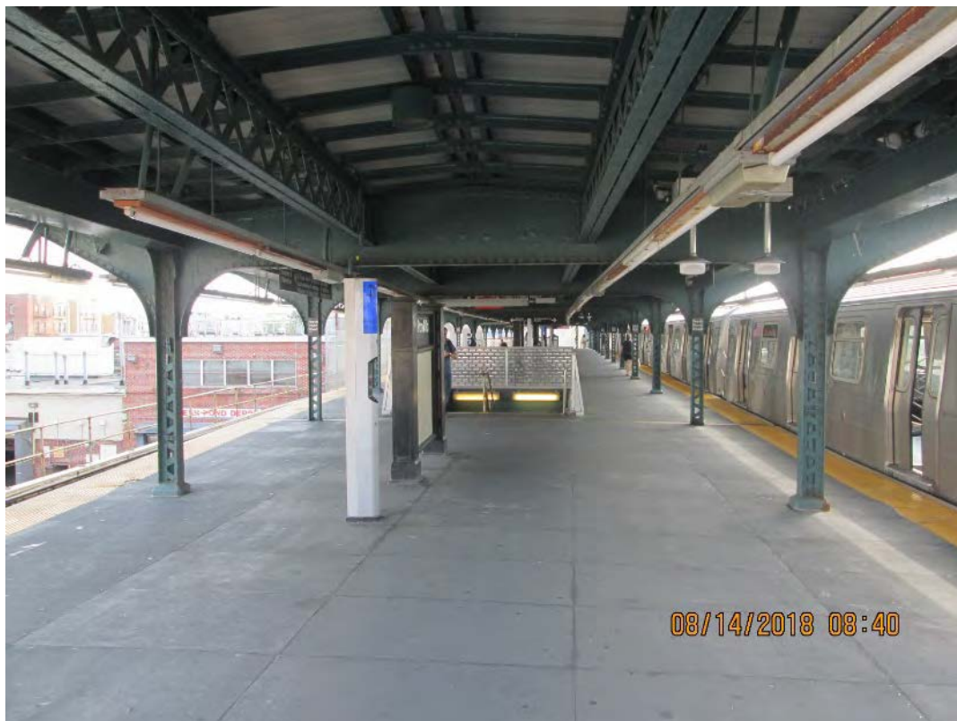
Figure 3 – Typical platform view Fresh Pond Road Station
