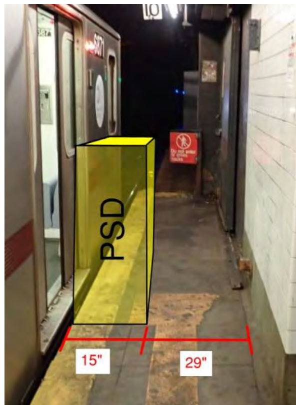
Figure 1 – Non-compliant ADA condition Winthrop Street Station
