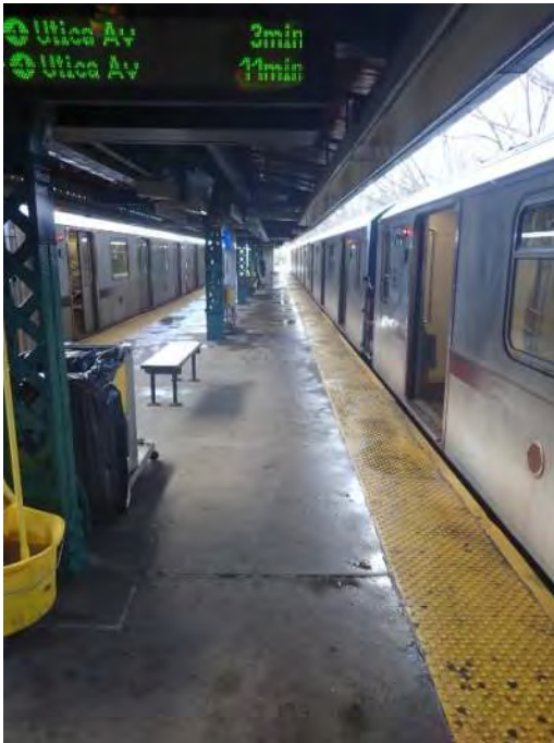
Figure 1 – General Station Condition Woodlawn Station
