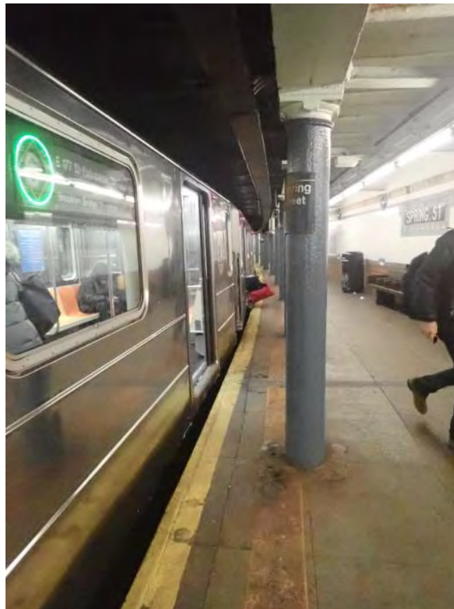
Figure 1 – Column 22” from the edge Spring St. Station
