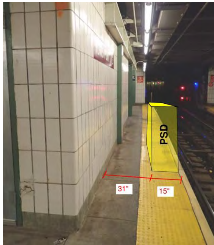
Figure 1 – Area of ADA non-compliance Hunts Point Avenue Station
