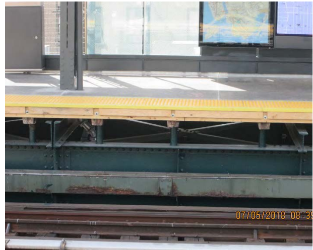
Figure 2 – Precast concrete platforms 30 th Avenue Station
