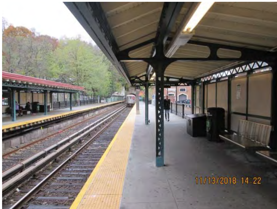
Figure 3 – Typical platform view Dyckman Street Station
