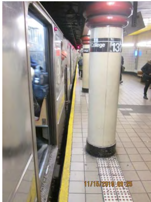
Figure 1 – Column 1'-2" from the edge 137 th Street Station
