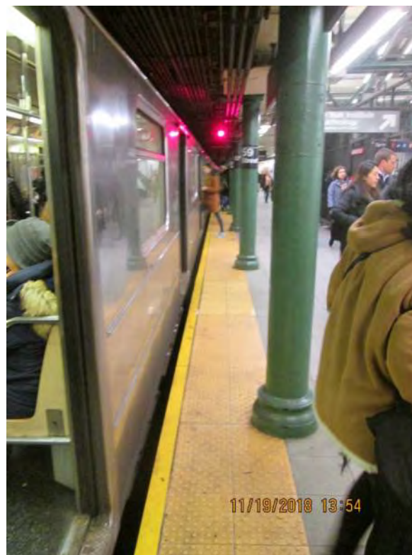
Figure 1 – Column 18” from the edge 59 th Street Station
