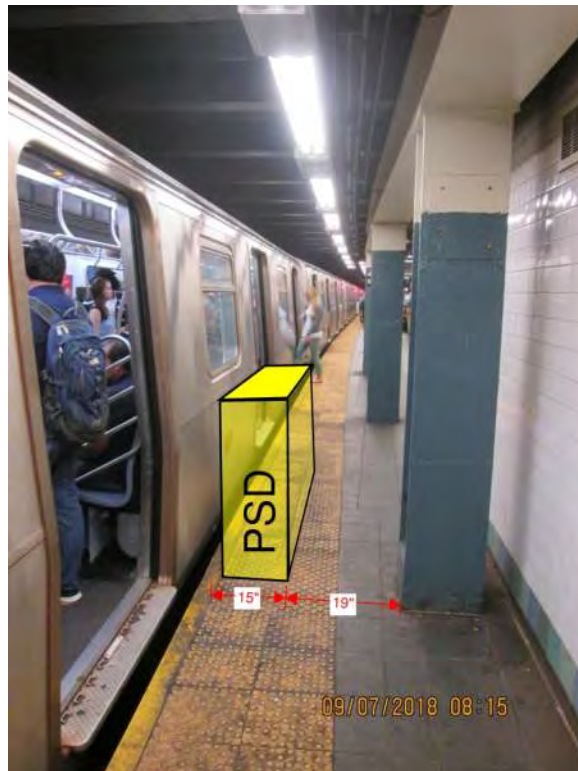
Figure 1 – Non-Compliant ADA condition 42 nd Street / Times Square Station
