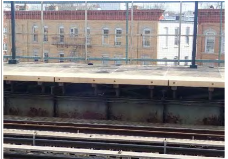
Figure 2 – Precast Slab 79 th Street Station
