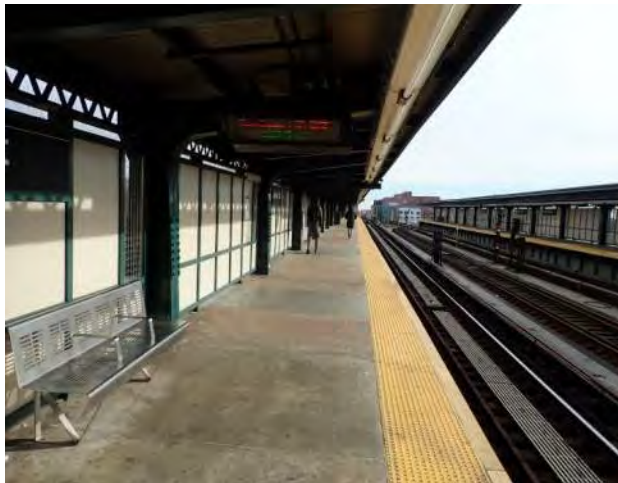
Figure 1 – General Station Condition Junius Street Station
