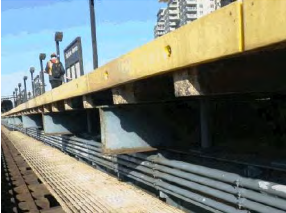
Figure 2– Precast T-beam Platform – Neptune Avenue Station
