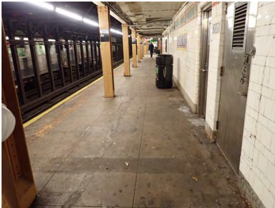
Figure 3 – Typical platform view Brook Avenue Station
