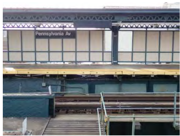
Figure 2 – Precast Slab Pennsylvania Avenue Station
