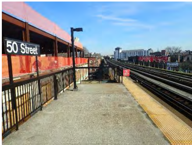
Figure 1 – General Station Condition 50 th Street Station
