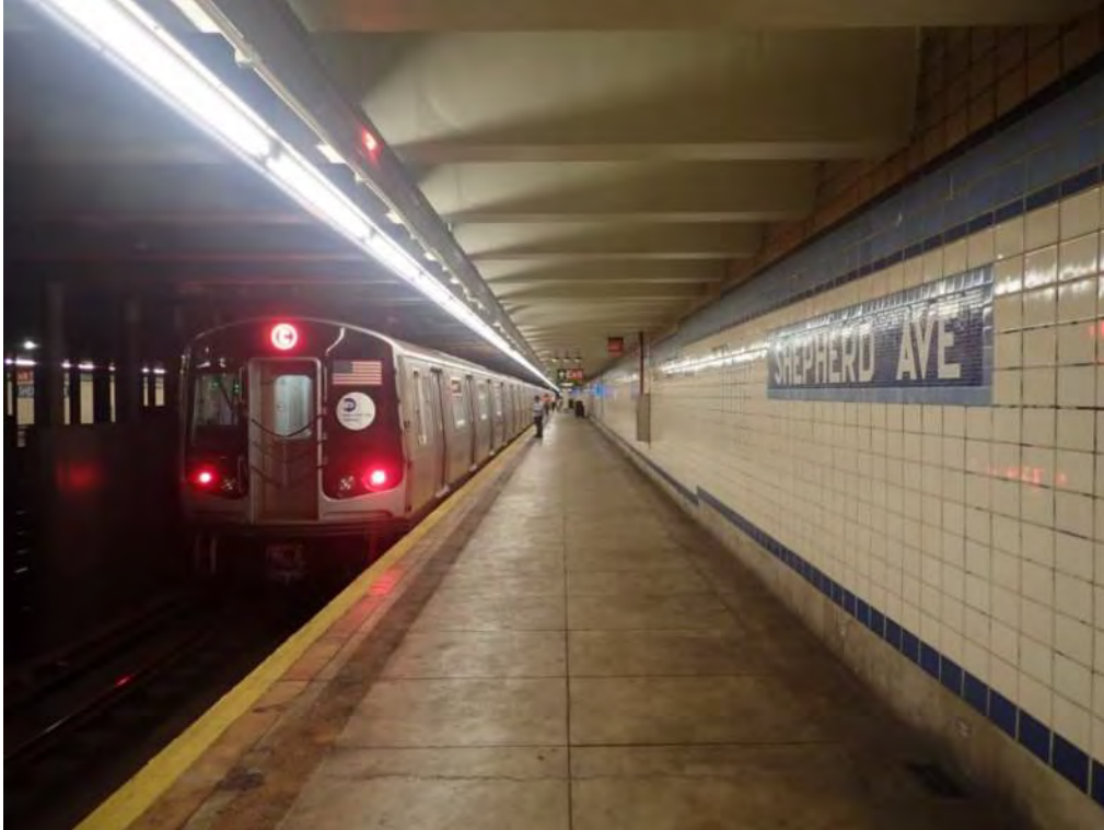
Figure 3 – General platform view Shepherd Avenue Station
