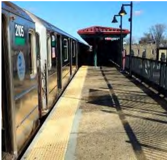
Figure 1 – General Station Condition Saint Lawrence Avenue Station
