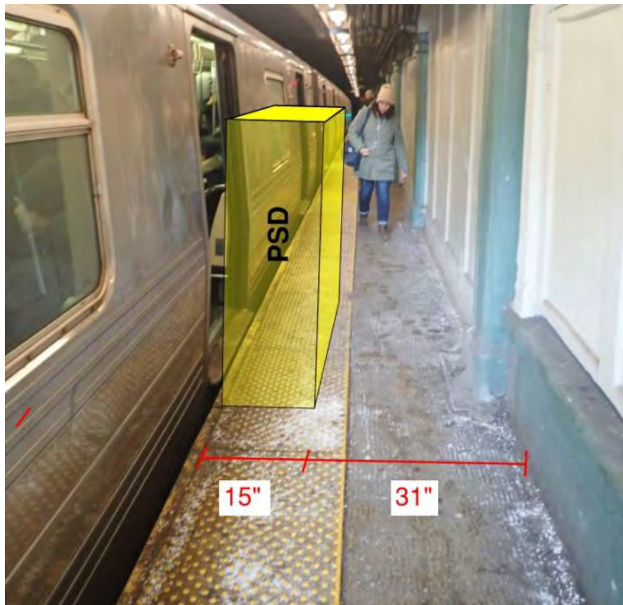
Figure 1 – Non-compliant ADA condition Prospect Park Station
