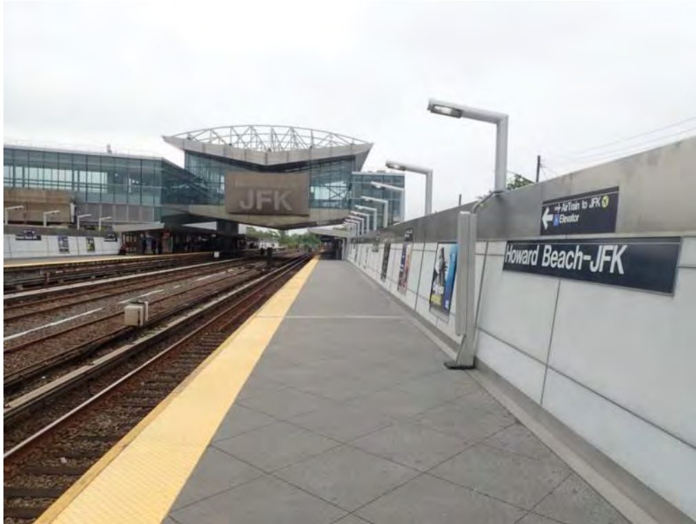
Figure 3 – General platform view Howard Beach - Airtrain Station
