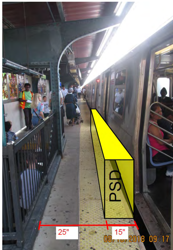
Figure 1 – Non-Compliant ADA condition Lorimer Street Station
