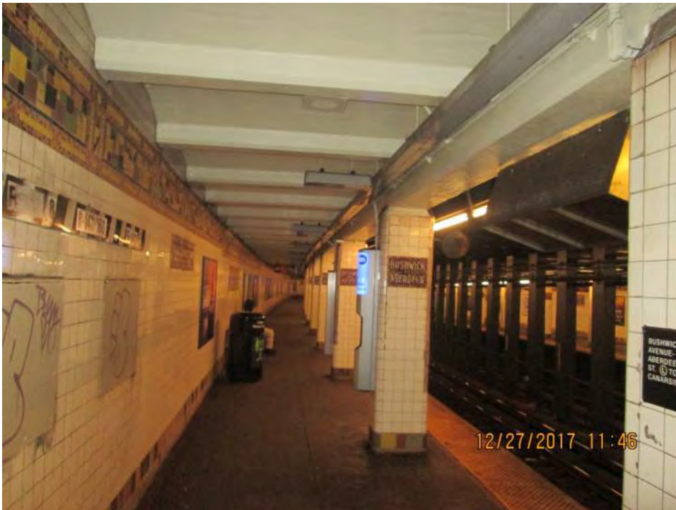
Figure 3 – General view of Canarsie-bound track platform – Bushwick Avenue Station
