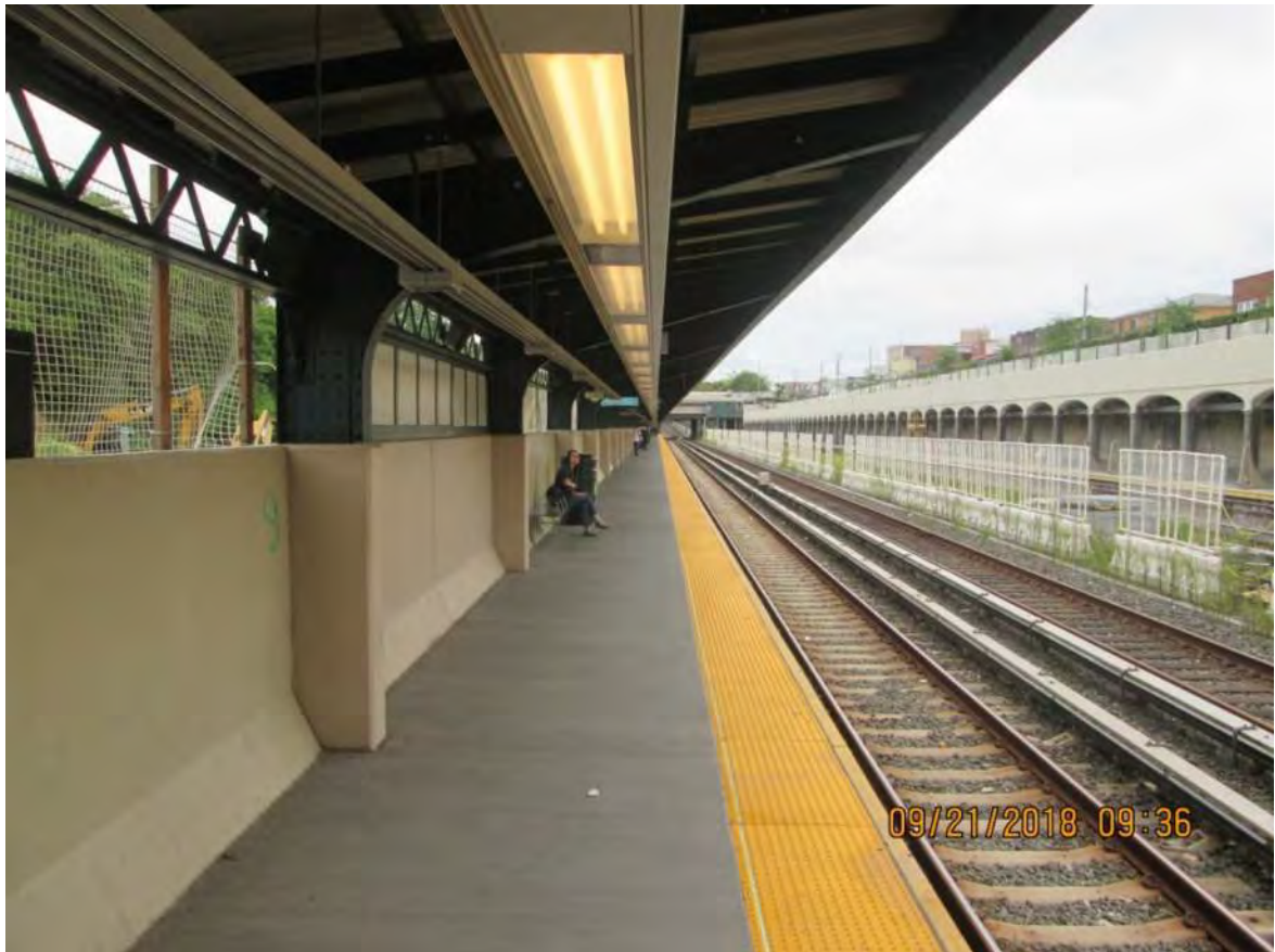
Figure 3 – Typical platform view Fort Hamilton Station
