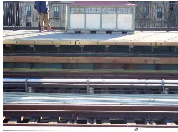
Figure 2 – Precast Slab 167 th Street Station
