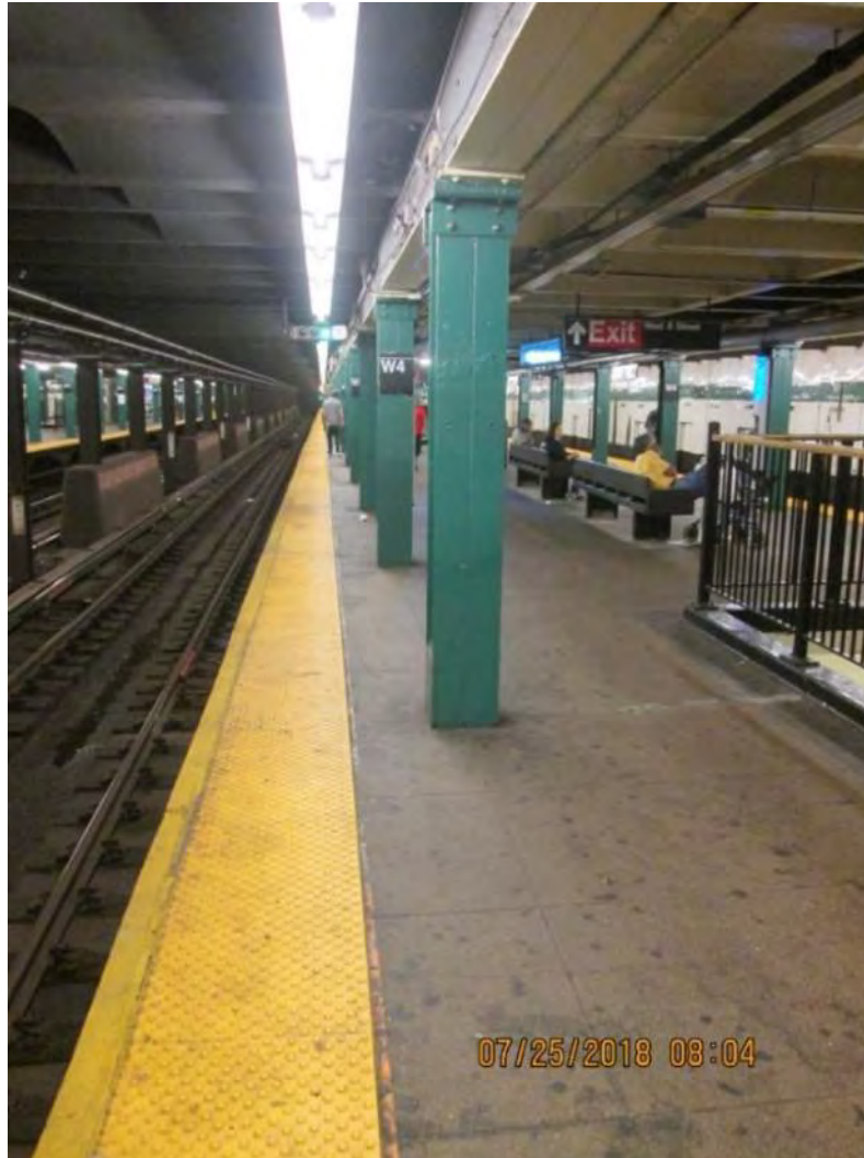
Figure 4 – Typical platform view with signal light West 4 th Street Station
