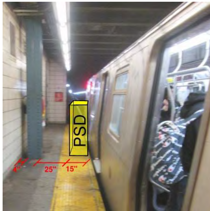
Figure 1 – Non-Compliant ADA condition 45 th Street Station
