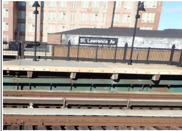
Figure 2 – Precast Slab Saint Lawrence Avenue Station
