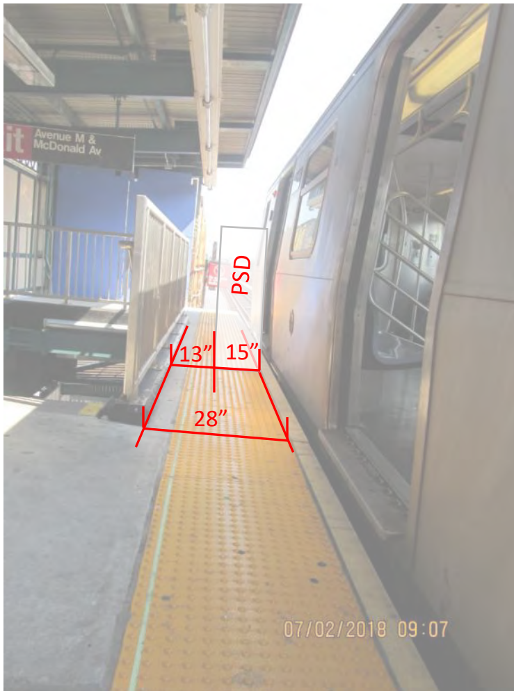
Figure 1– General Platform Condition – Avenue N Station
