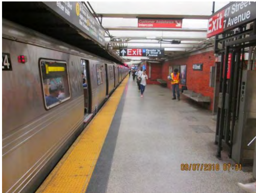
Figure 3 – General platform view 49th Street Station
