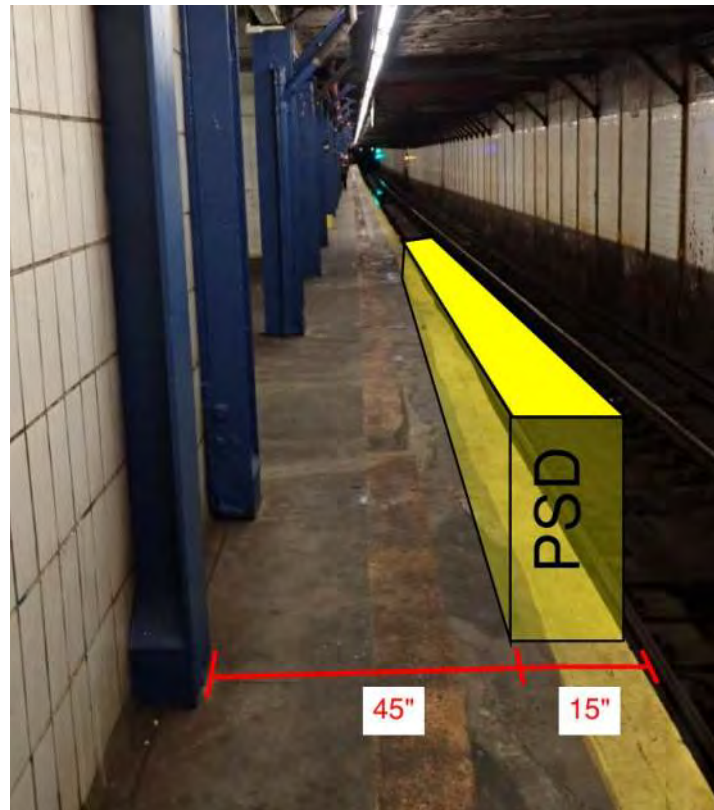
Figure 1 – Non-Compliant egress condition 14 th Street Station
