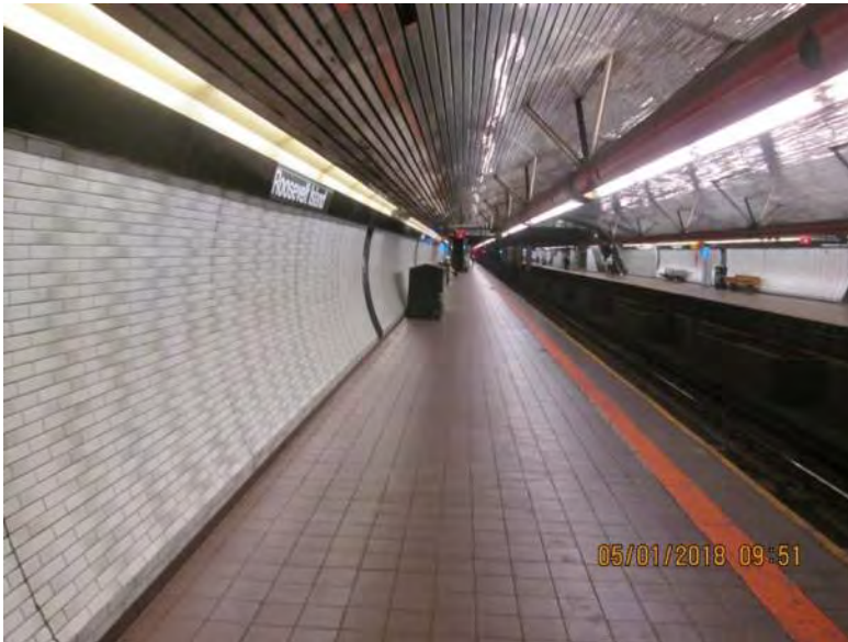
Figure 3 – Typical platform view featuring curved walls and ceilings- Roosevelt Island Station
