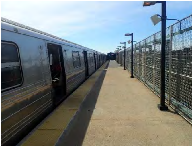
Figure 1 – General Station Condition 79 th Street Station
