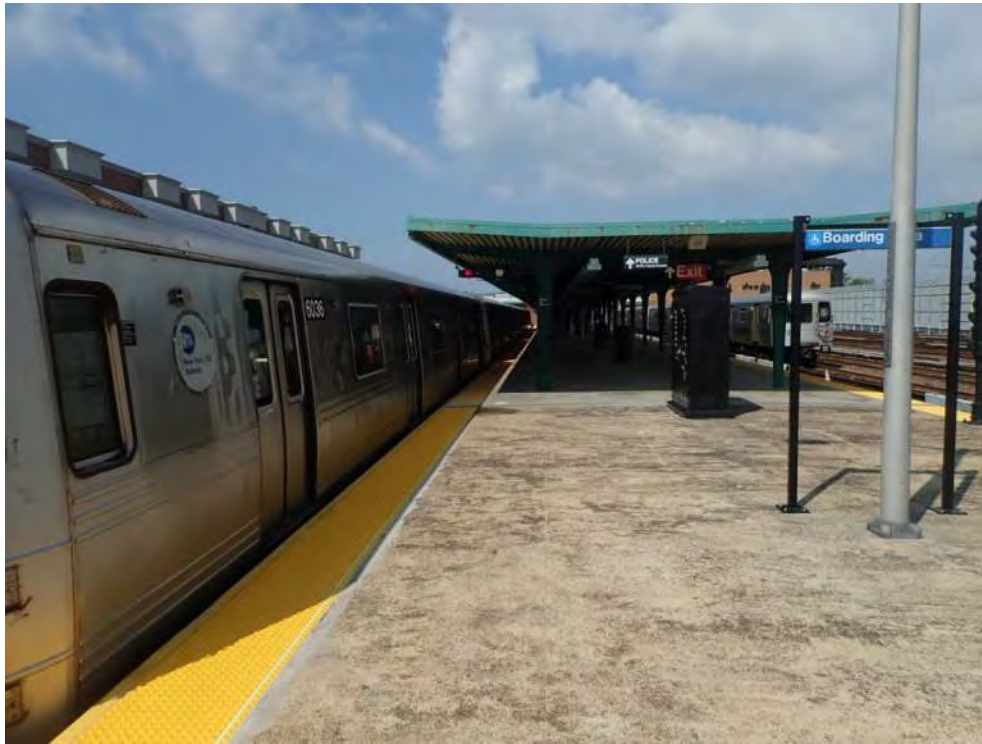
Figure 3 – General platform view Rockaway Park Station
