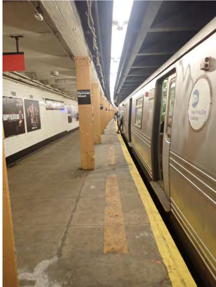
Figure 3 – General platform view Dyckman Street Station
