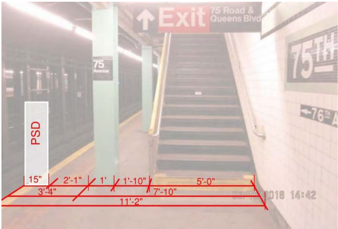
Figure 1 – Non-compliant condition at stairs (typical) - 75 th Avenue
