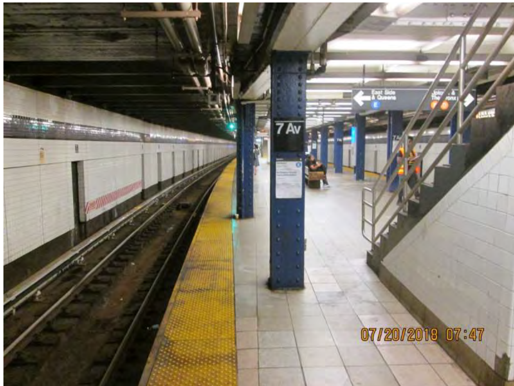
Figure 4 – Typical platform view 7 th Avenue Station
