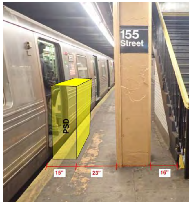
Figure 1 – Area of ADA non-compliance 155 th Street 8 th Ave Station
