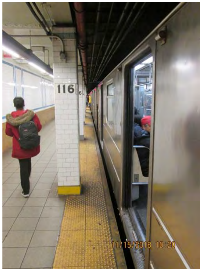
Figure 1 – Column 12” from the edge 116 th Street Station
