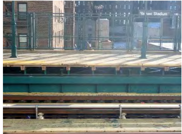
Figure 2 – Precast Slab 161 st Street Station
