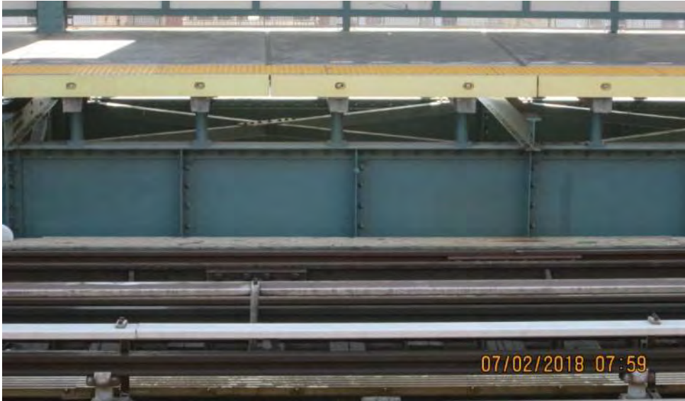
Figure 2– Precast T-Beam platform – Ditmas Avenue Station
