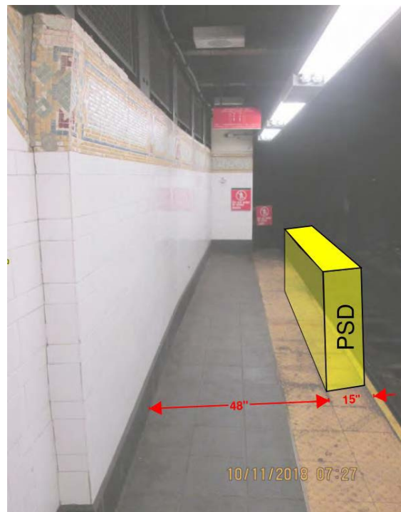
Figure 1 – Non-Compliant code condition Cortlandt Street Station
