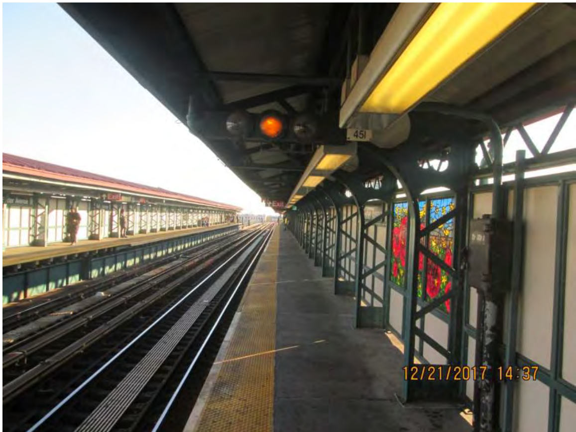
Figure 1 – Typical Platform View- Sutter Avenue Station
