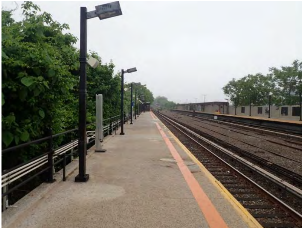
Figure 3 – General platform view Aqueduct North Conduit Station
