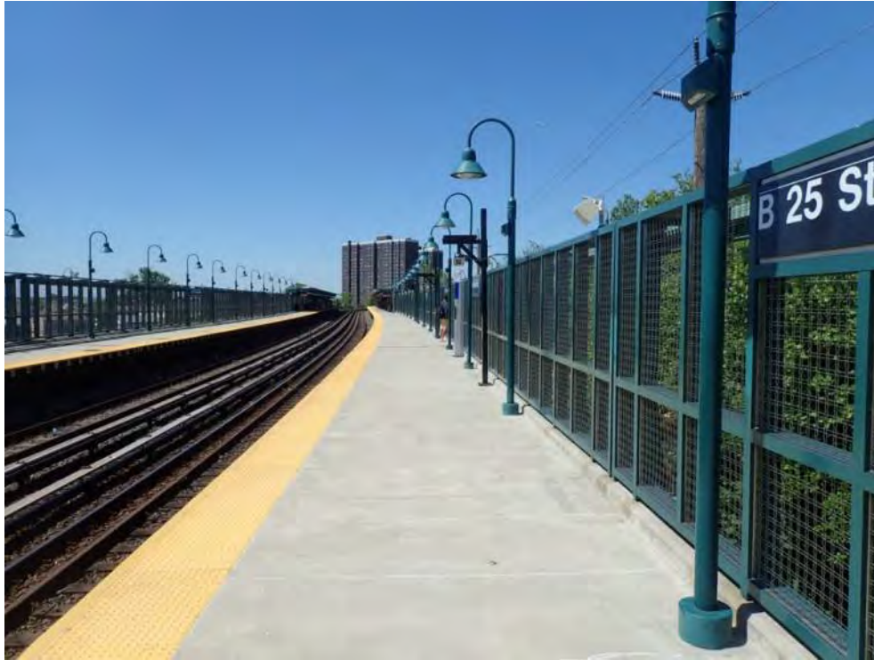
Figure 3 – General platform view Beach 25 th Street Station
