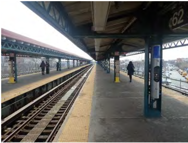
Figure 1 – General Station Condition 62 nd Street Station
