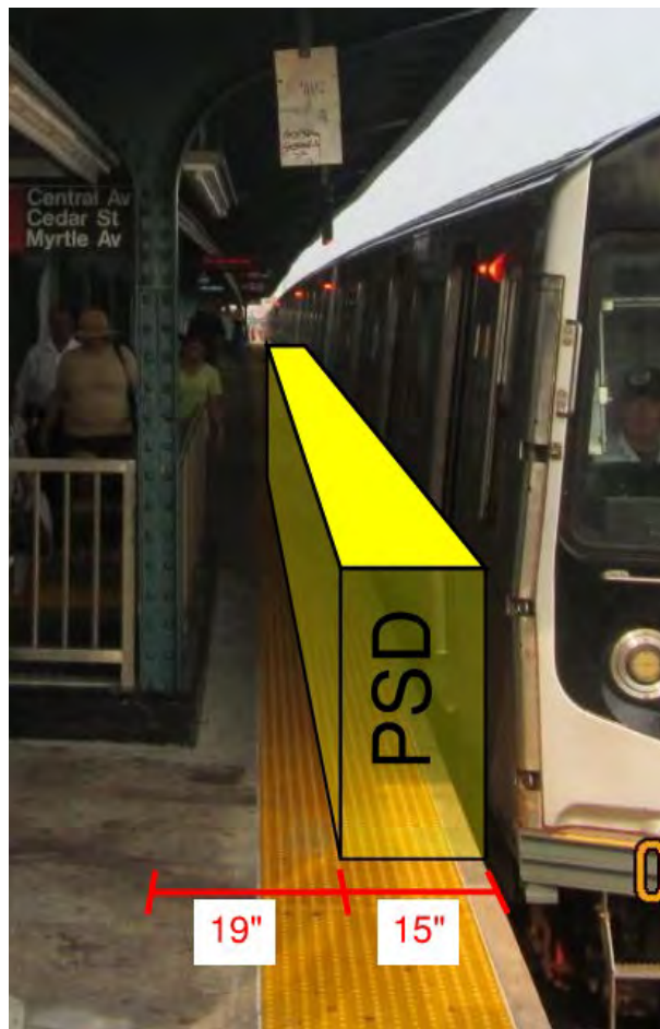
Figure 1 – Non-Compliant ADA condition Central Avenue Station
