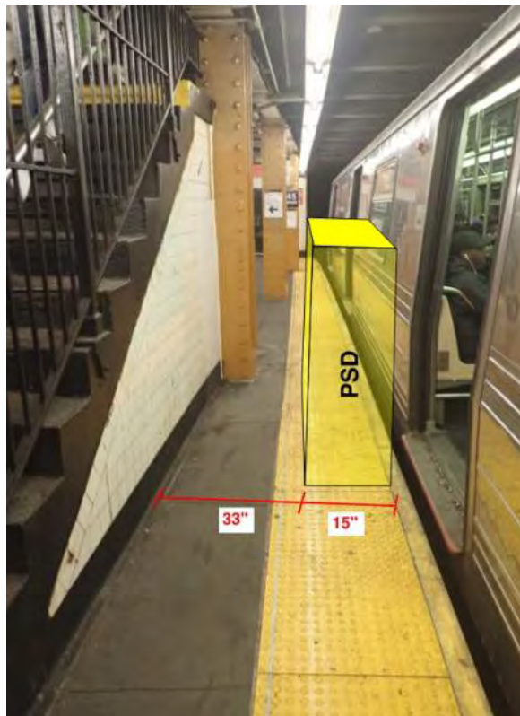
Figure 1 – Non-compliant ADA dimension 145 th Street Station
