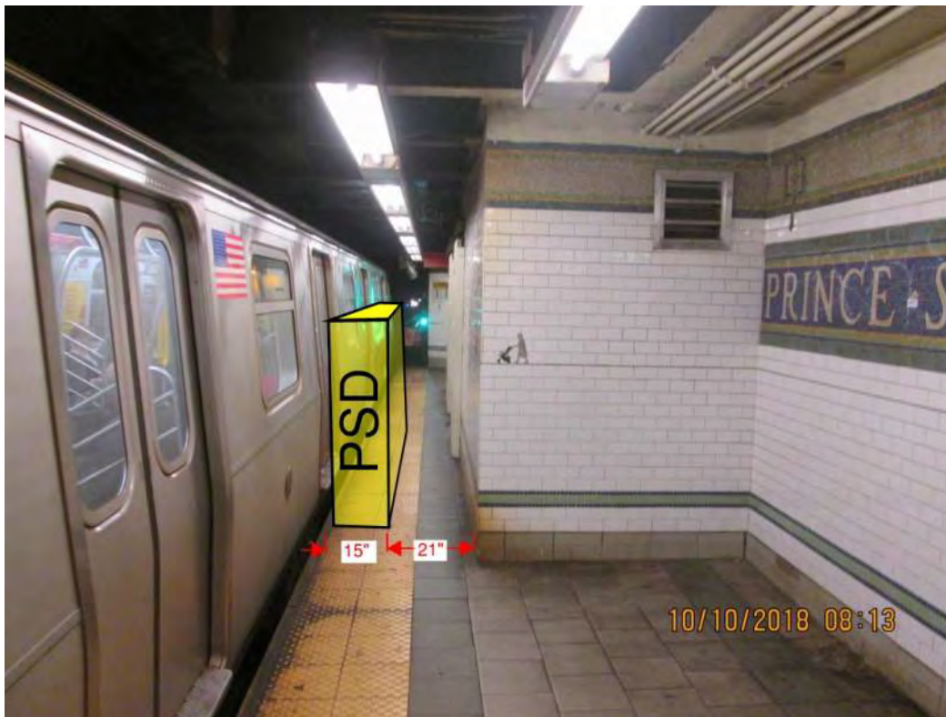
Figure 1 – Non-Compliant ADA condition Prince Street
