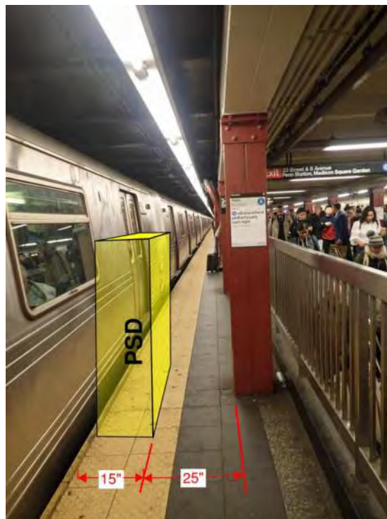
Figure 1 – Non-Compliant ADA condition 34 th Street Penn Station
