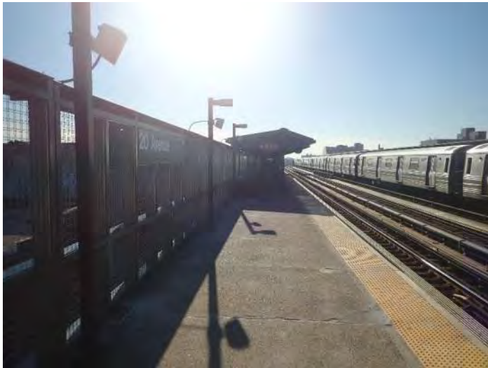
Figure 1 – General Station Condition 20 th Avenue Station
