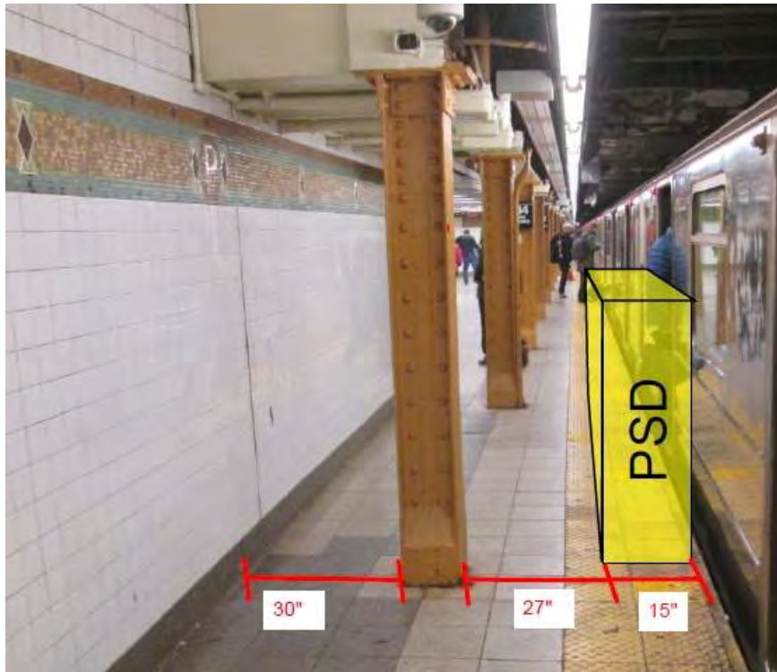
Figure 1 – Non-Compliant egress condition 34 th Street Station
