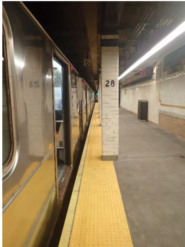
Figure 1 – Column 14” from the edge 28th Street Station
