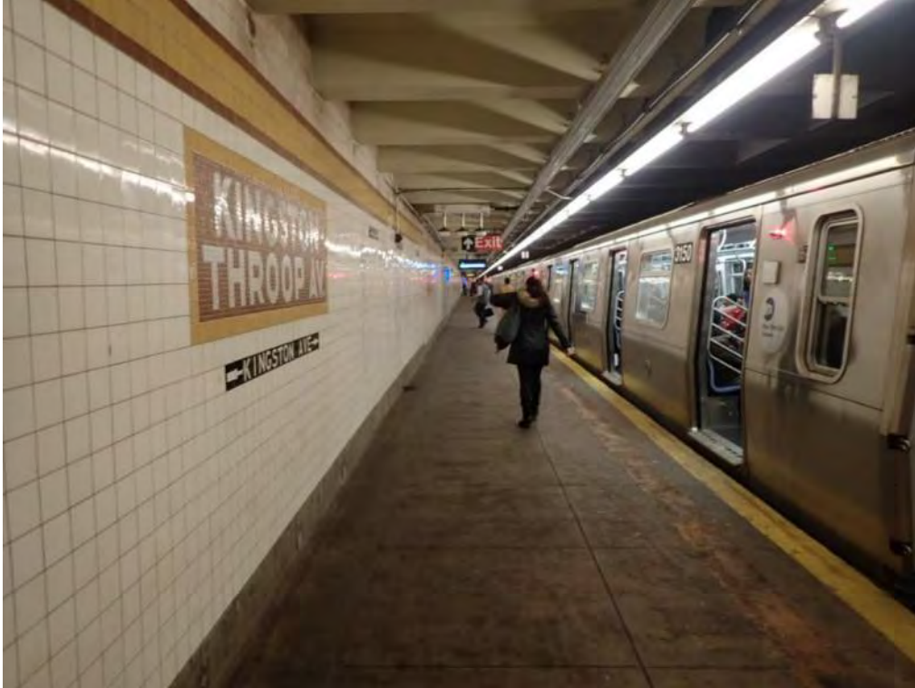
Figure 3 – General platform view Kingston Throop Station
