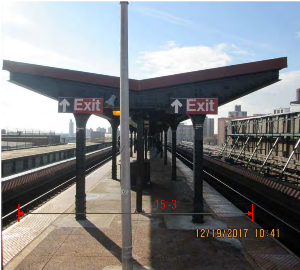
Figure 1 – General view of platform width and canopy – Atlantic Avenue Station
