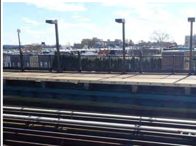
Figure 2 – Precast Slab Castle Avenue Station
