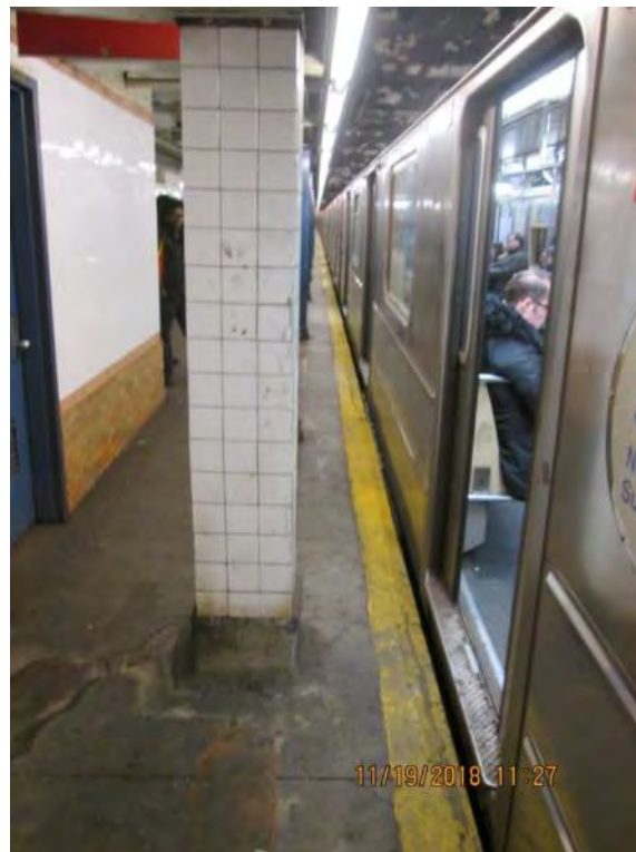
Figure 1 – Column 16” from the edge 86 th Street Station
