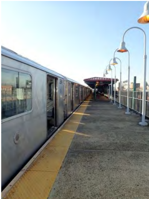
Figure 1 – General Station Condition 238 th Street Station
