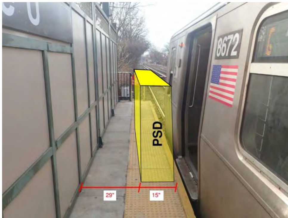
Figure 1 – Area of ADA non-compliance Avenue U Station
