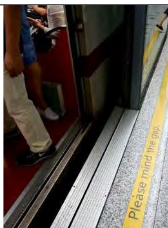
Figure 7 - Shanghai: End of platform light detection
