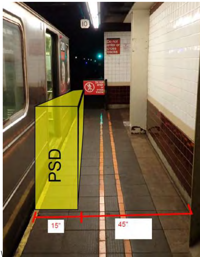
Figure 1 – Non-Compliant egress condition 18 th Street Station
