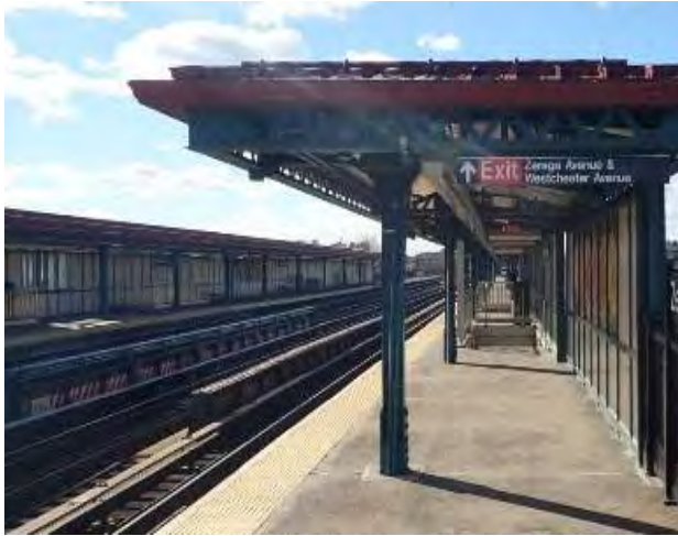
Figure 1 – General Station Condition Zerega Avenue Station
