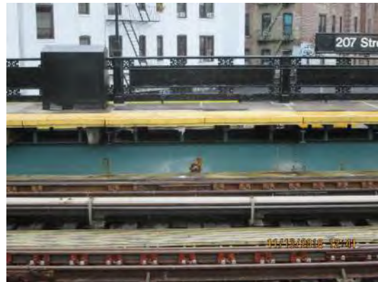
Figure 2 – Precast concrete platforms 207 th Street Station
