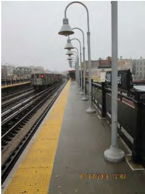
Figure 1 – General Station Condition 238 th Street Station
