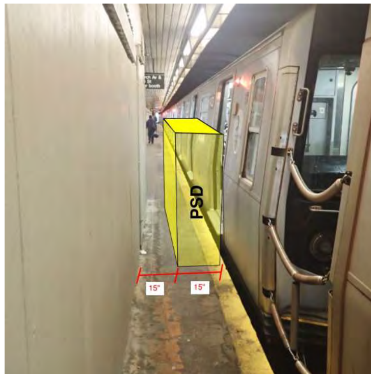
Figure 1 – Area of ADA non-compliance Church Avenue
