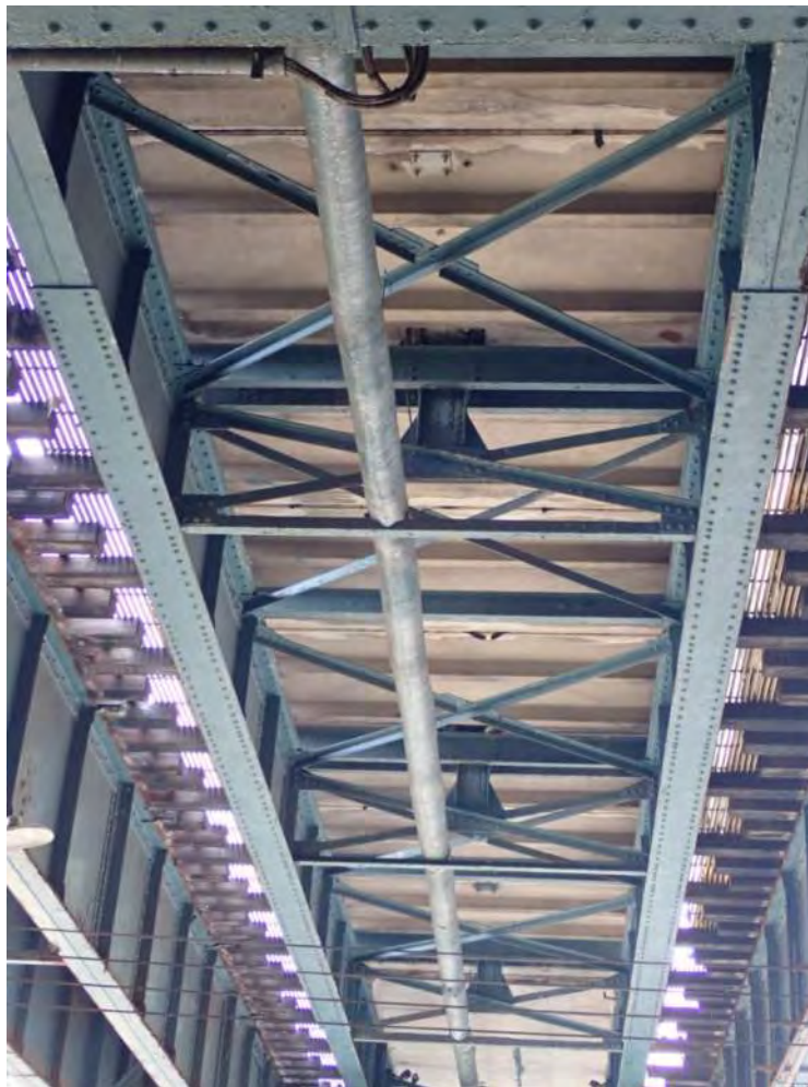
Figure 1 – Precast Slab New Lots Avenue Station
