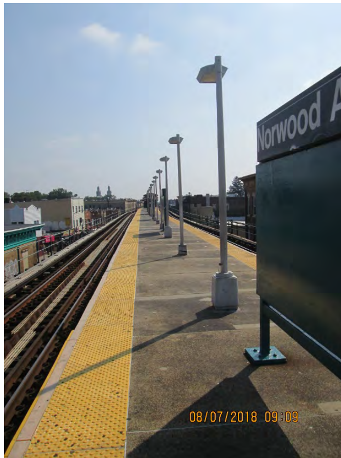
Figure 1 – Precast platform Norwood Avenue Station
