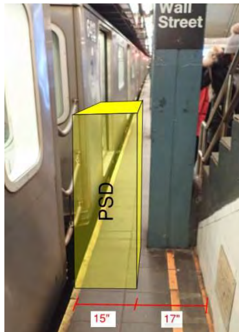
Figure 1 – Non-compliant ADA condition Wall Street Station
