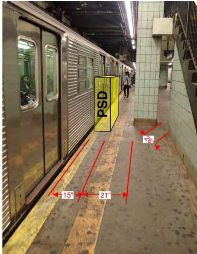
Figure 1 – Non-Compliant ADA condition Grant Avenue
