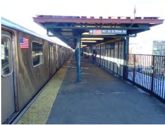
Figure 1 – General Station Condition 167 th Street Station
