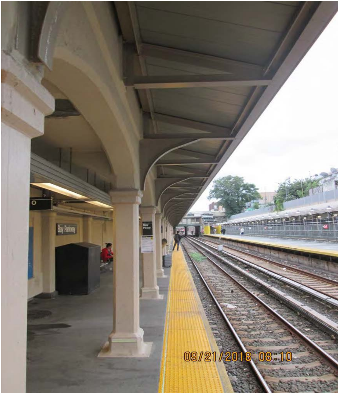
Figure 3 – Typical platform view Bay Parkway Station
