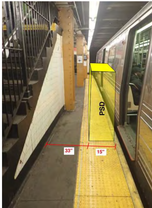
Figure 1 – Non-compliant ADA dimension 145 th Street Station
