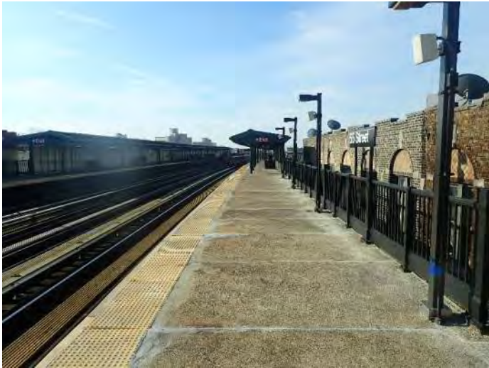
Figure 1 – General Station Condition 55 th Street Station
