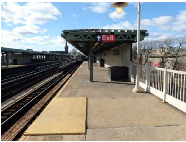
Figure 1 – General Station Condition Westchester Square East Tremont Station
