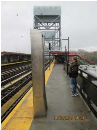
Figure 1 – Overall view 225 th Street Station
