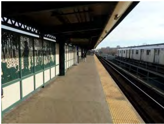
Figure 1 – General Station Condition Van Siclen Avenue Station
