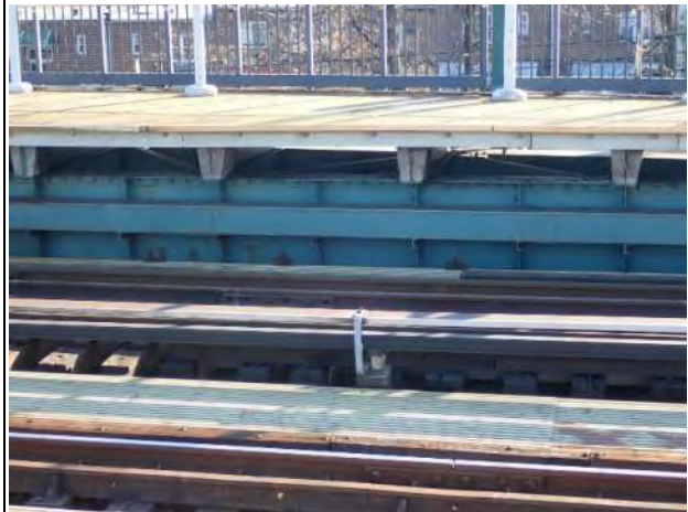
Figure 2 – Precast Slab Middletown Road Station
