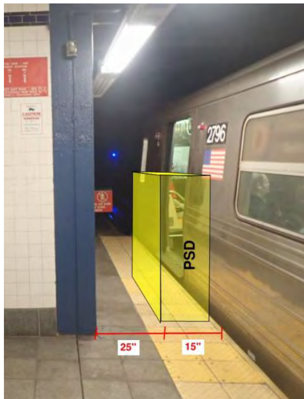
Figure 1 – Non-Compliant ADA condition 81st St. Station
