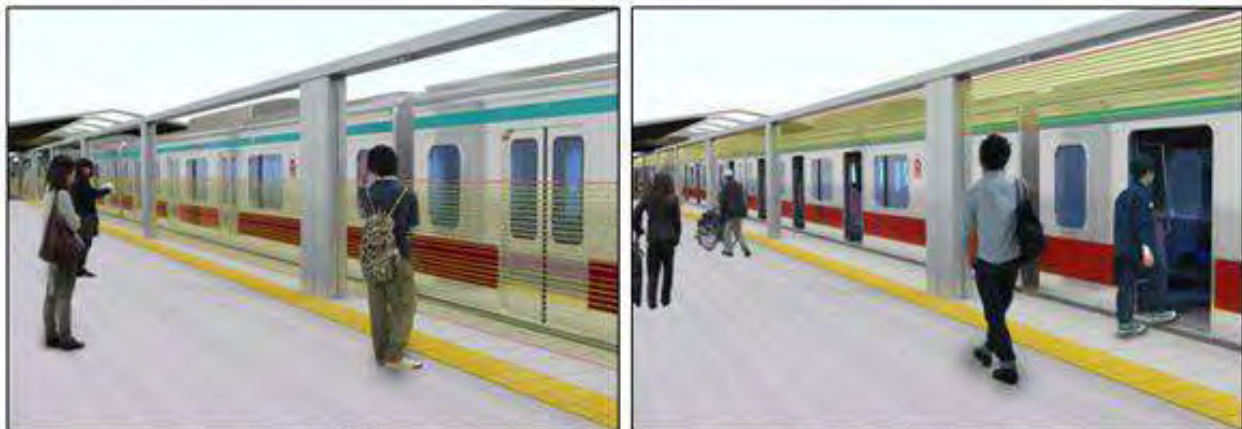
Photo 3 – Roped Platform Screen Doors, (closed in left image, open in right image)
