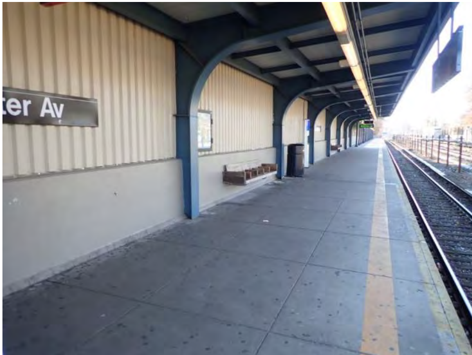
Figure 3 – Typical platform view Baychester Avenue Station
