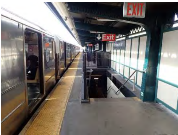
Figure 1 – General Station Condition Rockaway Avenue Station
