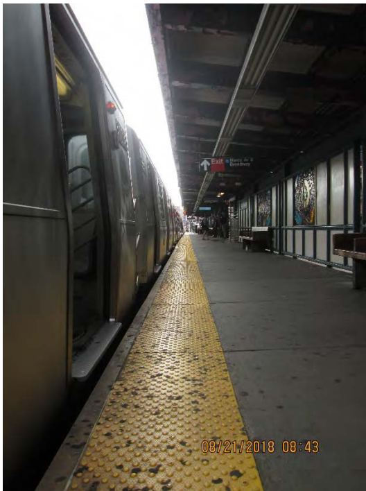
Figure 1 – General Station condition Marcy Avenue Station
