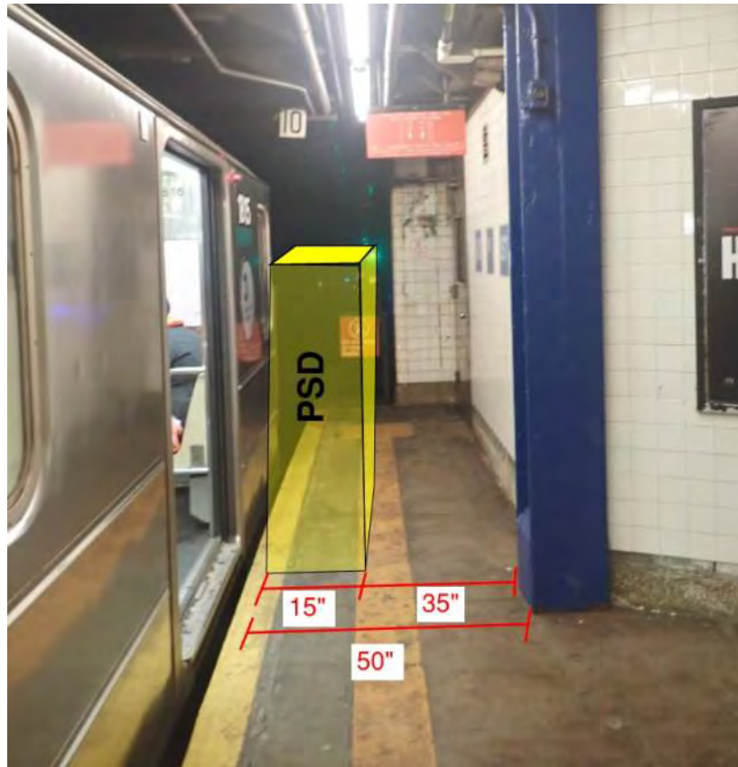
Figure 1 – Non-Compliant egress condition 68th Street Hunter College Station
