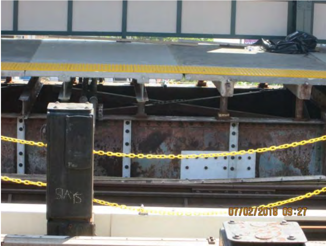
Figure 2– Precast T-Beam platform – Avenue P Station
