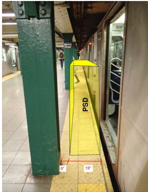
Figure 1 – Non-compliant ADA condition Nevins Street Station
