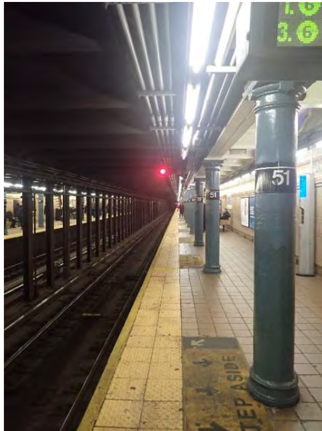
Figure 3 – Typical platform view 51 st Street Station
