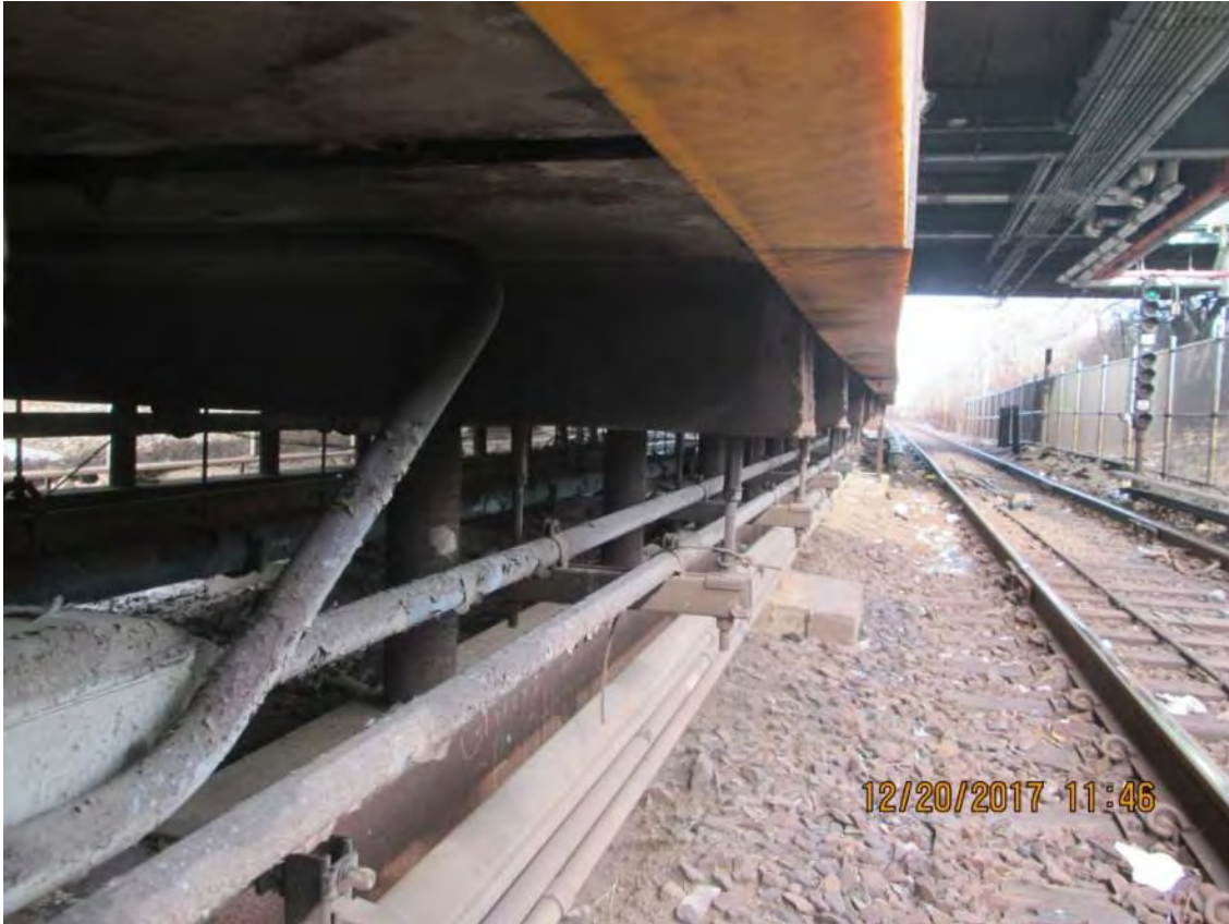
Figure 2– Precast T-Beam platform – East 105th Station
