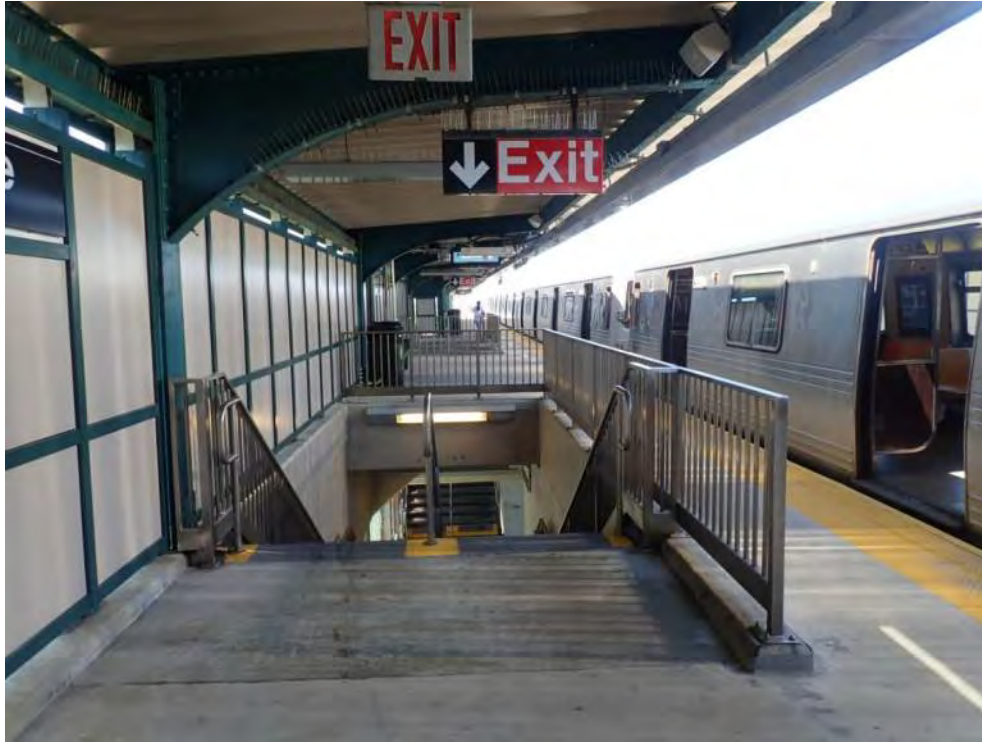
Figure 3 – General platform view Beach 36 th Street Station
