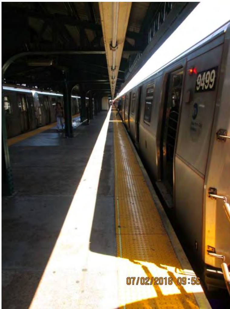
Figure 1– General Platform Condition – Kings Highway Station
