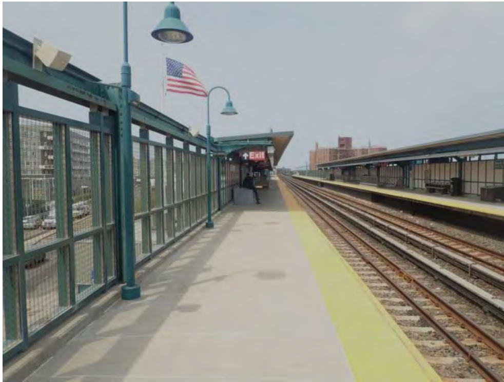
Figure 3 – General platform view Beach 67 th Street Station
