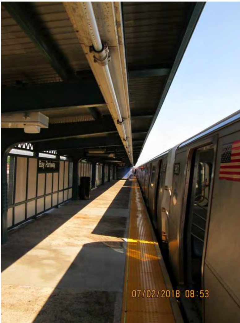
Figure 1– General Platform Condition – Bay Parkway Station
