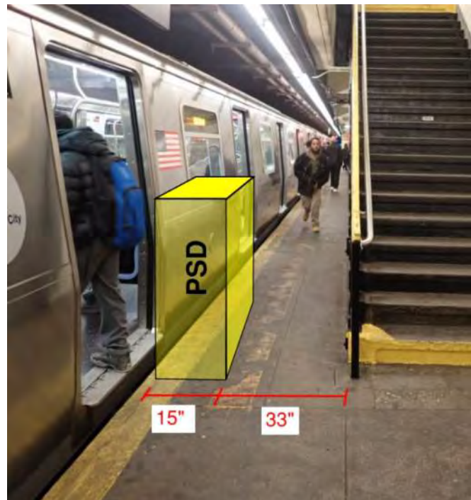
Figure 1 – Non-Compliant ADA condition Nostrand Avenue Station – lower level C-train platform
