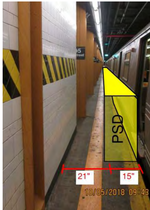
Figure 1 – Column 1’-2” from the edge 95 th Street Station
