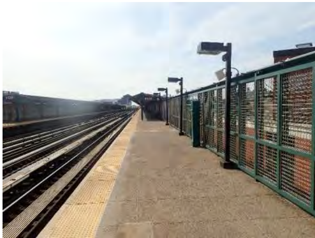
Figure 1 – General Station Condition Fort Hamilton Station
