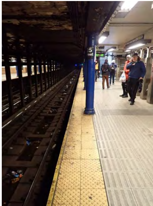
Figure 1 – Column 16” from the edge 125 th Street Station
