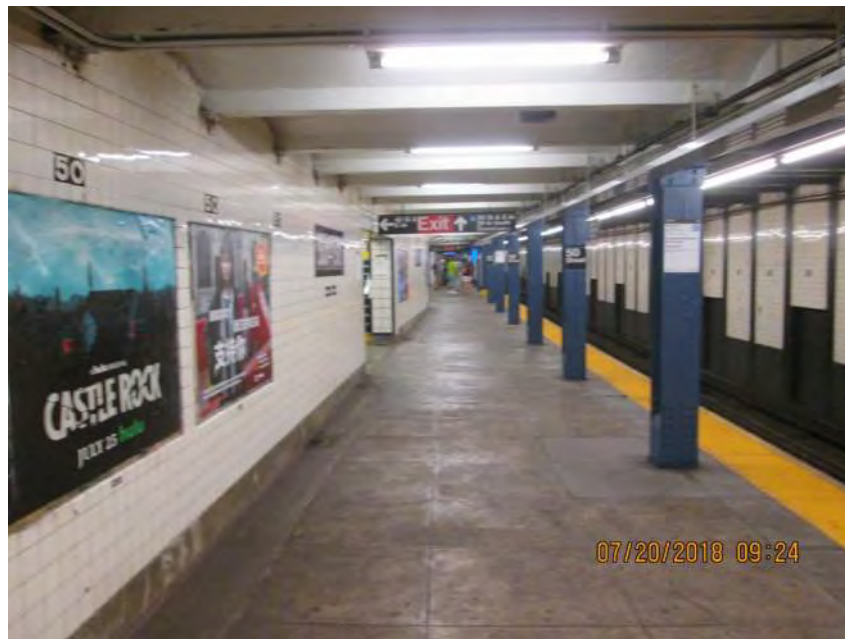
Figure 3 – Typical view – lower platform 50 th Street Station
