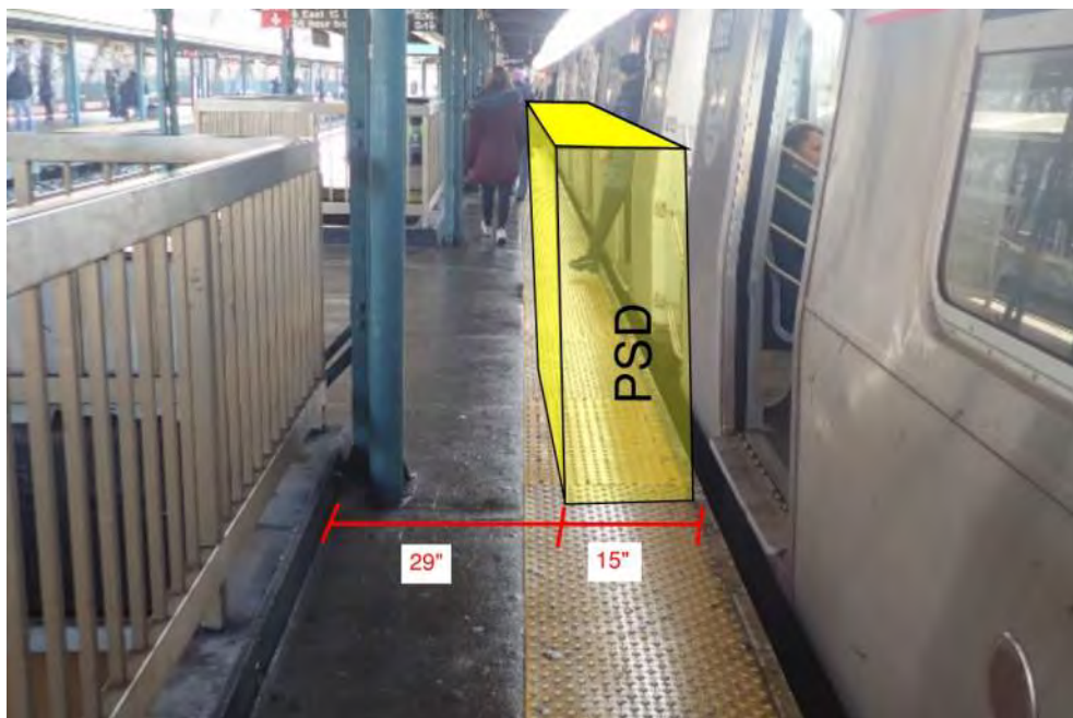
Figure 1 – Area of ADA non-compliance Sheepshead Bay Station
