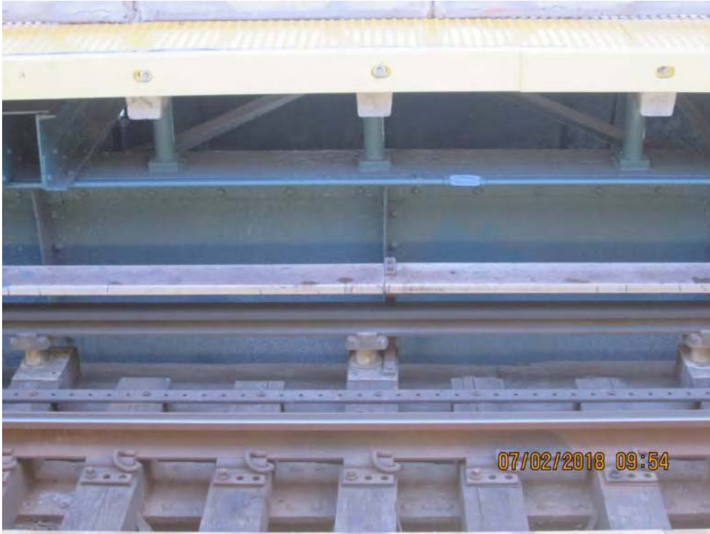
Figure 2– Precast T-Beam platform – Kings Highway Station
