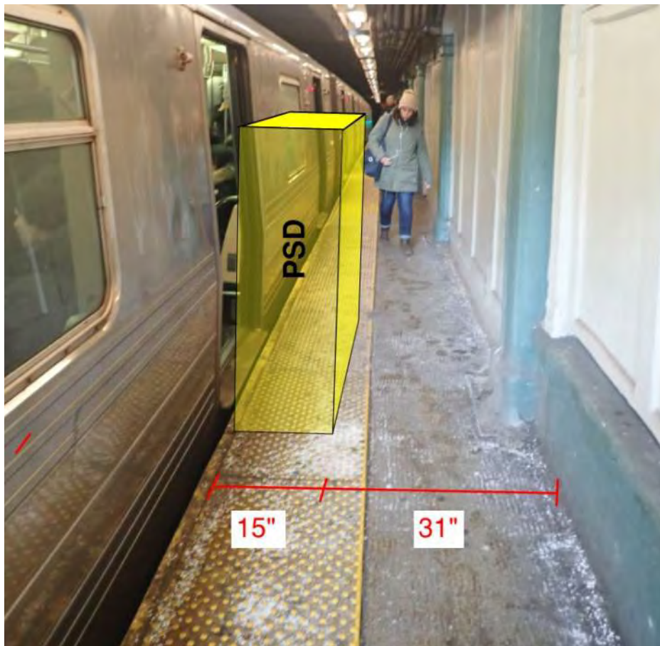
Figure 1 – Non-compliant ADA condition Prospect Park Station
