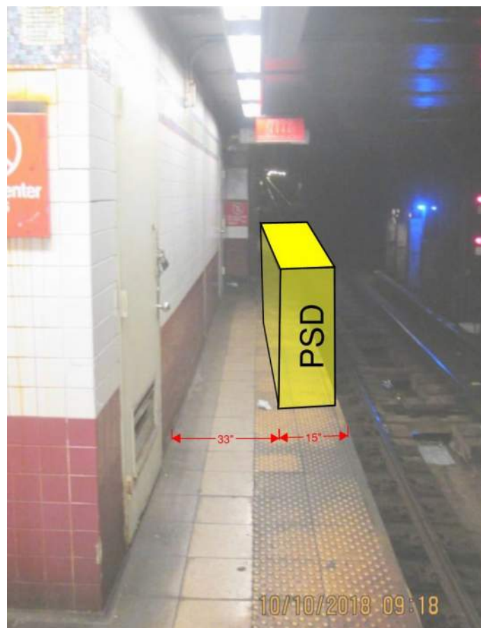
Figure 1 – Non-Compliant ADA condition Canal Street Station
