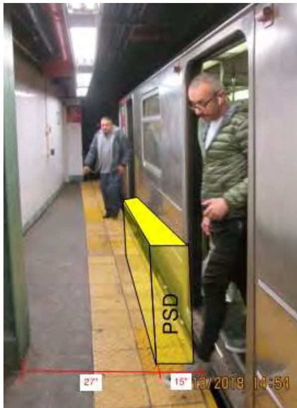
Figure 1 – Non-Compliant ADA condition 42nd Street Station
