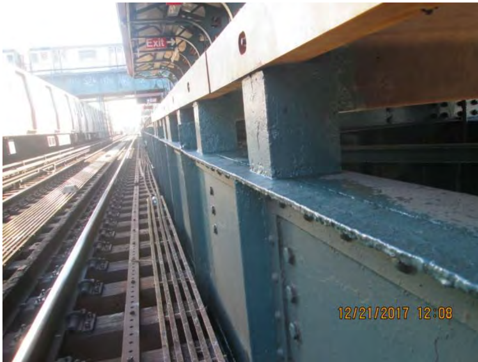
Figure 3 – Elevated Precast T-Beam platform – Livonia Avenue Station
