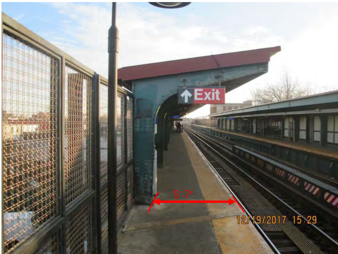
Figure 1—Columns are typically 5'-7" from the platform edge— New Lots Avenue Station
