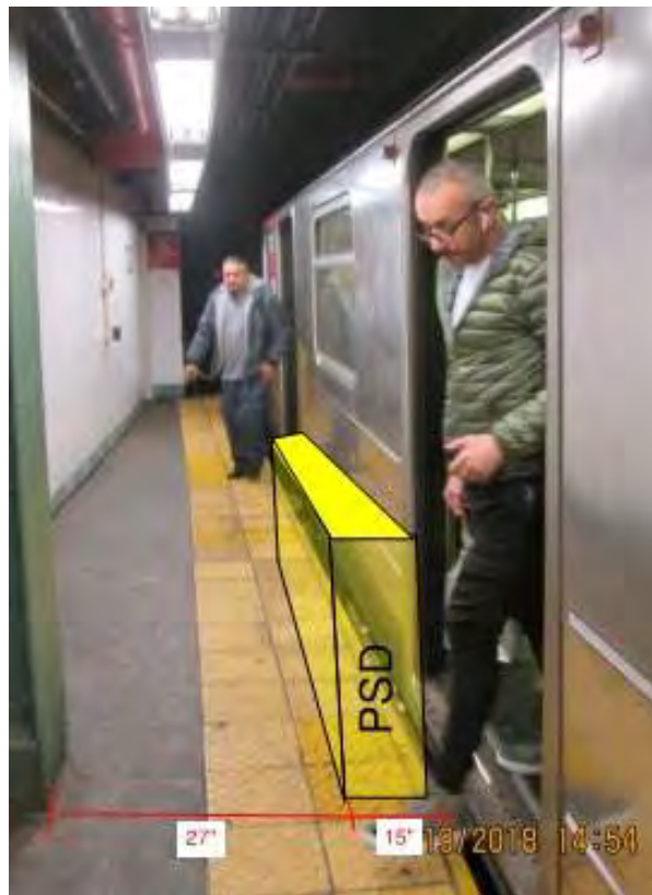
Figure 1 – Non-Compliant ADA condition 42nd Street Station
