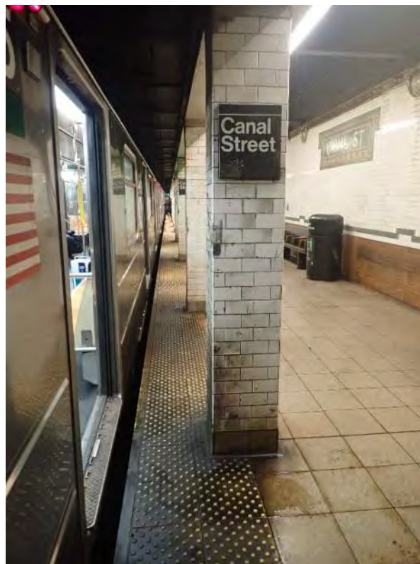
Figure 1 – Column 16” from the edge Canal Street Station
