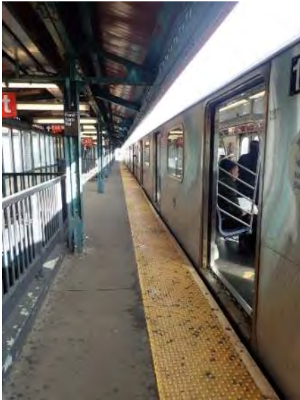
Figure 1 – General Station Condition Fordham Road Station
