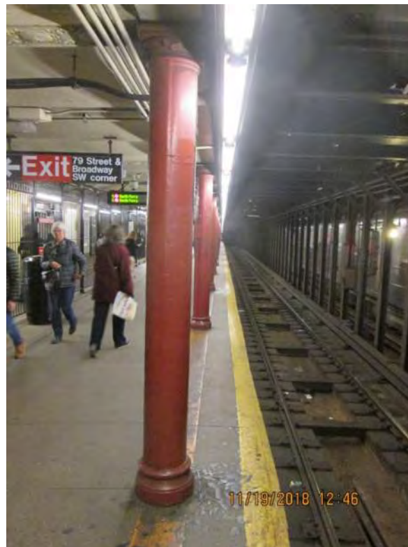
Figure 1 – Column 15” from the edge 79 th Street Station
