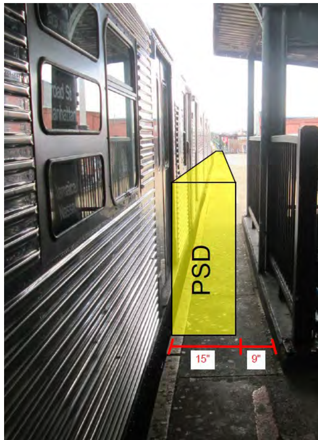
Figure 1 – Non-Compliant ADA condition 75th Street-Elders Lane Station
