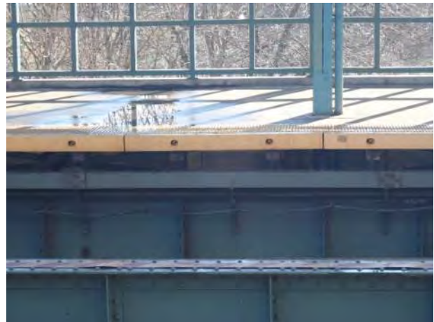
Figure 2 – Precast Slab Mosholu Parkway Station
