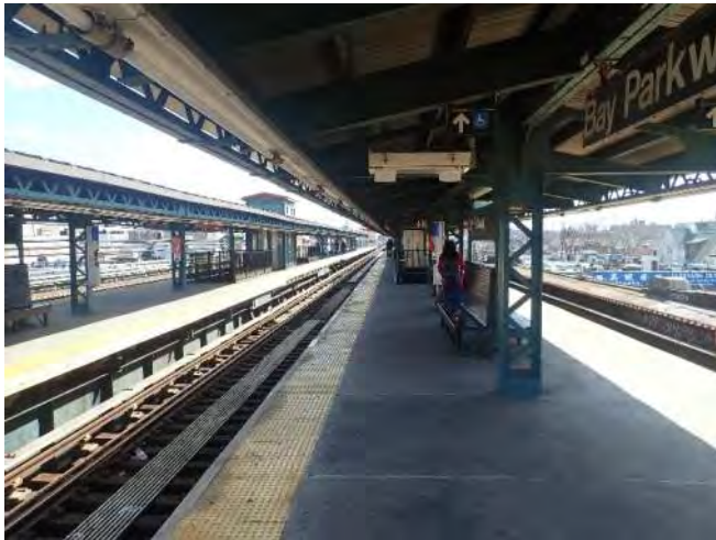
Figure 1 – General Station Condition Bay Parkway Station
