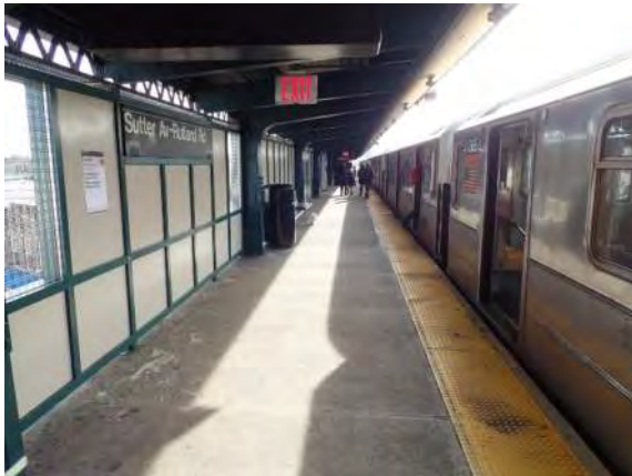
Figure 1 – General Station Condition Sutter Avenue Station
