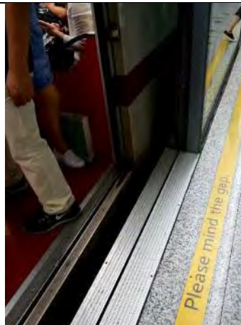
Figure 7 - Shanghai: End of platform light detection
