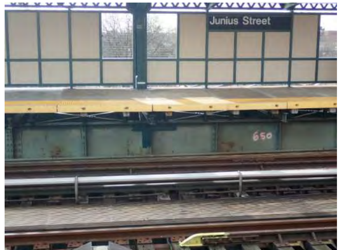
Figure 2 – Precast Slab Junius Street Station
