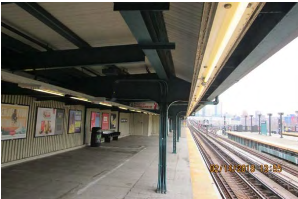
Figure 4 – Typical platform view- Mets-Willets Station
