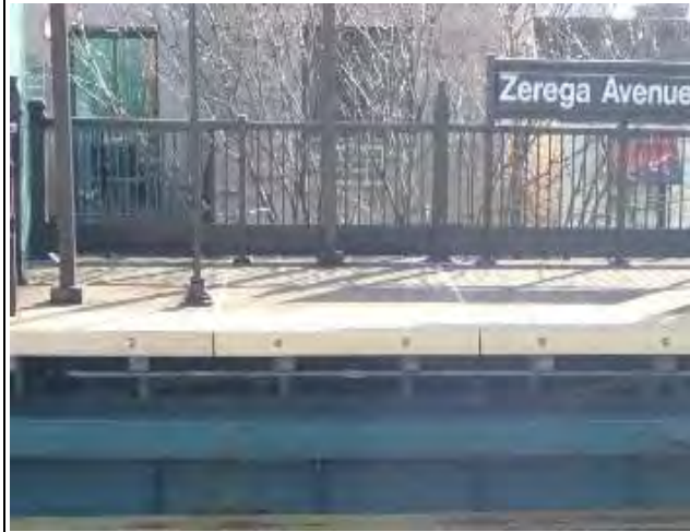
Figure 2 – Precast Slab Zerega Avenue Station
