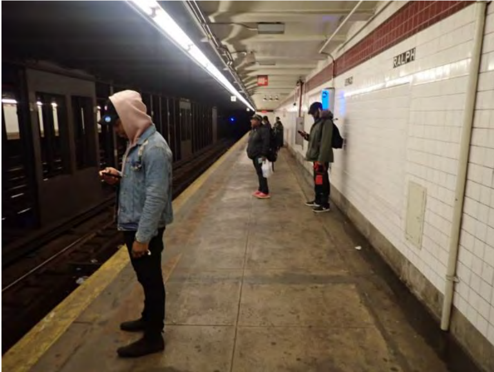
Figure 3 – General platform view Ralph Avenue Station
