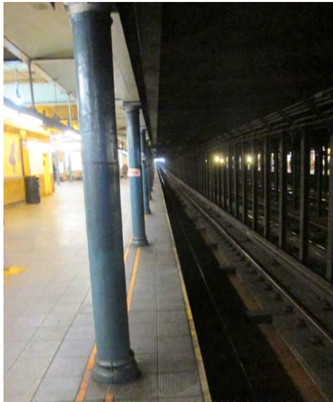
Figure 1 – Column 18” from the edge 50 th Street Station
