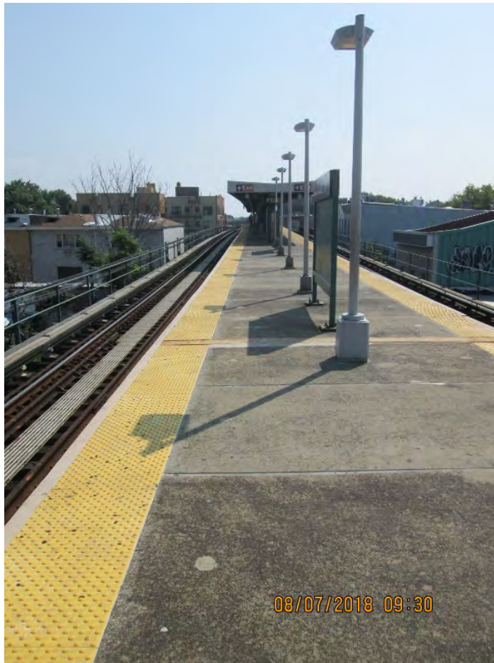
Figure 1 – Precast platform Van Siclen Avenue Station
