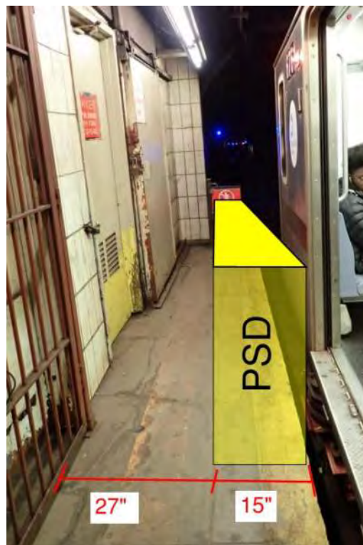
Figure 1 – Non-compliant ADA condition President Street Station
