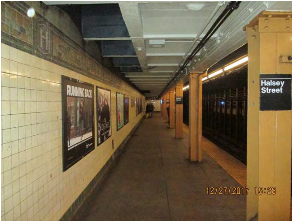
Figure 3– Typical Platform View– Halsey St Station
