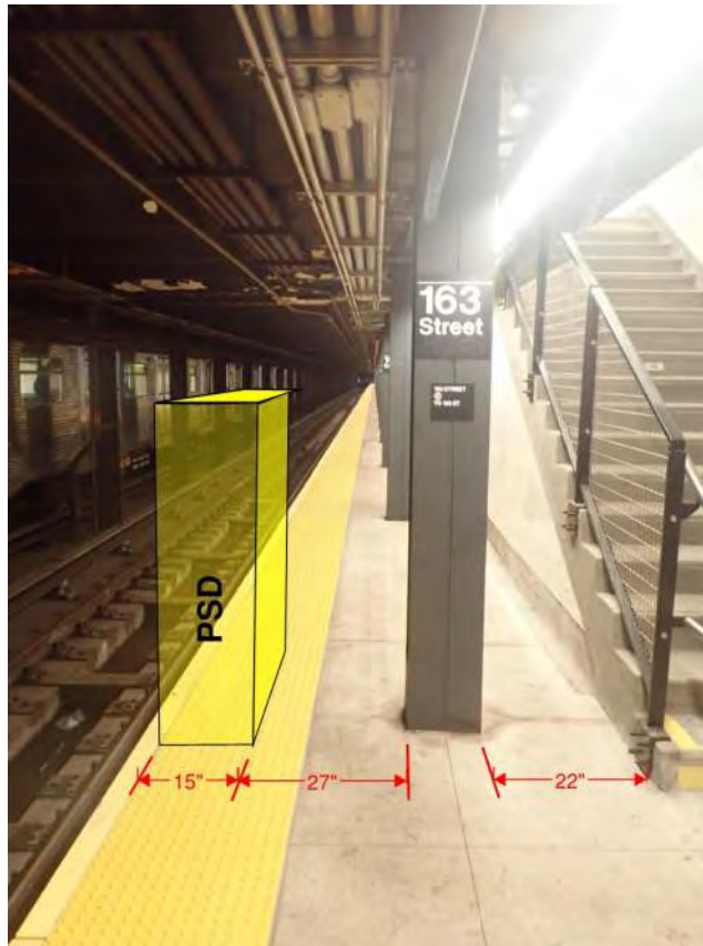
Figure 1 – Non-Compliant ADA condition 163 rd Street Station
