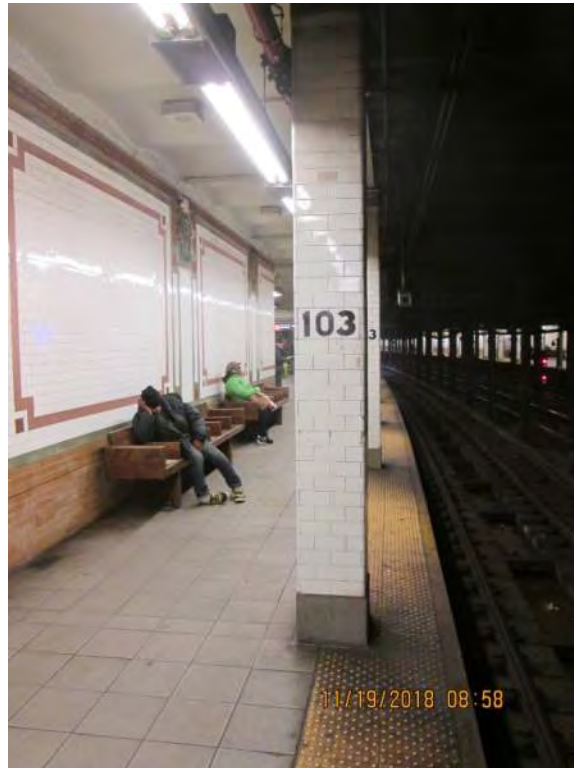
Figure 1 – Column 12” from the edge 103rd Street
