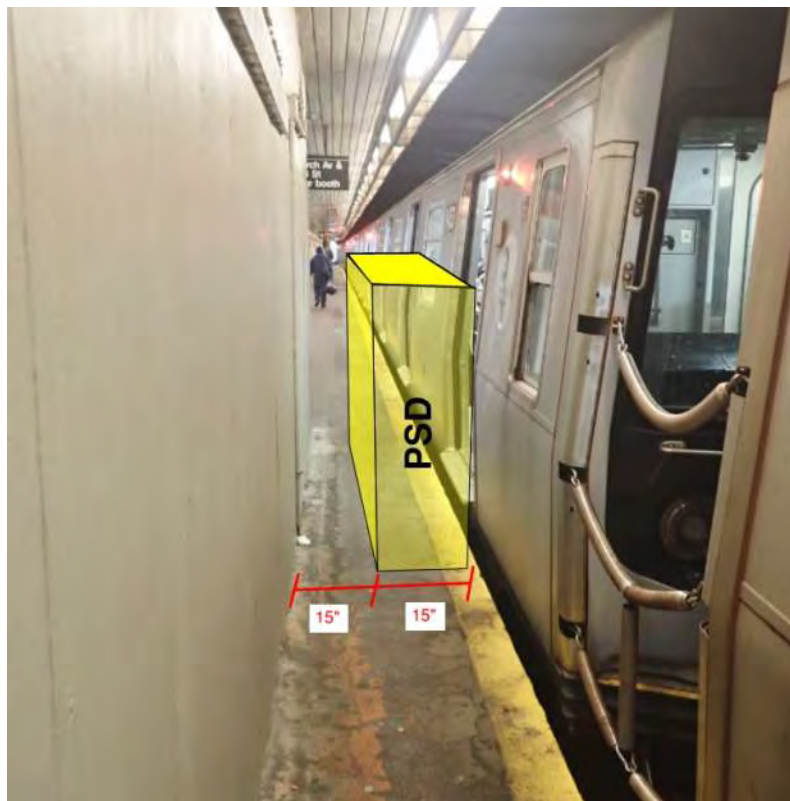
Figure 1 – Area of ADA non-compliance Church Avenue Station
