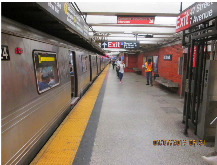
Figure 3 – General platform view 49th Street Station
