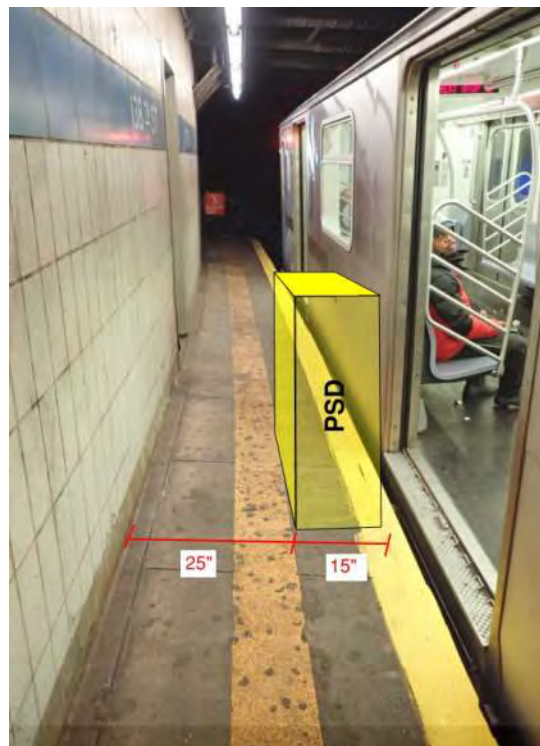
Figure 1 – Non-compliant ADA condition 138 th Street Grand Concourse Station
