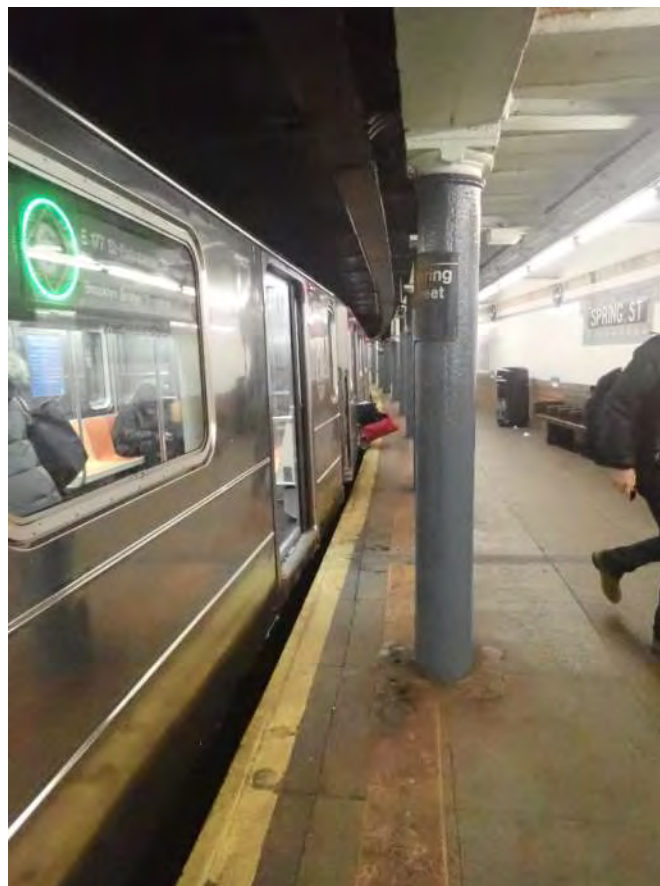
Figure 1 – Column 22” from the edge Spring St. Station
