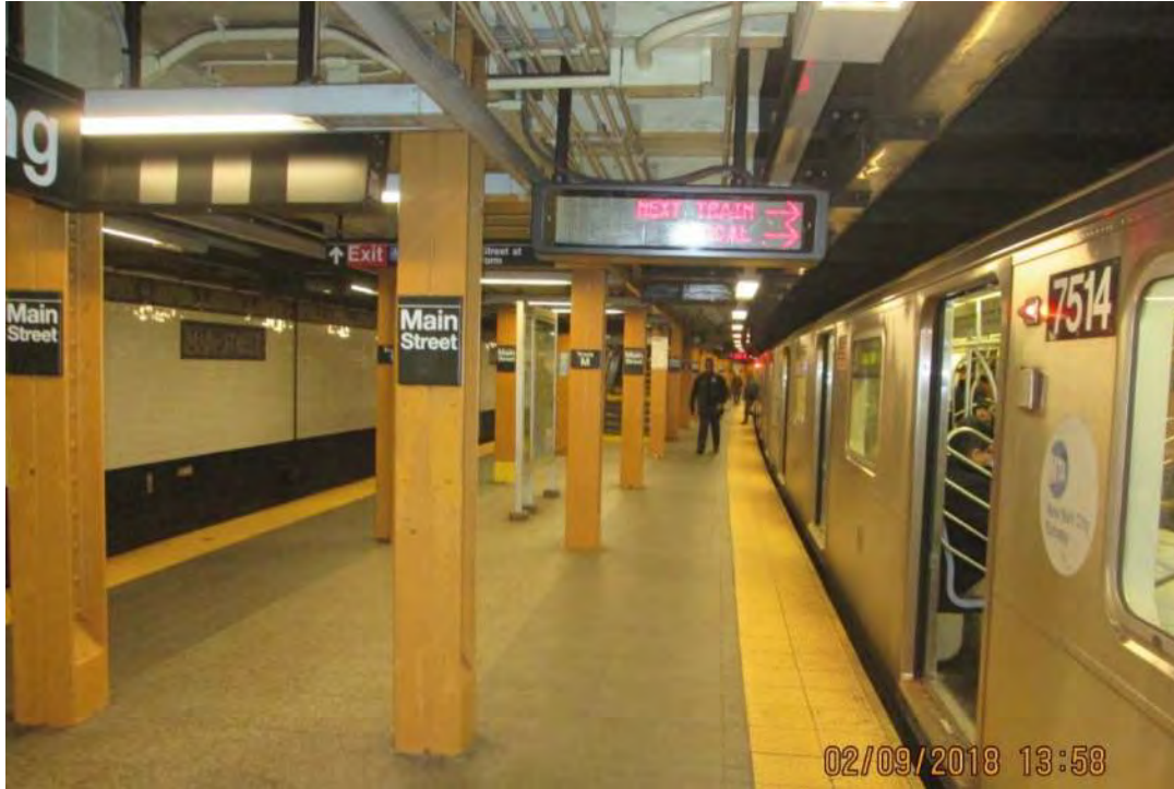
Figure 3 – Typical platform view- Flushing-Main Street Station
