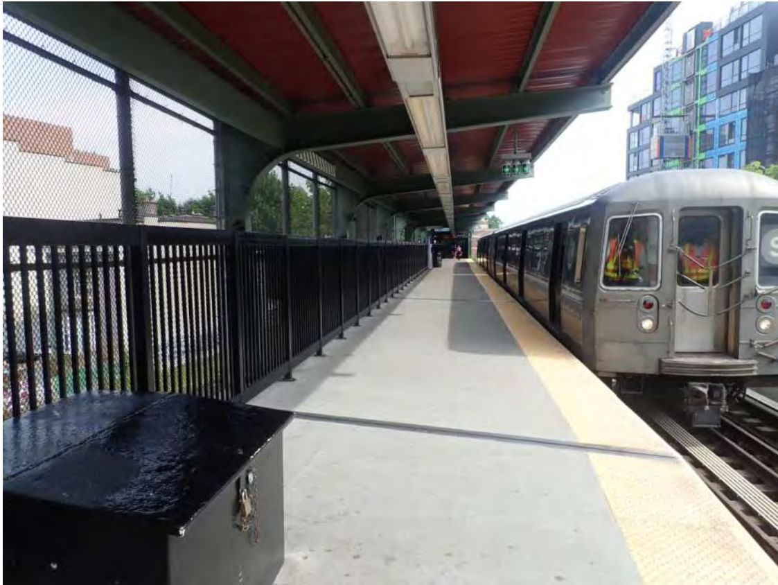
Figure 3 – General platform view Franklin Avenue Station
