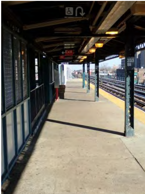
Figure 1 – General Station Condition 233 rd Street Station
