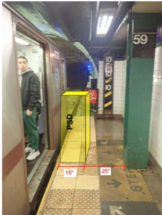
Figure 1 – Non-Compliant egress condition 59 th Street Station- lower level
