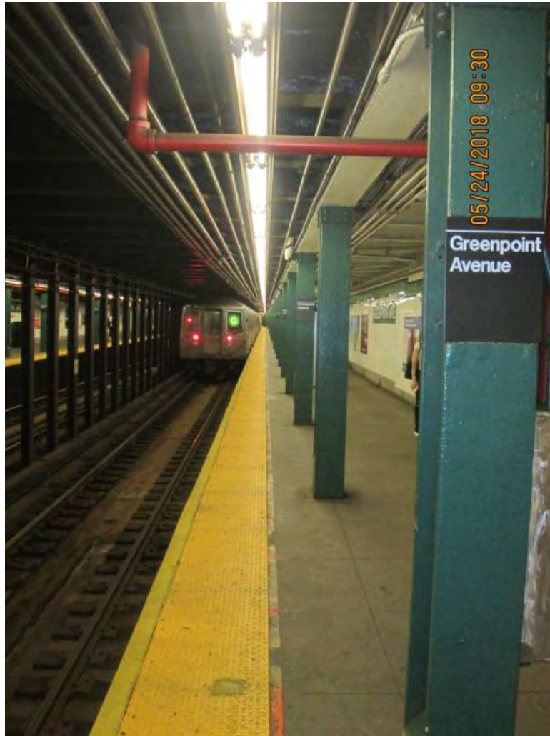
Figure 3 – Typical platform view with standpipe MRN 283 – Greenpoint Avenue
