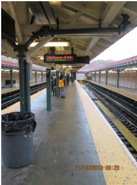
Figure 1 – General Station Condition 242 nd Street Station
