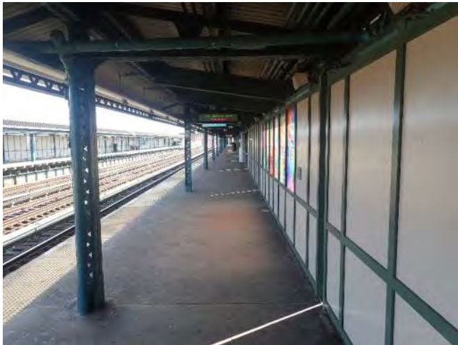
Figure 1 – General Station Condition 25 th Avenue Station
