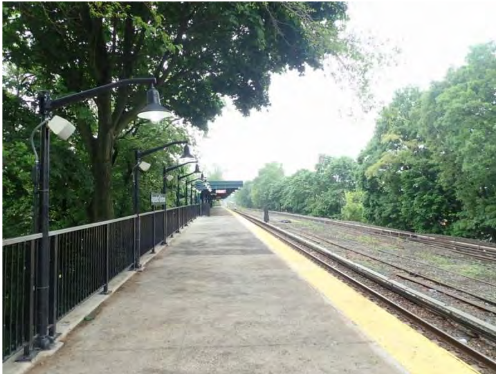
Figure 3 – General platform view Aqueduct Racetrack Station
