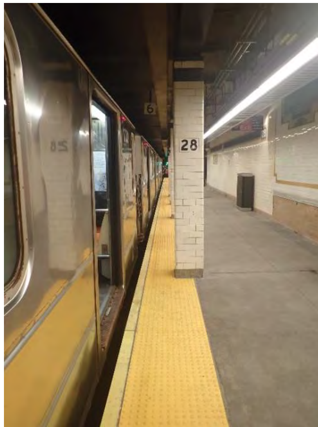
Figure 1 – Column 14” from the edge 28th Street Station
