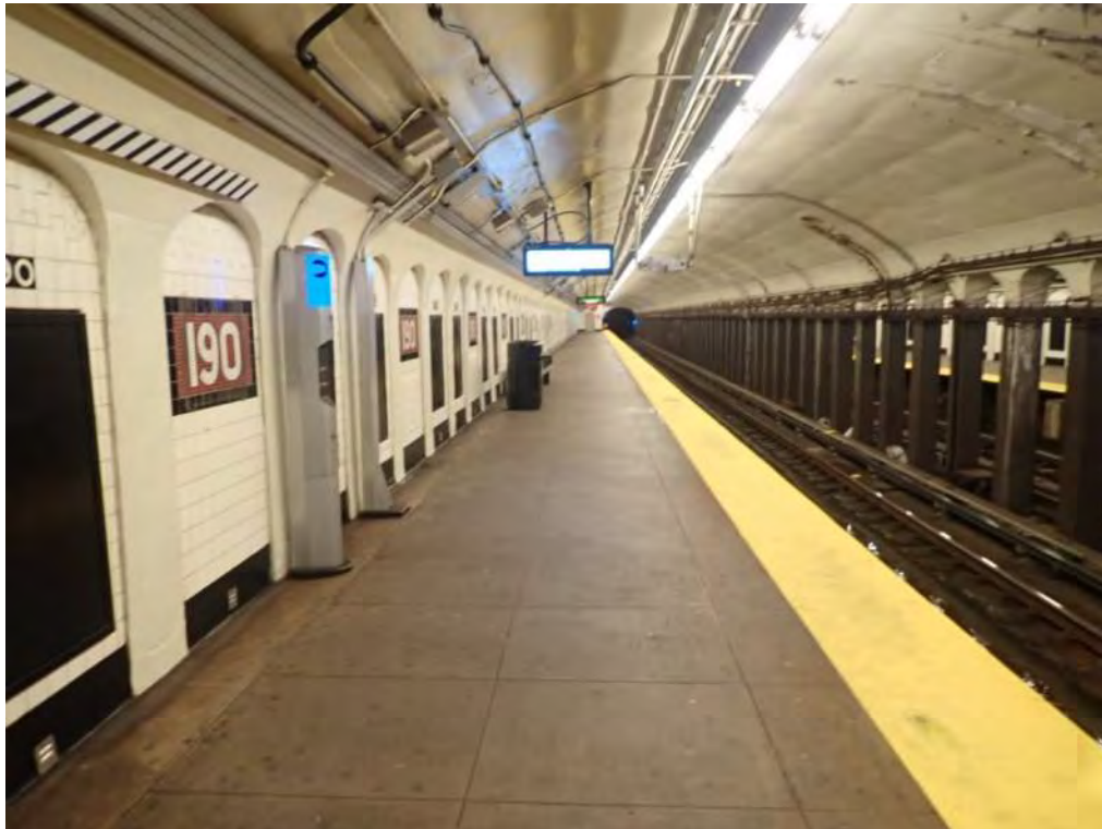
Figure 3 – General platform view 190th Street Ft. Washington Avenue Station
