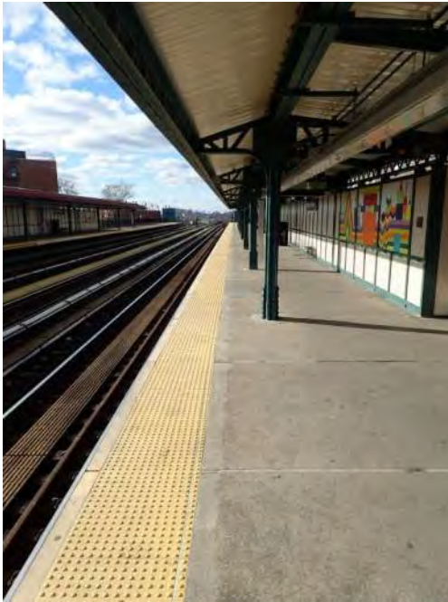
Figure 1 – General Station Condition Buhre Avenue Westchester Avenue Station
