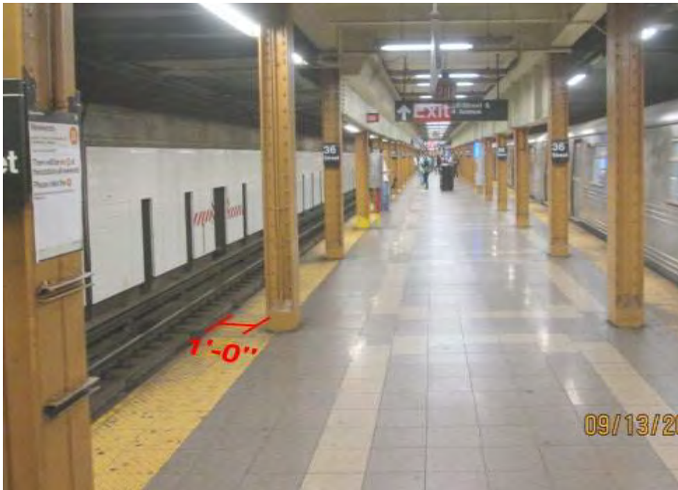
Figure 1 – Obstruction within 12” 36 th Street Station
