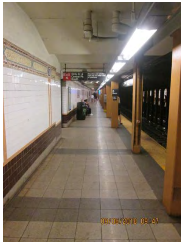
Figure 4 – Typical Platform View Fifth Avenue Station
