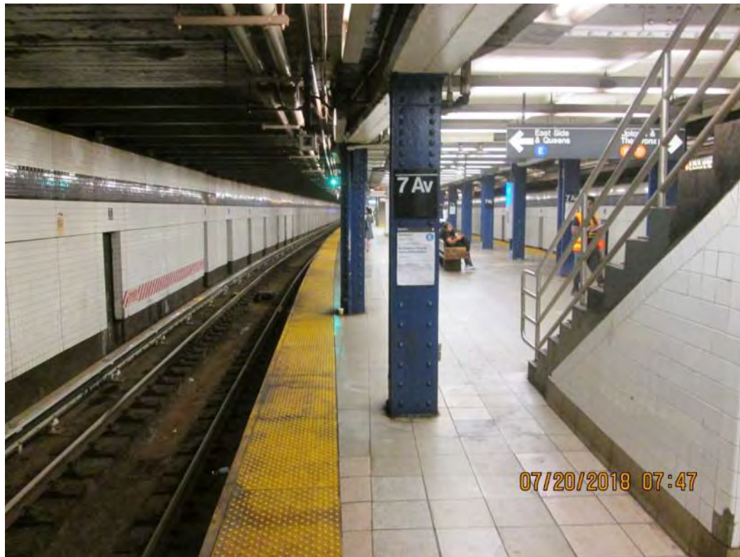
Figure 4 – Typical platform view 7 th Avenue Station
