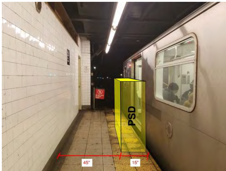
Figure 1 – Non-Compliant egress condition 34 th Street Station
