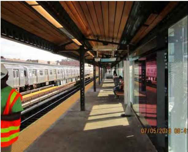
Figure 1 – Overall view 30 th Avenue Station
