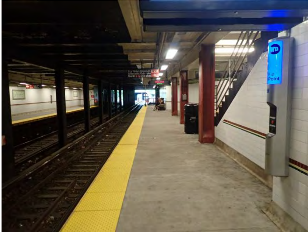
Figure 3 – General platform view Botanic Gardens Station
