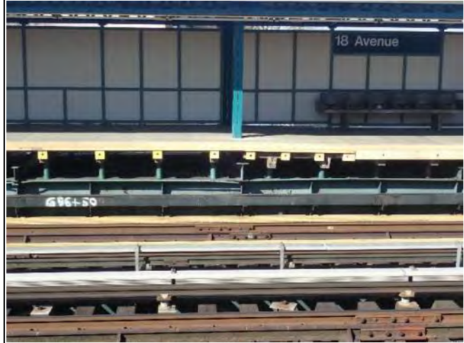
Figure 2 – Precast Slab 18 th Avenue Station
