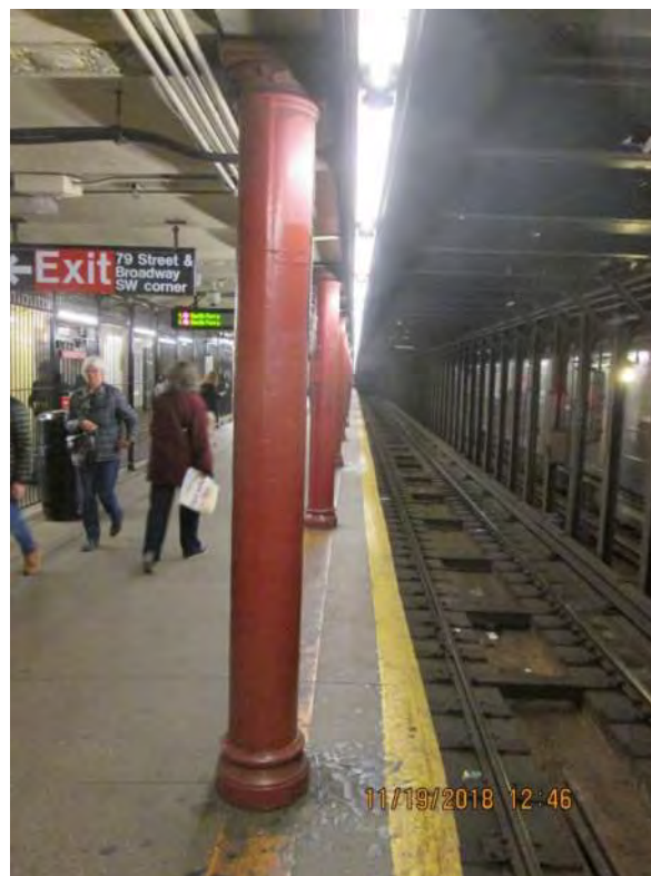
Figure 1 – Column 16” from the edge 79 th Street Station
