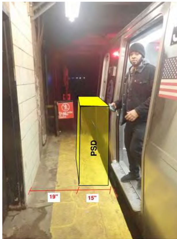
Figure 1 – Non-Compliant ADA condition 116 th Street Station
