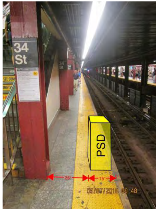
Figure 1 – Non-Compliant ADA condition 34 th Street Station
