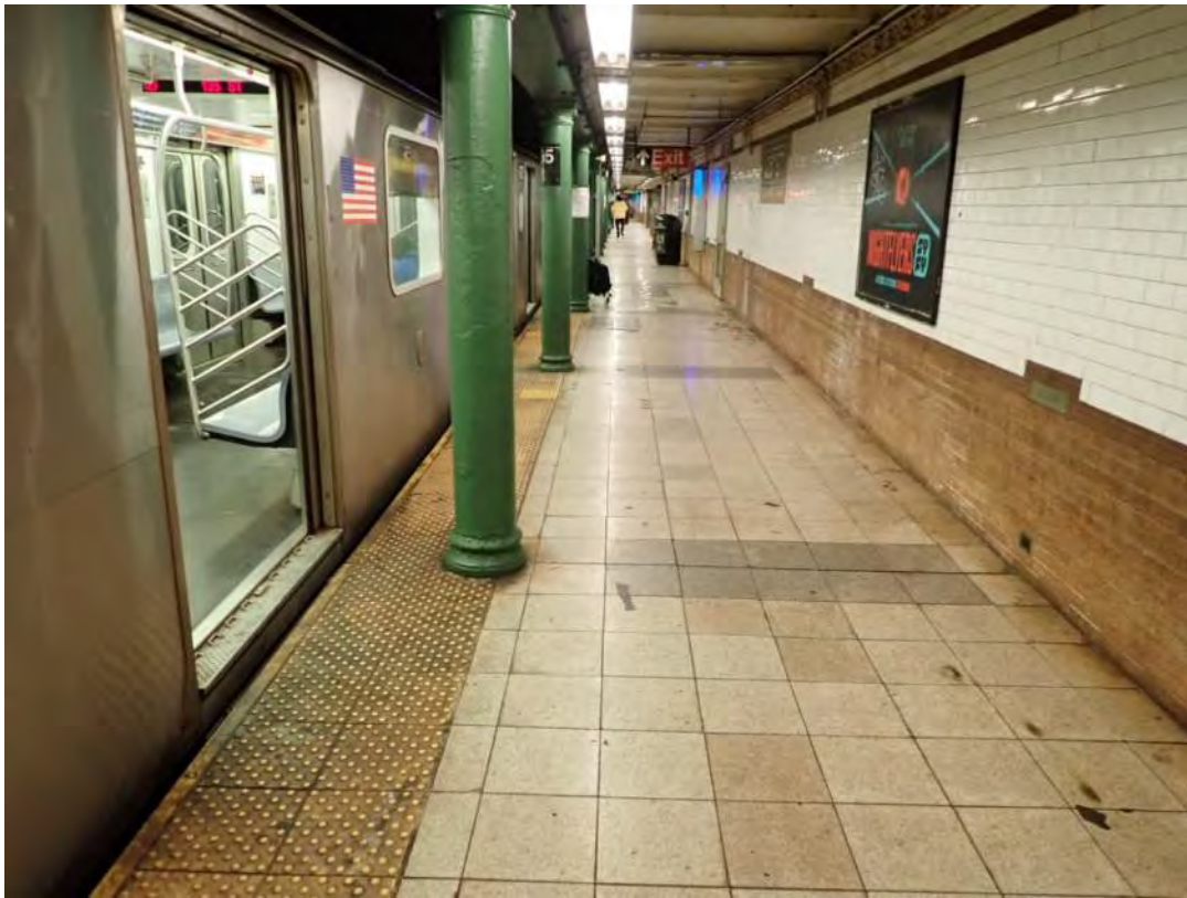
Figure 1 – Column 16” from the edge 135 th Street Station
