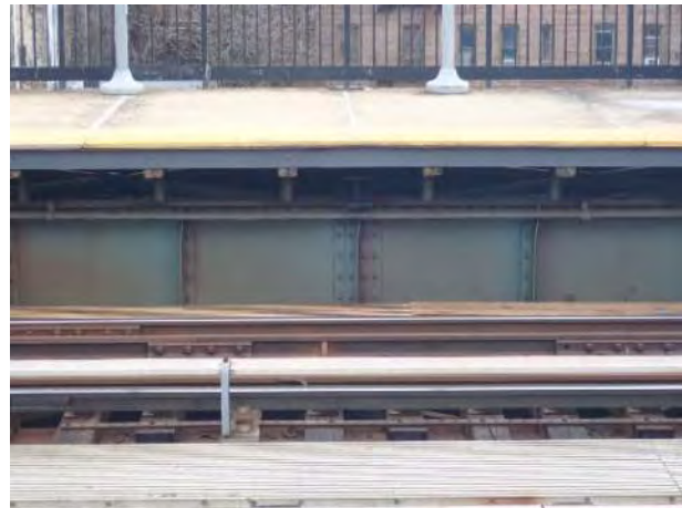
Figure 2 – Precast Slab Kingsbridge Road Station
