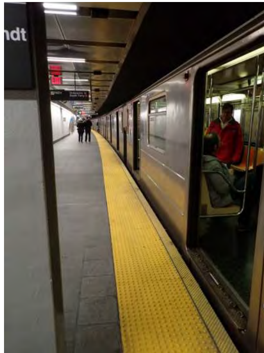
Figure 3 – Typical platform view Cortlandt Street Station
