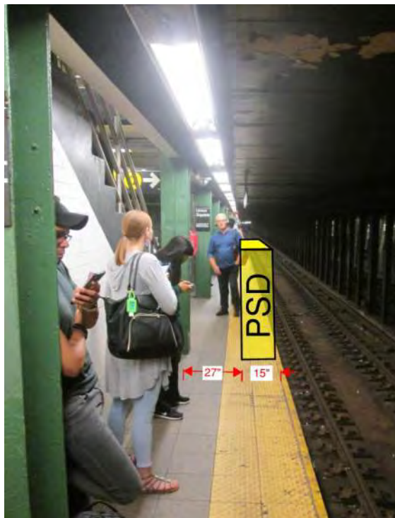
Figure 1 – Non-Compliant ADA condition 14th Street / Union Square
