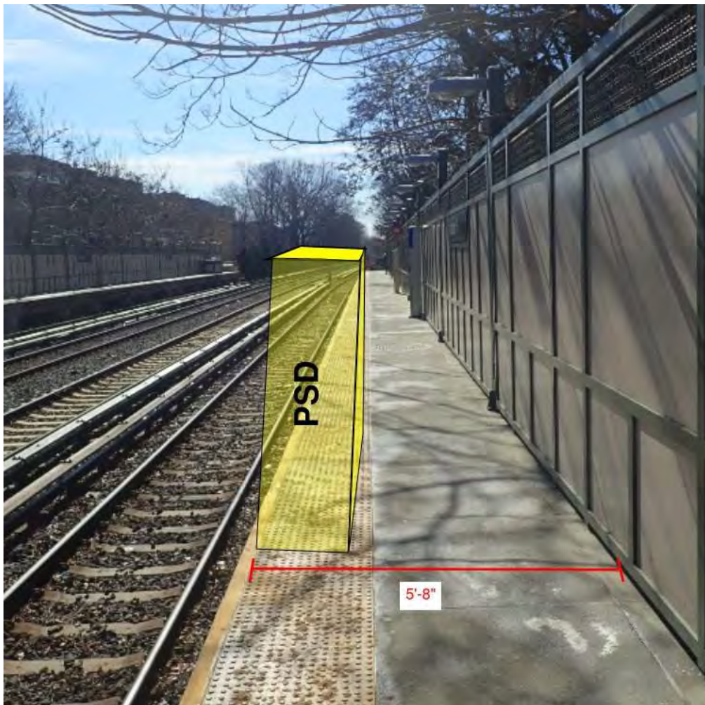
Figure 1 – Non-Compliant egress condition Avenue H Station
