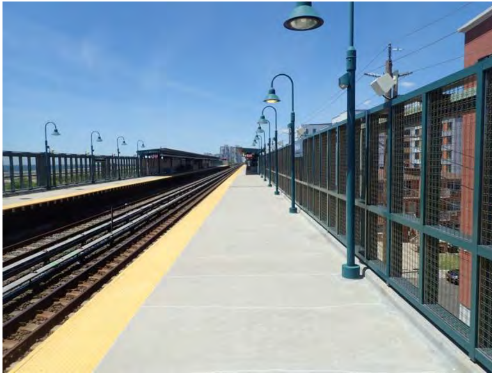
Figure 3 – General platform view Beach 44 th Street Station
