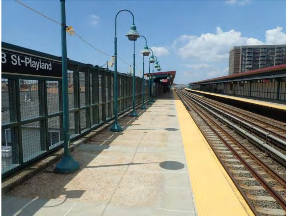
Figure 3 – General platform view Beach 98 th Street Station
