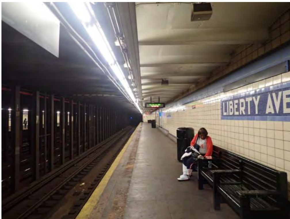
Figure 3 – General platform view Liberty Avenue Station
