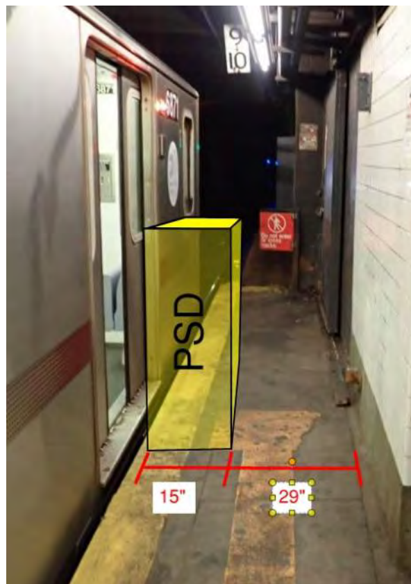
Figure 1 – Non-compliant ADA condition Winthrop Street Station
