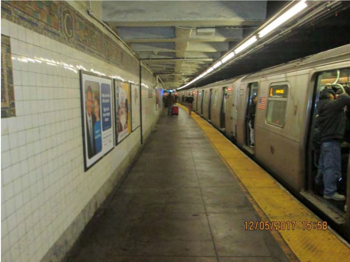
Figure 3 – Typical Platform Condition- Grand Avenue Station
