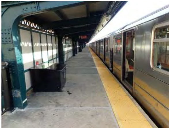
Figure 1 – General Station Condition Pennsylvania Avenue Station
