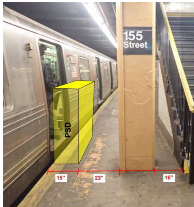
Figure 1 – Area of ADA non-compliance 155 th Street Station
