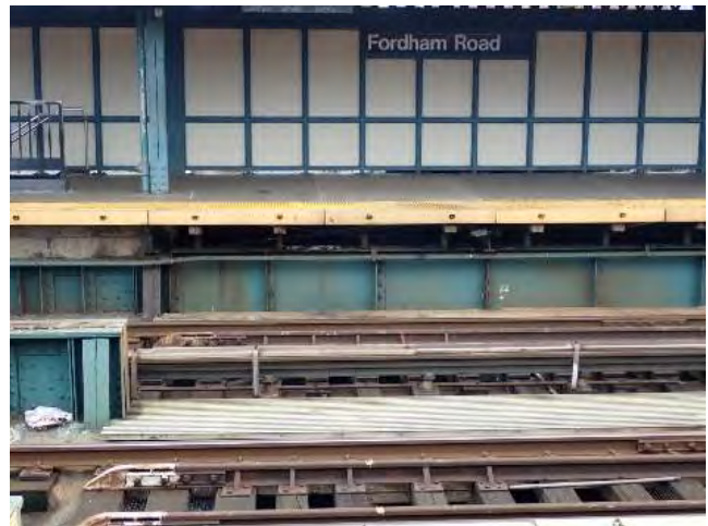
Figure 2 – Precast Slab Fordham Road Station
