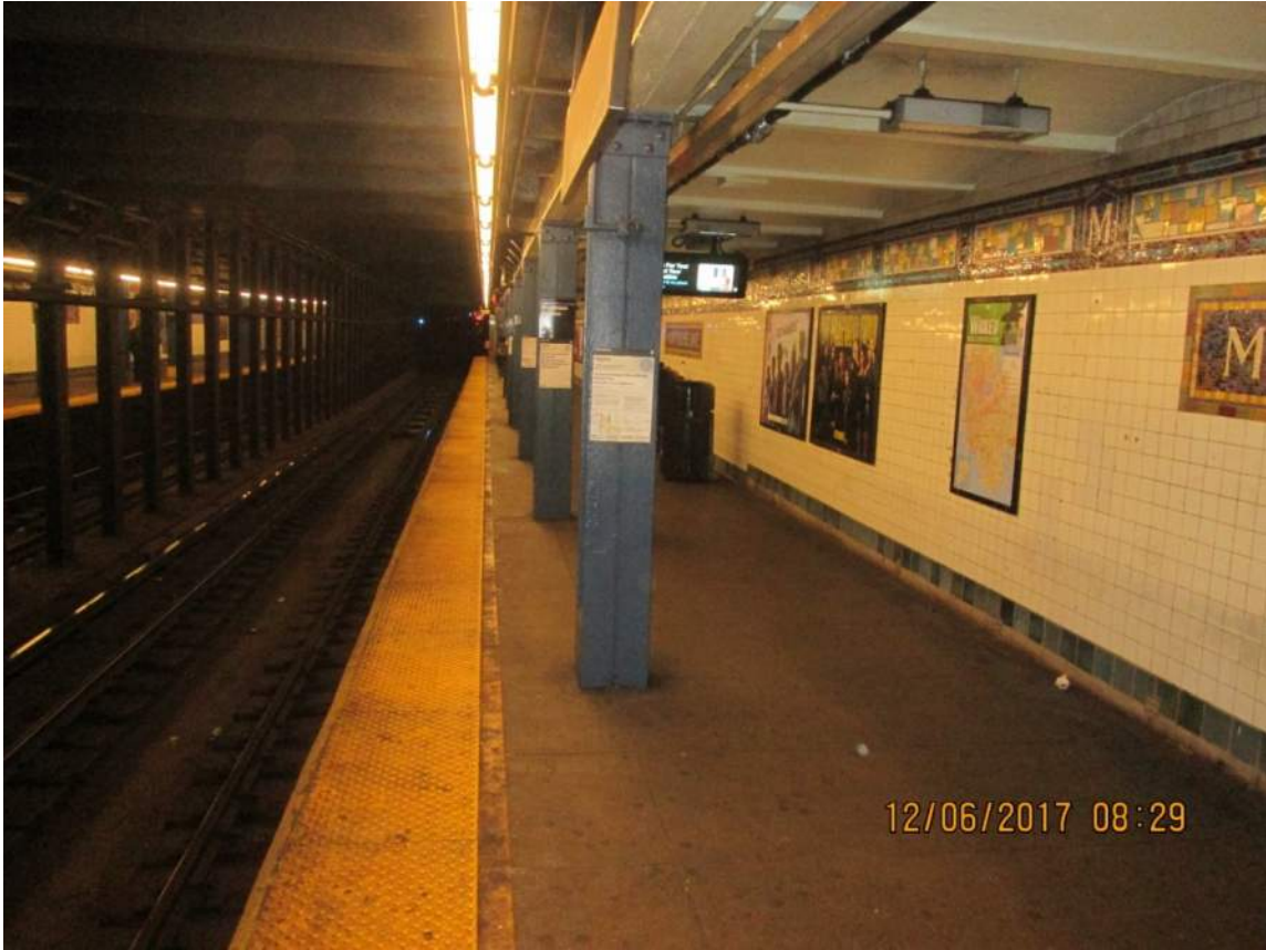
Figure 4 – Platform edge condition- Montrose Avenue Station
