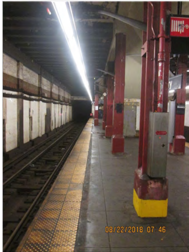
Figure 3 – Typical platform view Bowery Station
