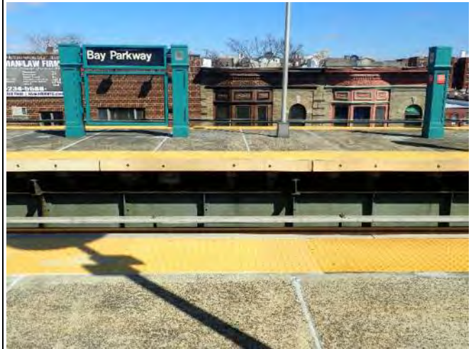
Figure 2 – Precast Slab Bay Parkway Station
