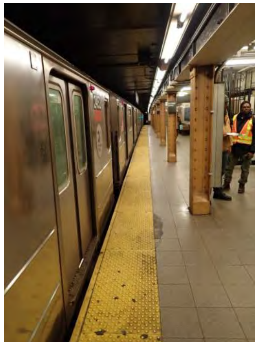
Figure 3 – Typical platform view Houston Street Station
