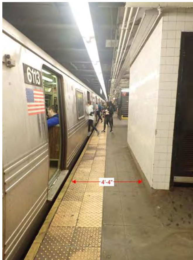
Figure 1 – Non-Compliant egress condition 168 th Street Station
