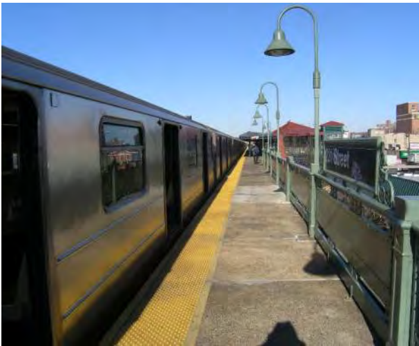
Figure 1 – Overall view 231 st Street Station
