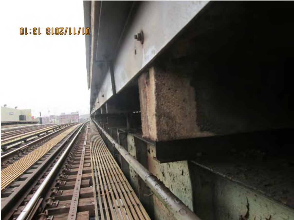
Figure 2 – Precast T-Beam platform – 52 nd Street-Lincoln Avenue Station
