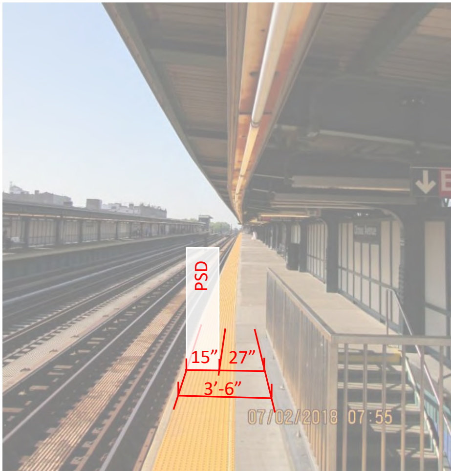
Figure 1– Non-compliant ADA Condition – Ditmas Avenue Station
