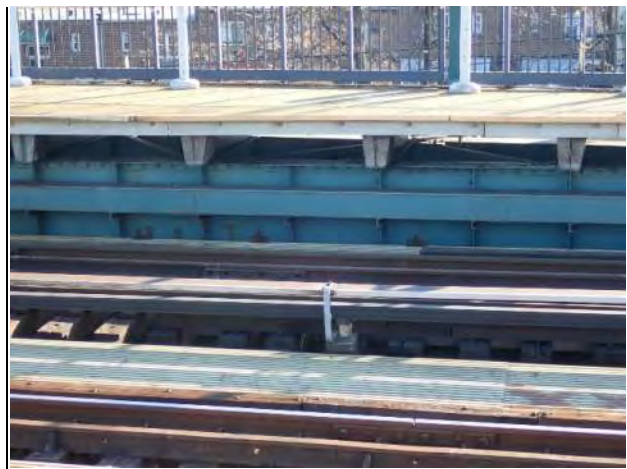
Figure 2 – Precast Slab Pelham Bay Parkway Station
