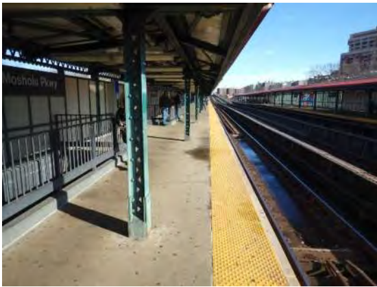
Figure 1 – General Station Condition Mosholu Parkway Station
