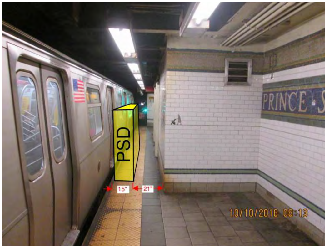
Figure 1 – Non-Compliant ADA condition Prince Street
