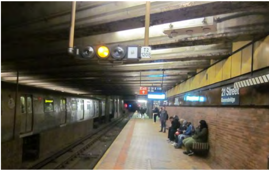
Figure 3 – Typical platform view with signal box- 21 st Street- Queensbridge Station
