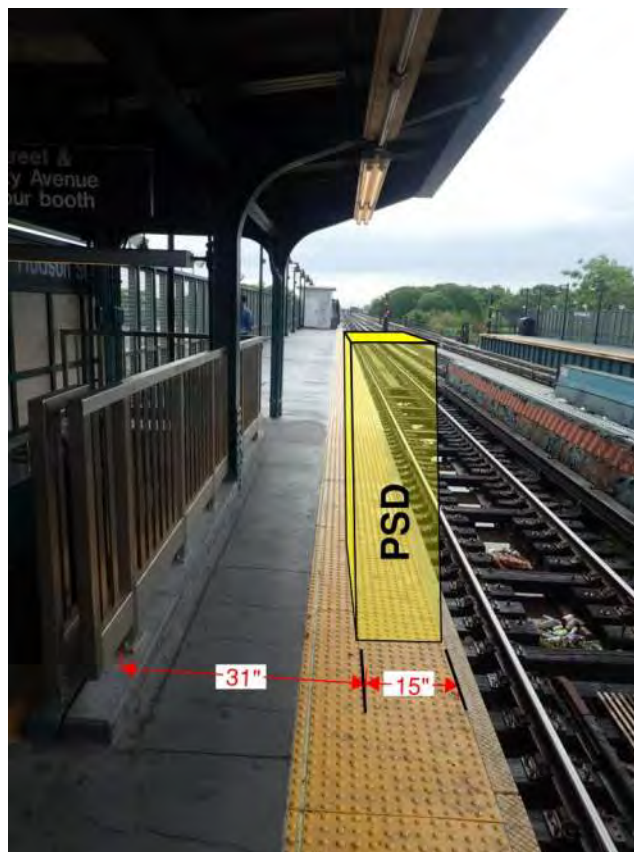
Figure 1 – Non-Compliant ADA condition 80 th Street
