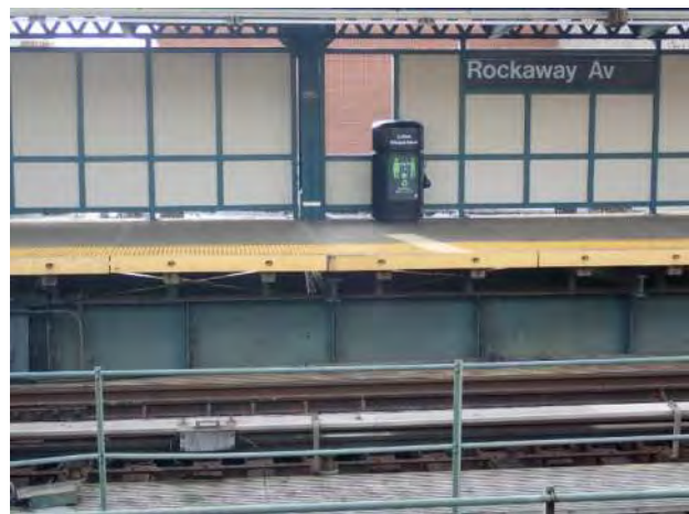
Figure 2 – Precast Slab Rockaway Avenue Station
