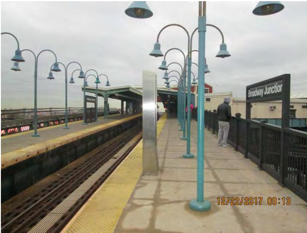
Figure 3 – Uncovered platform with canopy in the distance– Broadway Junction Station
