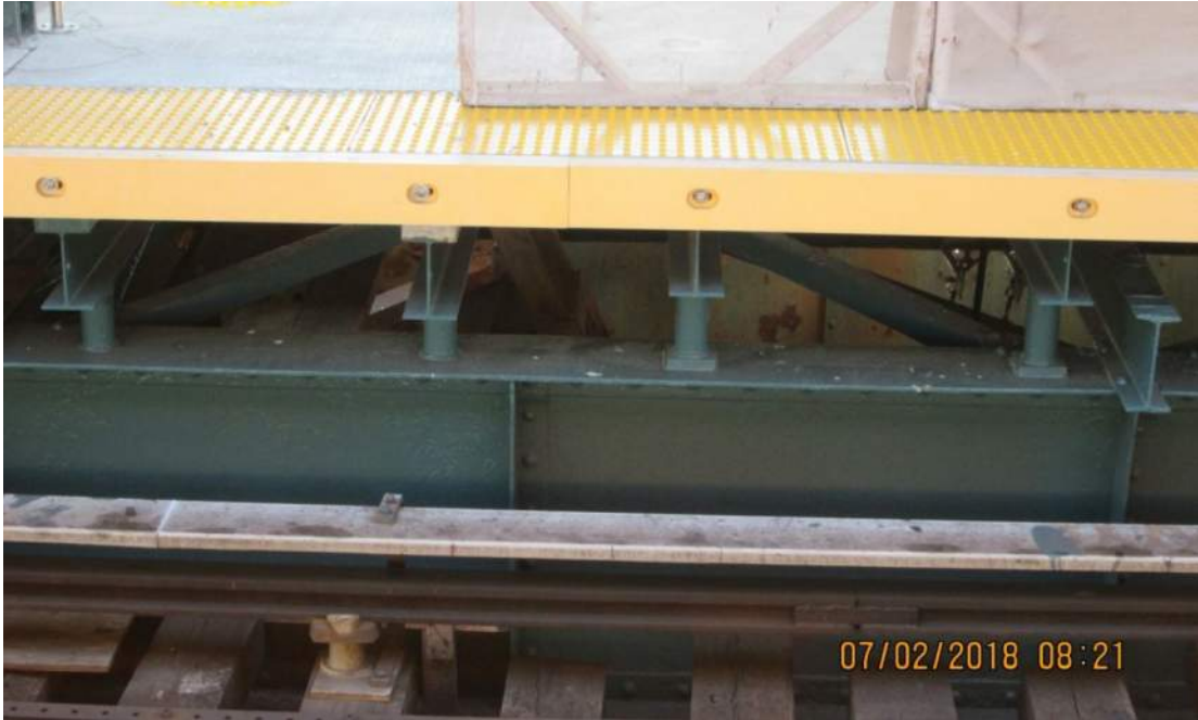
Figure 2– Precast T-Beam platform – 18 th Avenue Station
