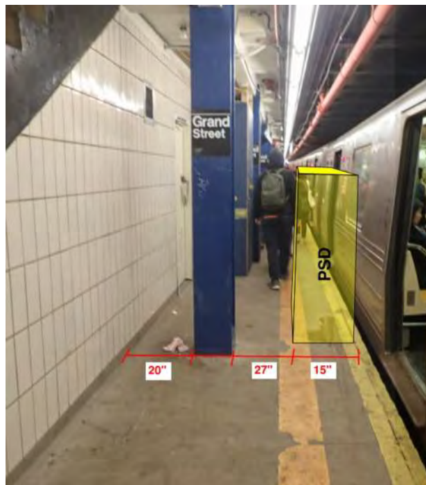
Figure 1 – Area of ADA non-compliance
