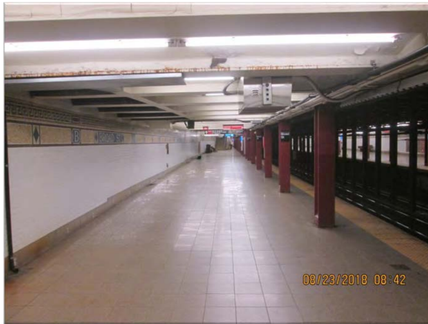
Figure 3 – Typical platform view Broad Street Station
