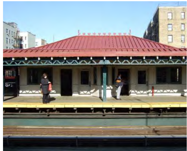
Figure 2 – Precast concrete platforms 231 st Street Station
