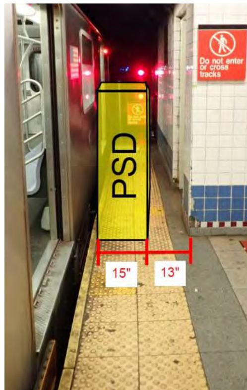
Figure 1 – Area of ADA non-compliance Flatbush Avenue Brooklyn College Station
