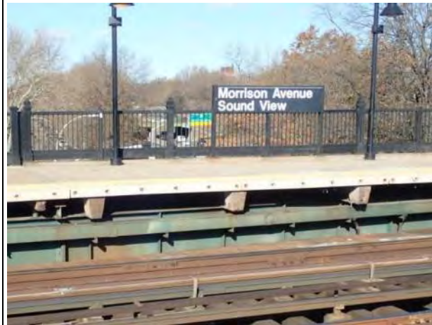
Figure 2 – Precast Slab Morrison Avenue – Soundview Station
