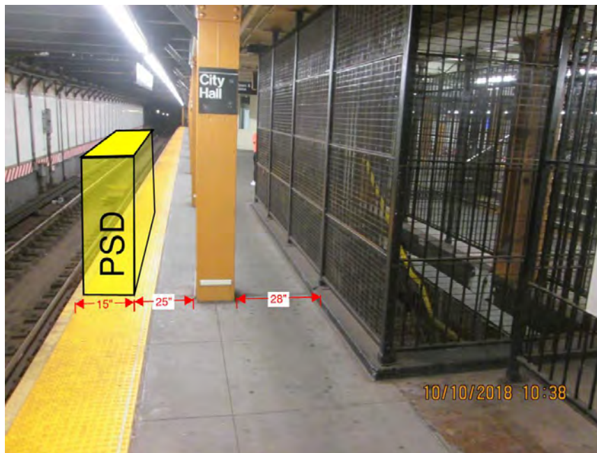
Figure 1 – Non-Compliant ADA condition City Hall Station
