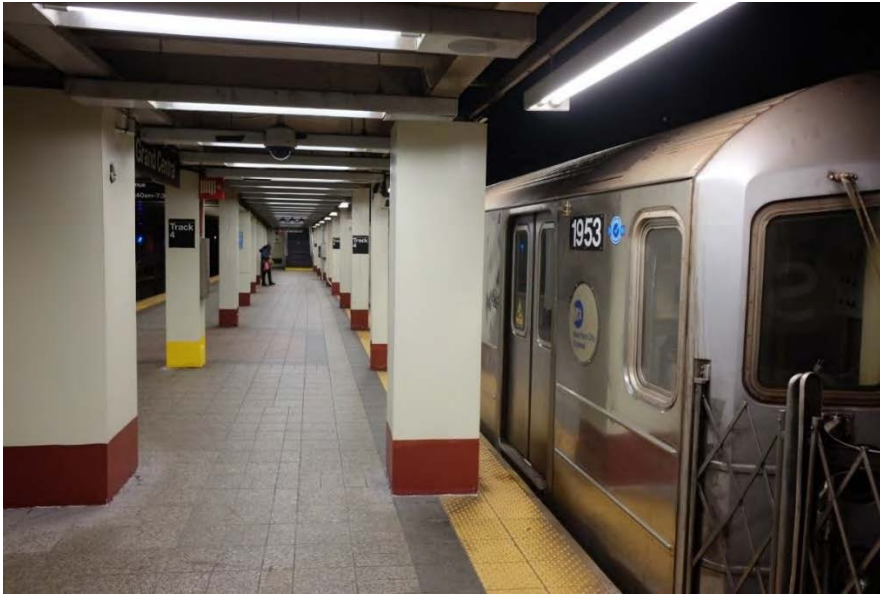
Figure 3 - Grand Central Station Shuttle – West end of north platform showing limited clearance for APGs or PSDs
