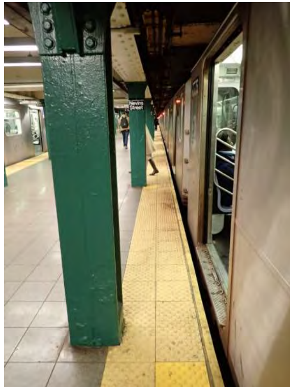
Figure 1 – Columns at 20” from platform edge Nevins Street Station
