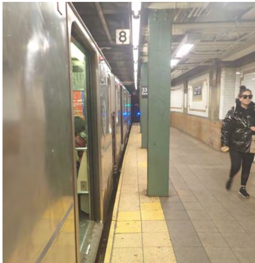
Figure 1 – Column 18” from the edge 33rd Street Station
