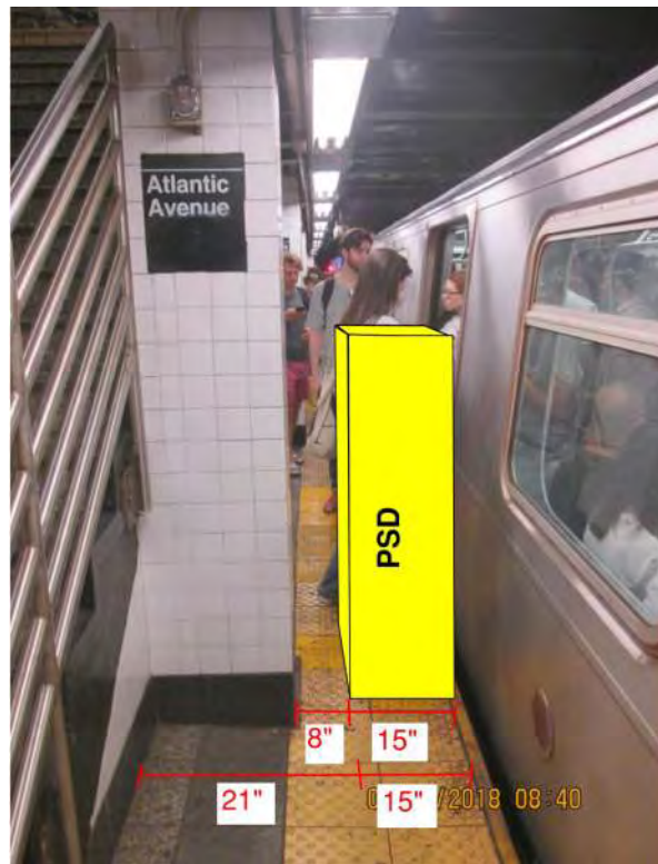
Figure 1 – Non-compliant ADA condition Atlantic Avenue Barclay Center Station
