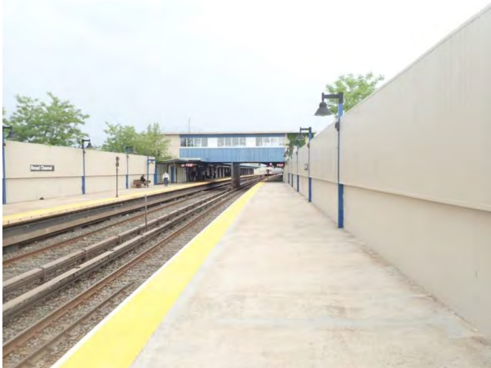
Figure 3 – General platform view Broad Channel Station
