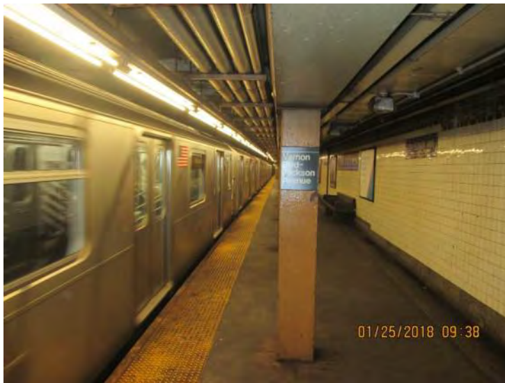
Figure 3 –Typical Platform Condition- Vernon Blvd.- Jackson Ave. Station
