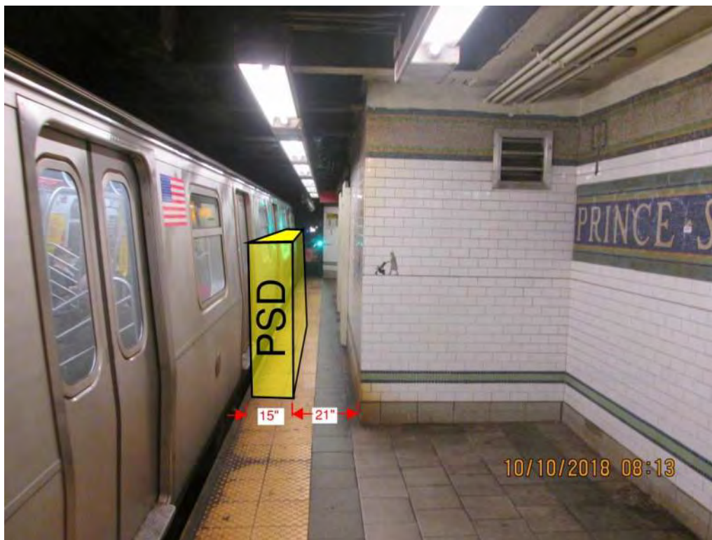
Figure 1 – Non-Compliant ADA condition Prince Street
