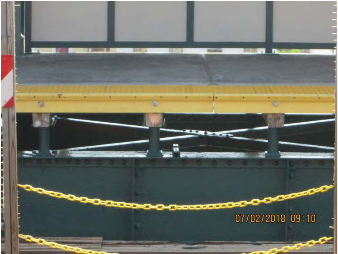
Figure 2– Precast T-Beam platform – Avenue N Station
