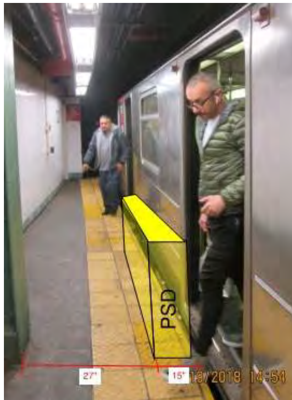
Figure 1 – Non-Compliant ADA condition 42nd Street Station
