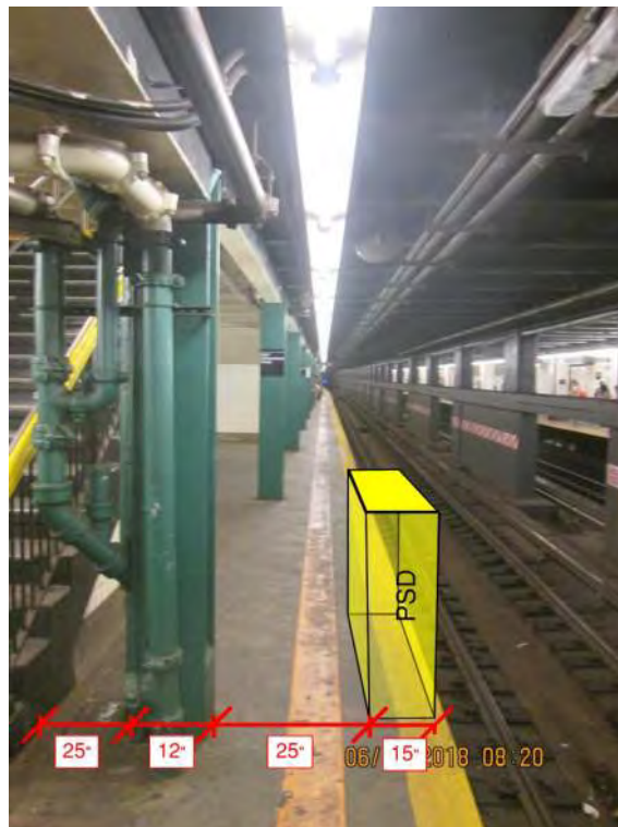
Figure 1: Non-Compliant ADA condition at stairs (typical on all platforms) MRN 175: Hoyt Schermerhorn Streets Station
