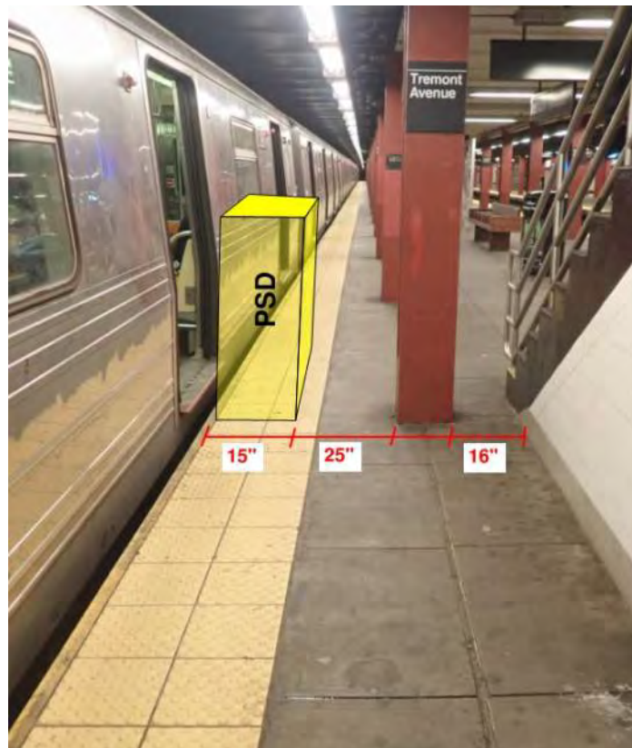
Figure 1 – Non-Compliant ADA condition Tremont Avenue
