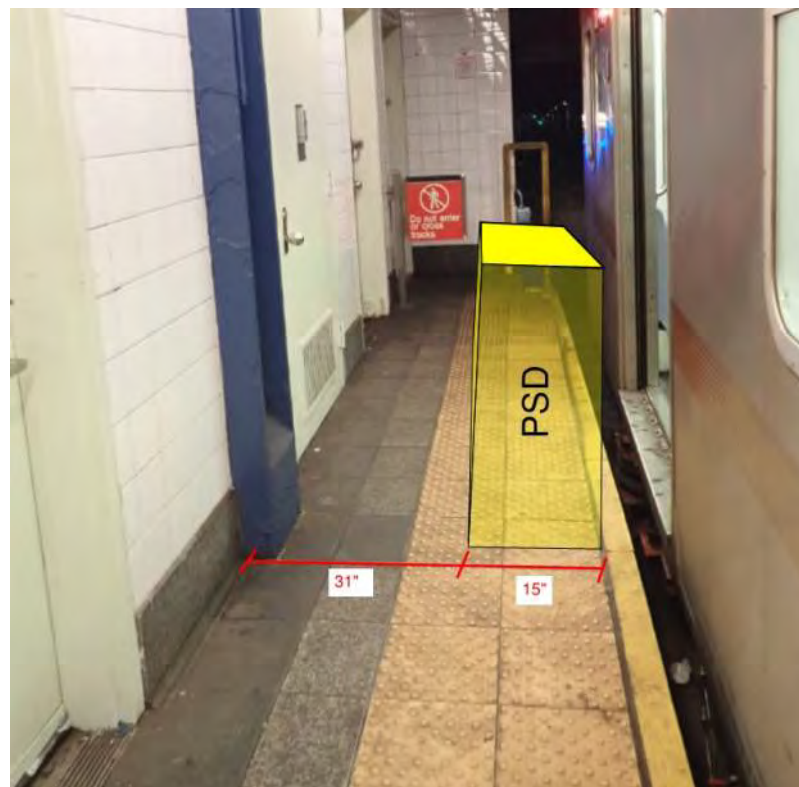
Figure 1 – Non-compliant ADA condition Fulton Street Station
