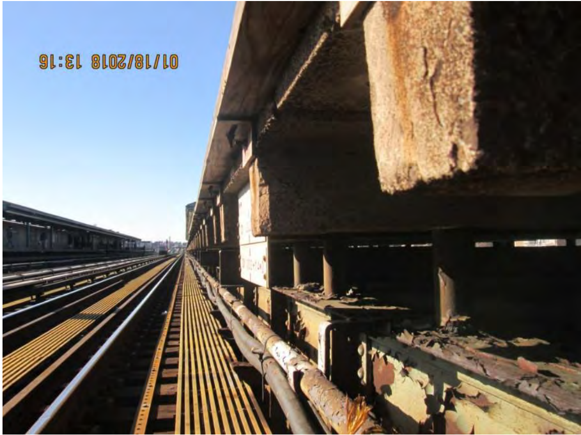
Figure 2 –Precast T-Beam Platform – 69 th Street-Fisk Avenue Station
