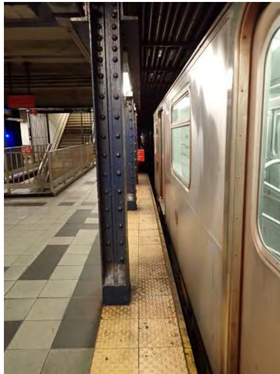
Figure 1 – Column 12” from the edge Crown Heights Utica Avenue
