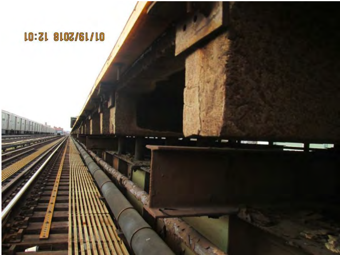
Figure 2 – Precast T-Beam platform – 82nd Street-Jackson Heights Station
