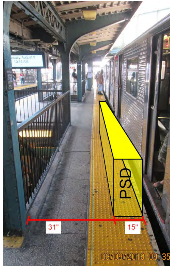
Figure 1 – Non-Compliant ADA condition Myrtle Avenue-Broadway Station
