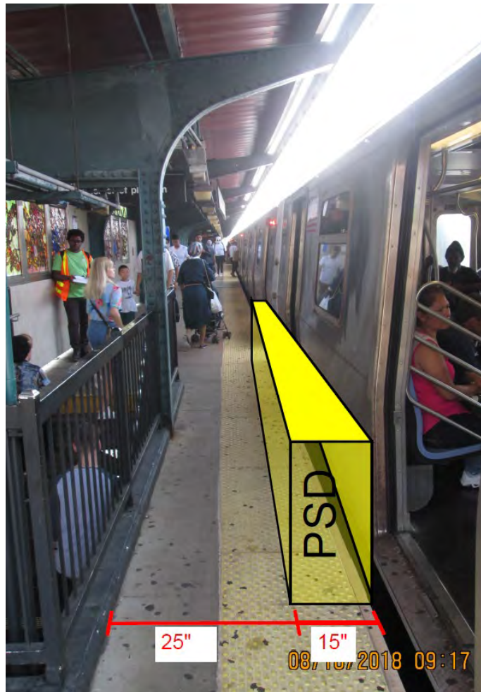
Figure 1 – Non-Compliant ADA condition Lorimer Street Station
