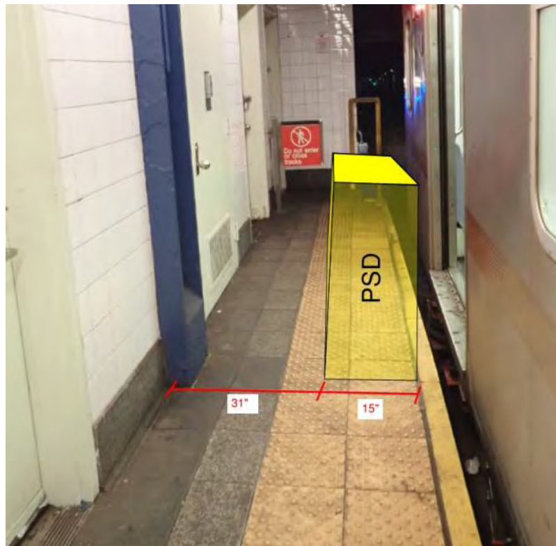
Figure 1 – Non-compliant ADA condition Fulton Street Station
