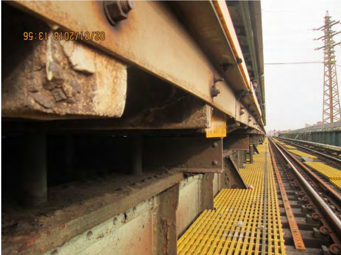
Figure 2– Precast T-Beam Platform – 61 st Street-Woodside Avenue Station
