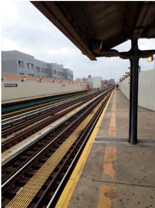
Figure 1 – General Station Condition Intervale Avenue Station
