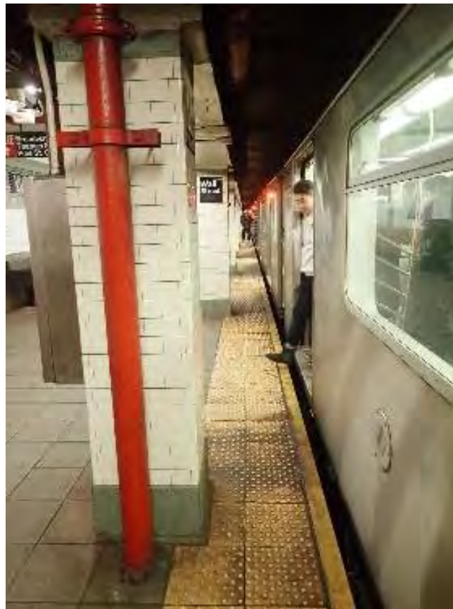
Figure 1 – Column 20” from the edge Wall Street Station
