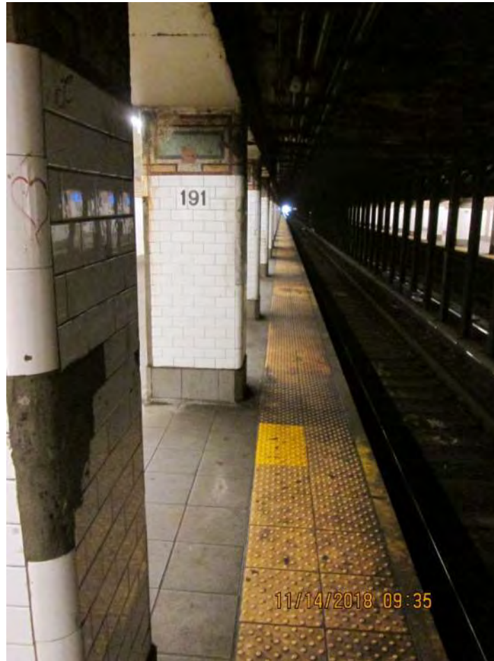
Figure 3 – Typical Platform View 191 st Street Station
