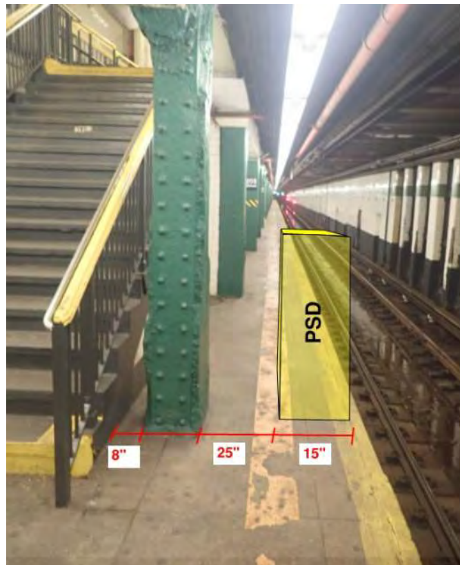
Figure 1 – Non-Compliant ADA condition 205 th Street Norwood
