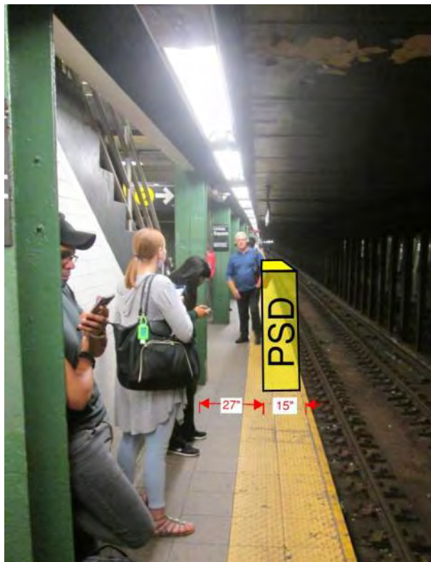
Figure 1 – Non-Compliant ADA condition 14th Street / Union Square
