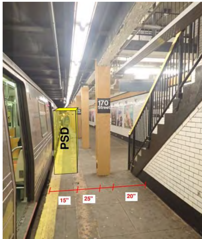
Figure 1 – Non-Compliant ADA condition 170 th Street
