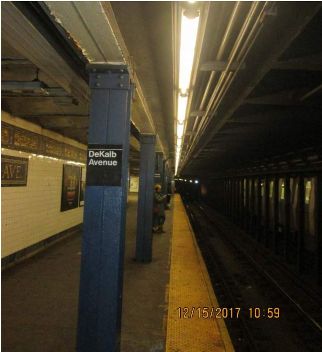
Figure 3– Typical Platform Edge Condition- DeKalb Avenue Station
