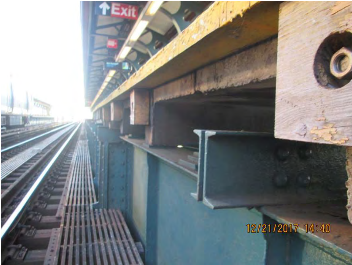
Figure 2 – Precast T-Beam platform – Junction Boulevard Station
