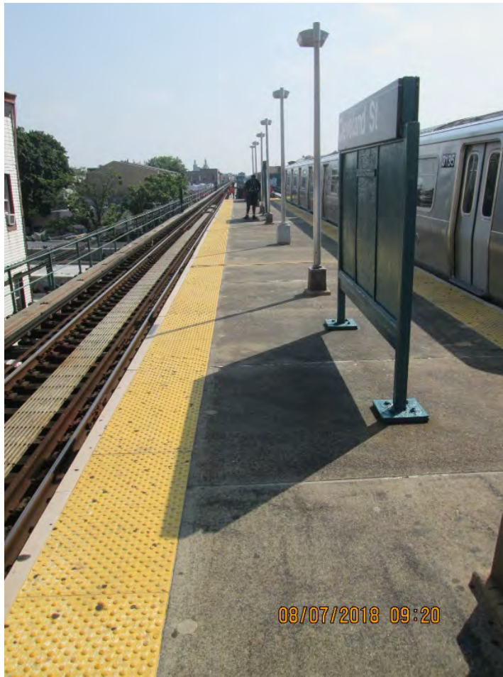
Figure 1 – Precast platform Cleveland Street Station
