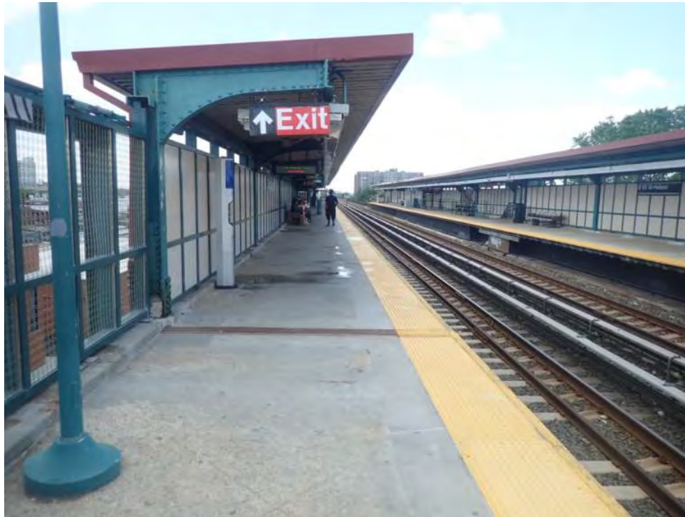
Figure 3 – General platform view Beach 90 th Street Station
