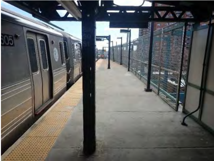
Figure 1 – General Station Condition Bay 50 th Street Station
