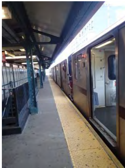
Figure 1 – General Station Condition Kingsbridge Road Station
