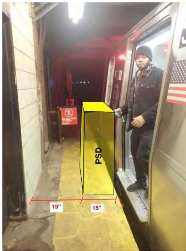
Figure 1 – Non-Compliant ADA condition 116 th Street Station
