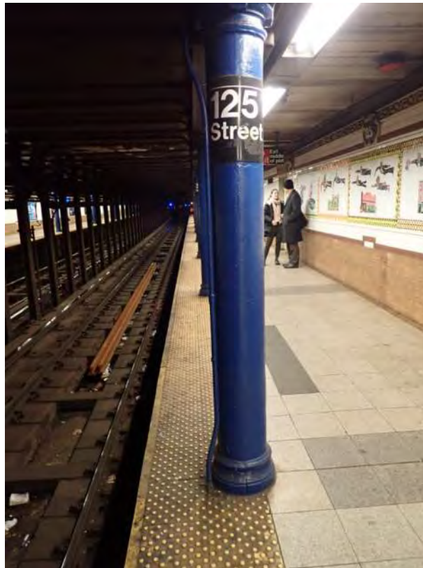
Figure 1 – Column 16” from the edge 125 th Street Station
