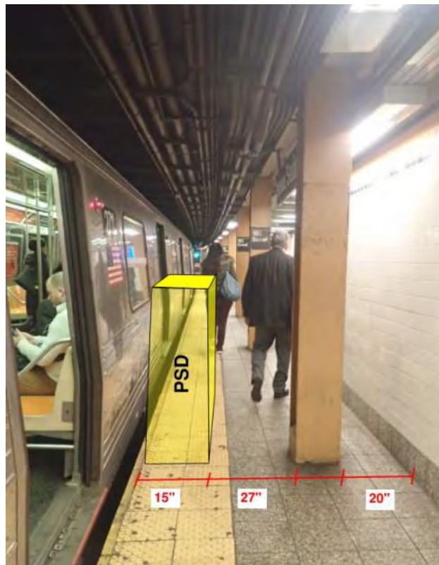
Figure 1 – Non-Compliant ADA condition 161 st Street Yankee Stadium Street
