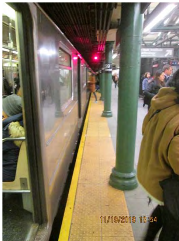
Figure 1 – Column 18” from the edge 59 th Street Station
