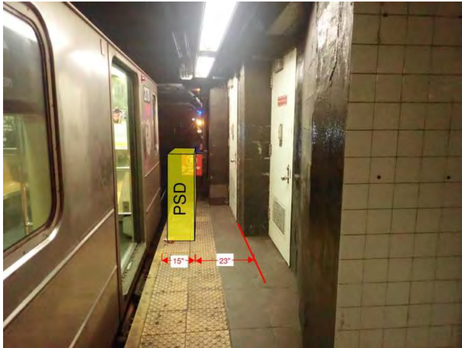
Figure 3– Non-compliant ADA zone at north end of northbound platform
