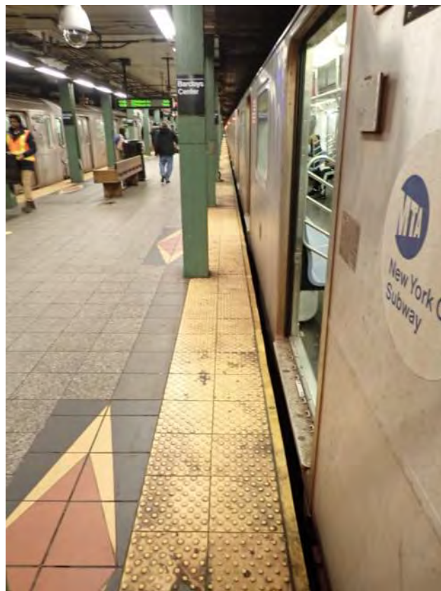
Figure 1 – Column 16” from the edge Atlantic Avenue Barclay Ctr. Station
