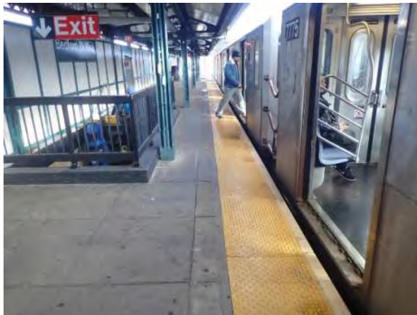
Figure 1 – General Station Condition Bedford Park Boulevard Station
