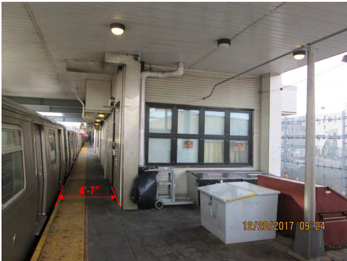
Figure 1 –Effective platform width at Track 2 side, looking south- Rockaway Parkway Station
