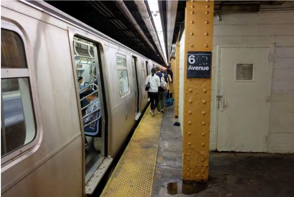
Figure 13 - Constrained space at 8th Ave-bound platform – 6 th Avenue Station
