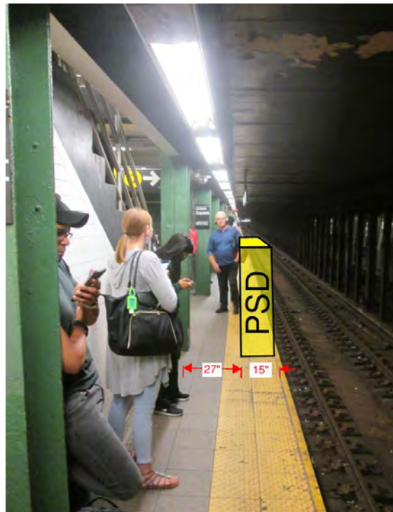
Figure 1 – Non-Compliant ADA condition 14 th Street / Union Square
