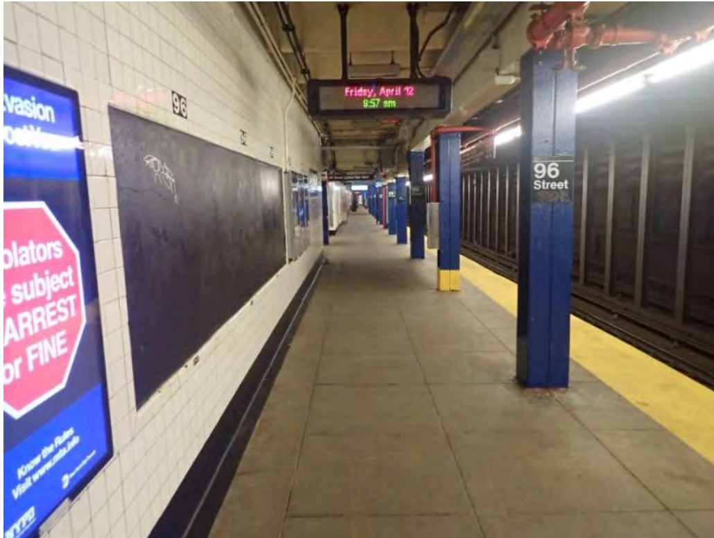
Figure 3 – General platform view 96th Street Station
