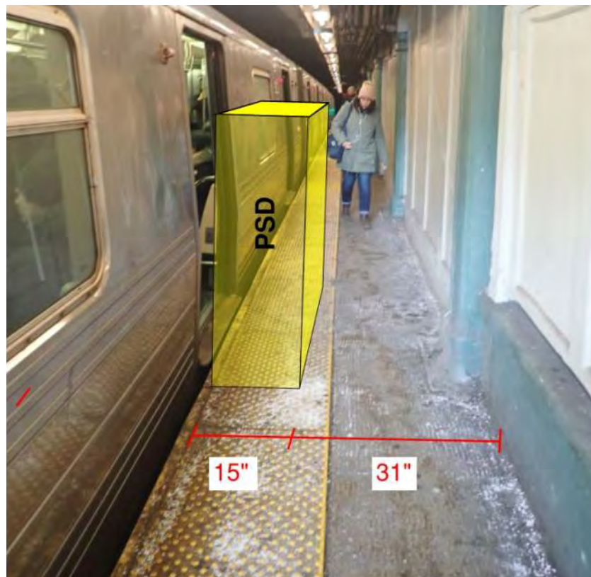
Figure 1 – Non-compliant ADA condition Prospect Park Station
