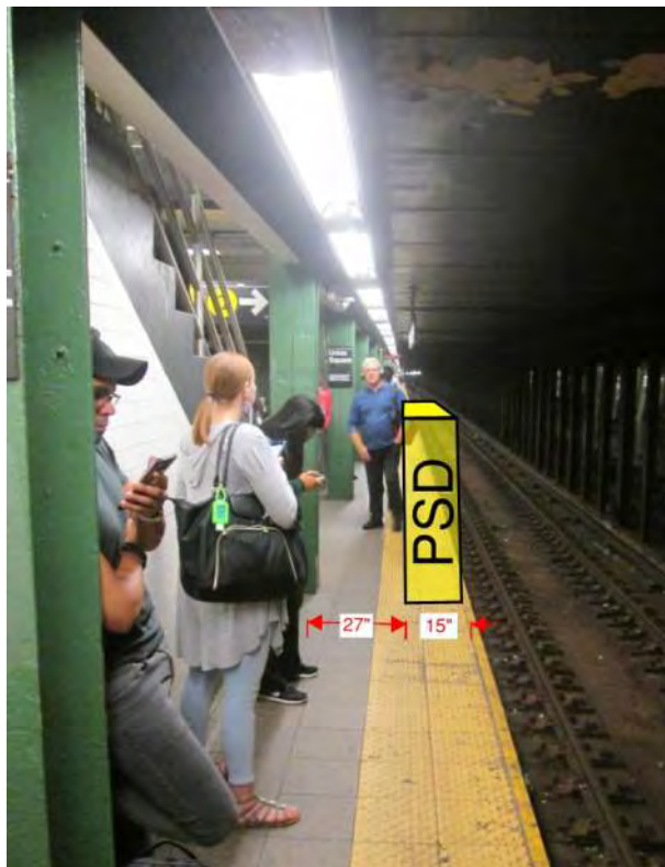
Figure 1 – Non-Compliant ADA condition 14 th Street / Union Square
