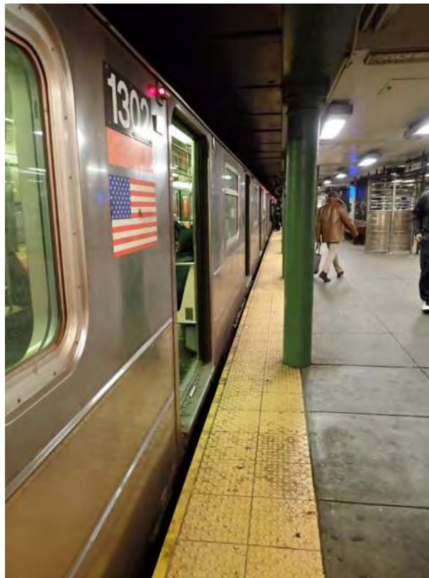
Figure 1 – Column 16” from the edge 116 th Street Station
