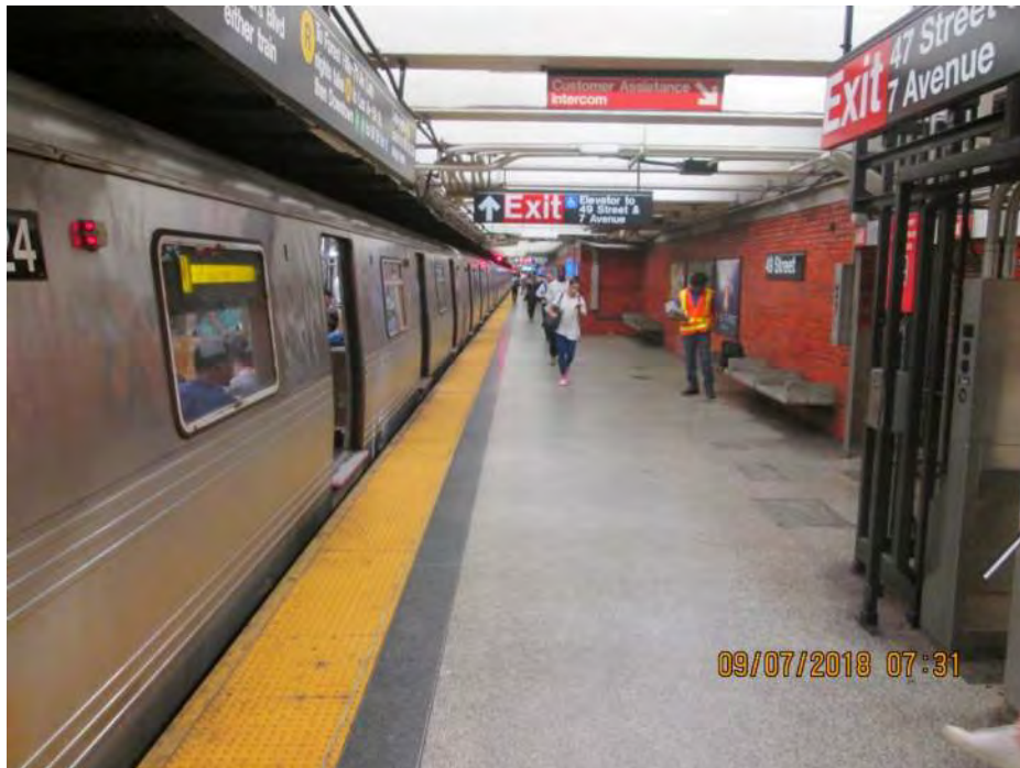
Figure 3 – General platform view 49th Street Station
