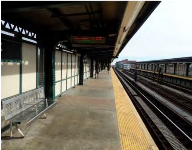
Figure 1 – General Station Condition Junius Street Station
