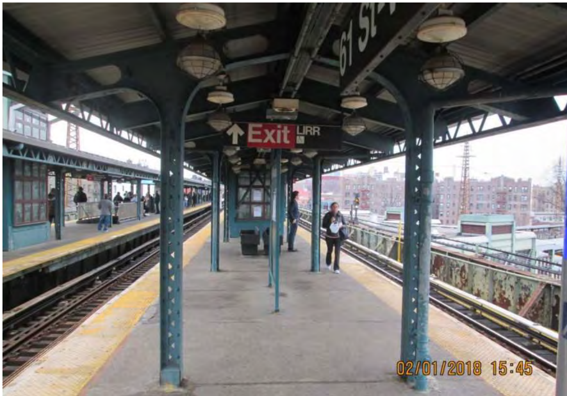
Figure 1– Typical Platform Condition – 61 st Street-Woodside Avenue Station
