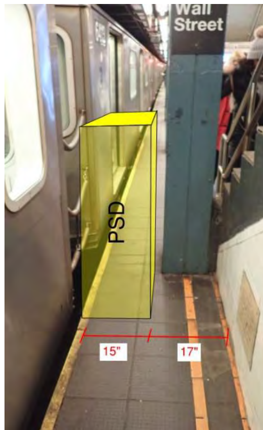
Figure 1 – Non-compliant ADA condition Wall Street Station
