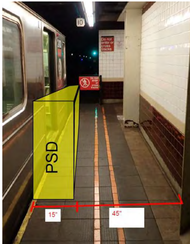
Figure 1 – Non-Compliant code condition 18 th Street Station
