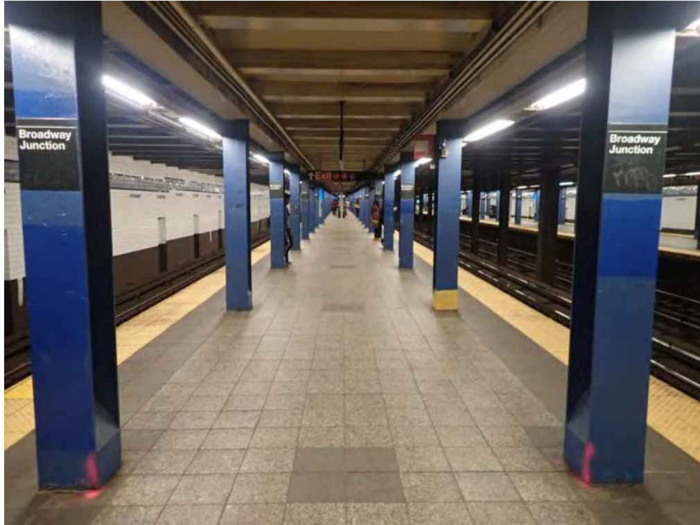
Figure 3 – Typical platform view Broadway Junction Station
