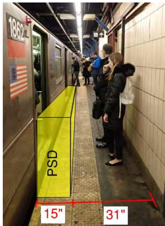
Figure 1 – Non-compliant ADA condition Chambers Street Station
