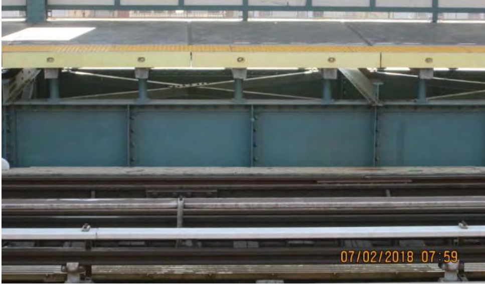
Figure 2– Precast T-Beam platform – Ditmas Avenue Station
