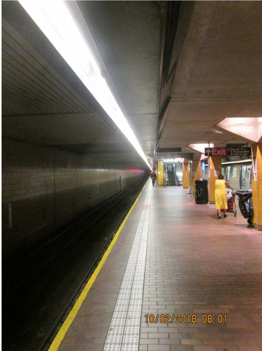
Figure 3 – Typical platform view Jamaica Center– Parsons Archer Station
