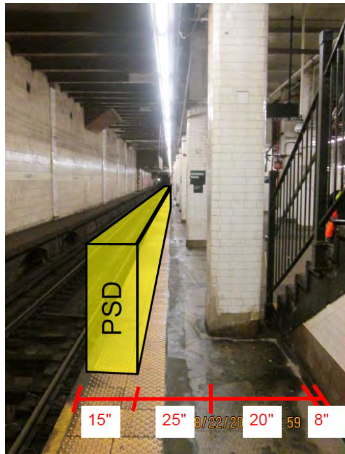
Figure 1 – Non-Compliant ADA condition Chambers Street Station
