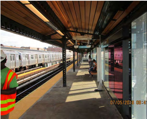
Figure 1 – Overall view 30 th Avenue Station
