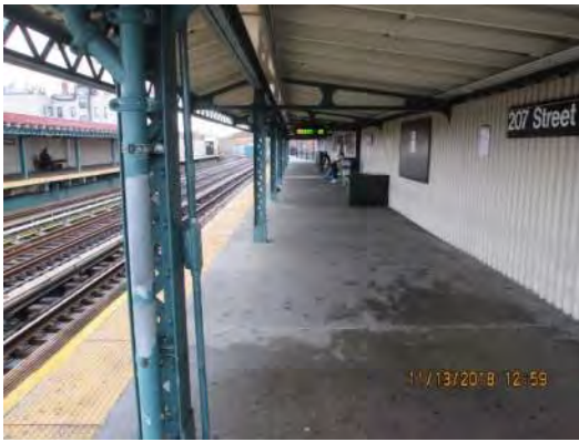
Figure 1 – Overall view 207 th Street Station
