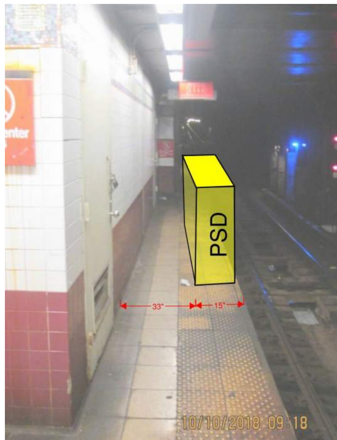
Figure 1 – Non-Compliant ADA condition Canal Street Station
