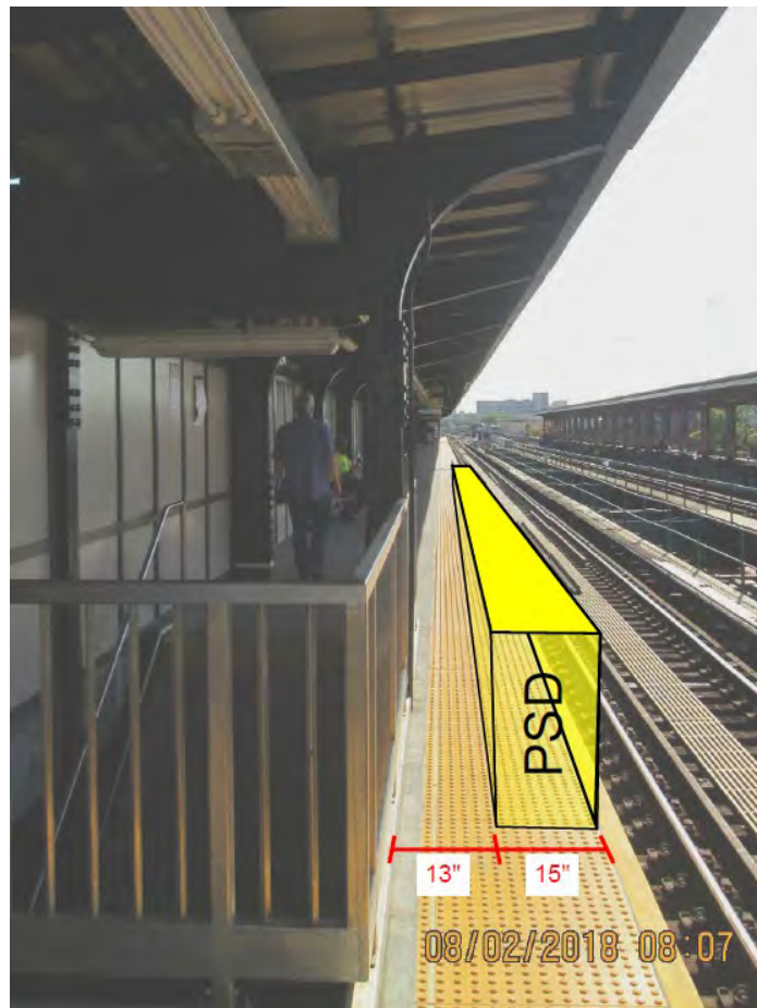
Figure 1 – Non-Compliant ADA condition 121 st Street Station
