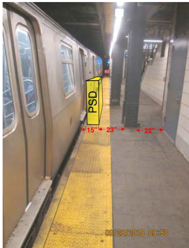
Figure 1 – Non-Compliant ADA condition 53 rd Street Station
