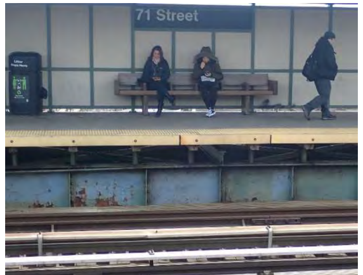
Figure 2 – Precast Slab 71 st Street Station
