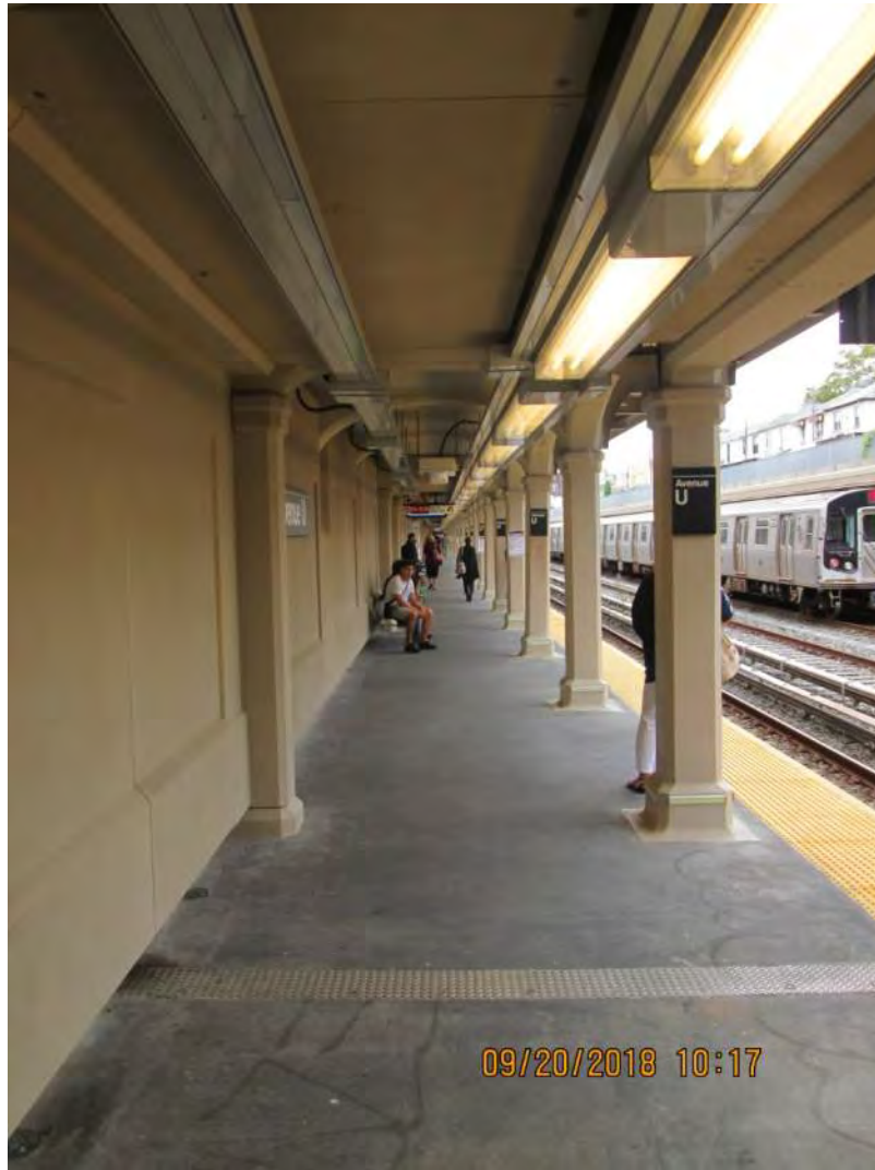
Figure 3 – Typical platform view Avenue U Station
