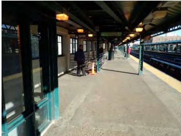
Figure 1 – General Station Condition 161 st Street Station
