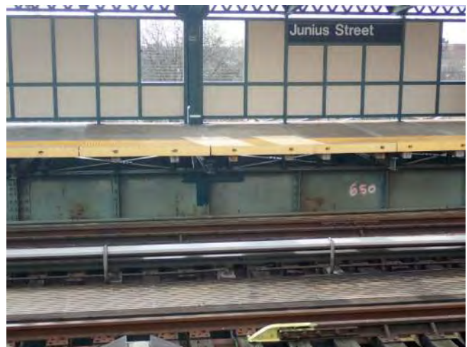
Figure 2 – Precast Slab Junius Street Station
