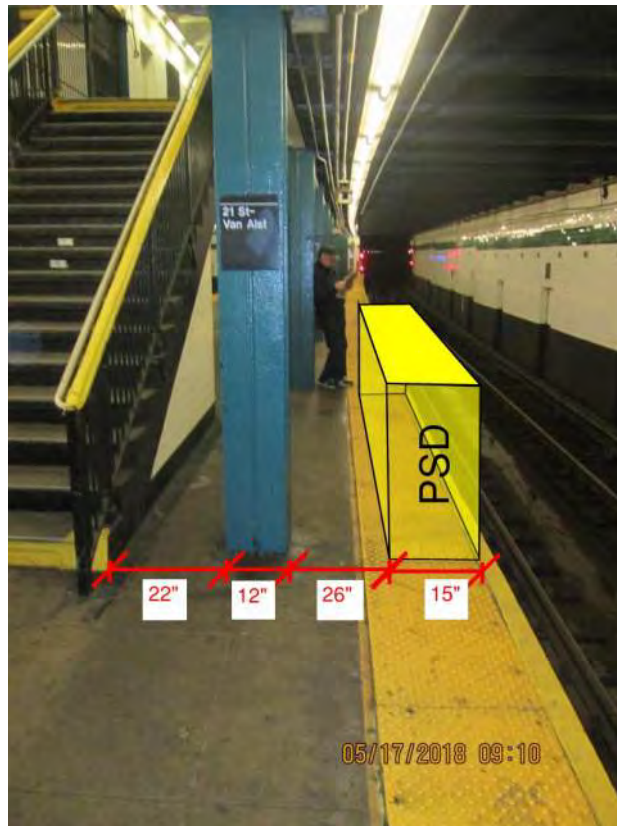
Figure 1 – Non-Compliant ADA condition at staircase P5 MRN 282: 21 st Street Van Alst Jackson A
