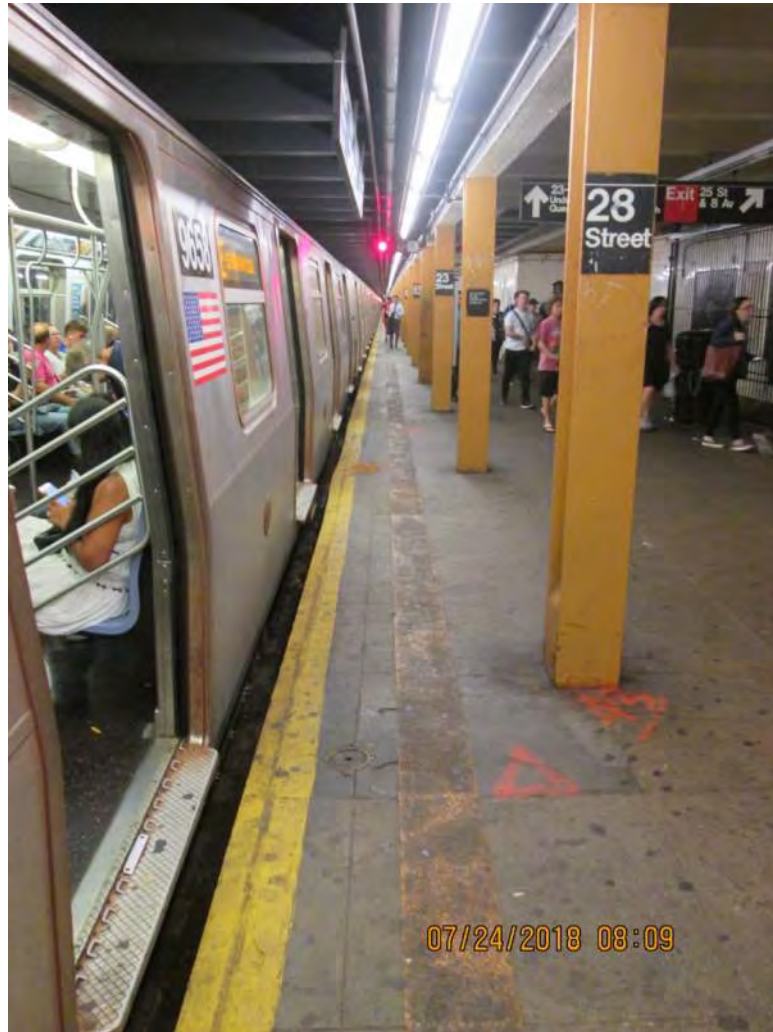
Figure 3 – Typical platform view with signal light 23 rd Street Station
