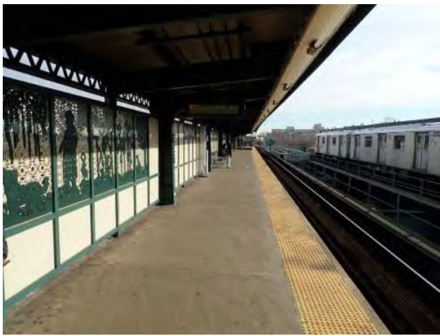
Figure 1 – General Station Condition Van Siclen Avenue Station
