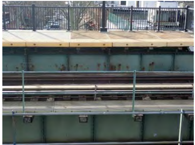
Figure 2 – Precast Slab Van Siclen Avenue Station
