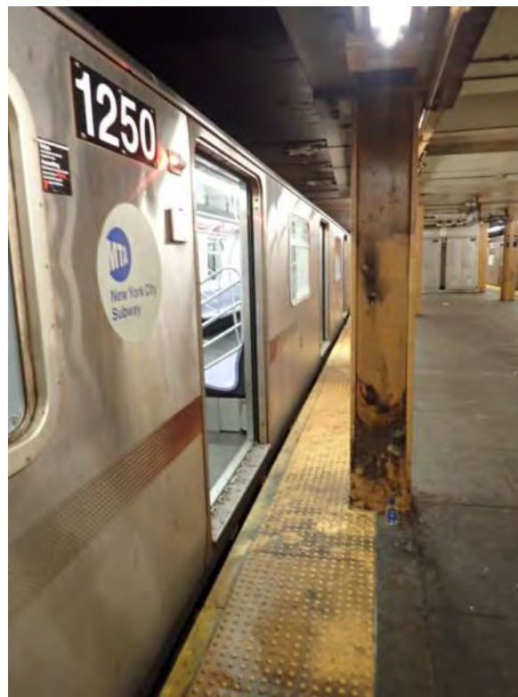
Figure 1 – Column 16” from the edge Franklin Avenue Station
