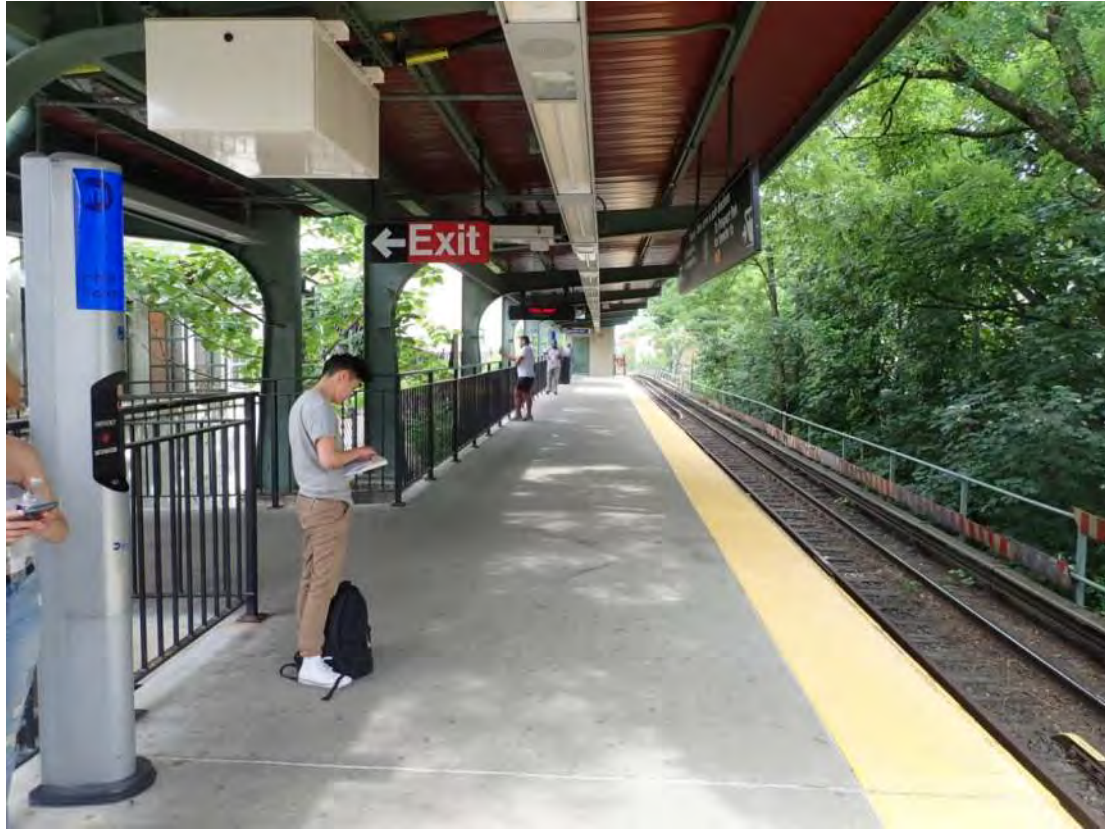
Figure 3 – General platform view Park Place Station
