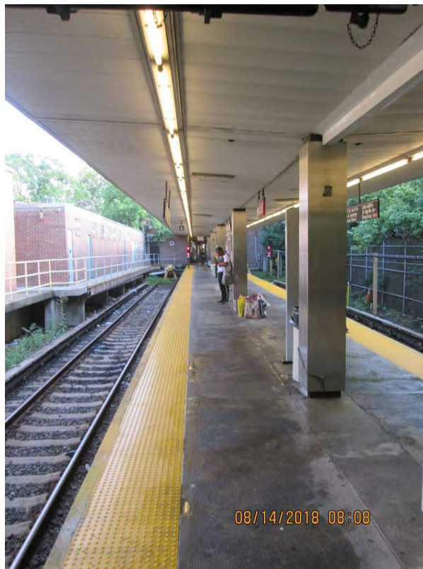
Figure 3 – Typical platform view Middle Village Metropolitan Avenue Station
