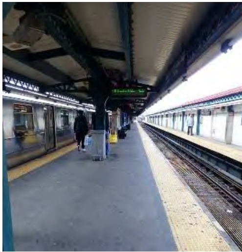
Figure 1 – General Station Condition Pelham Bay Parkway Station
