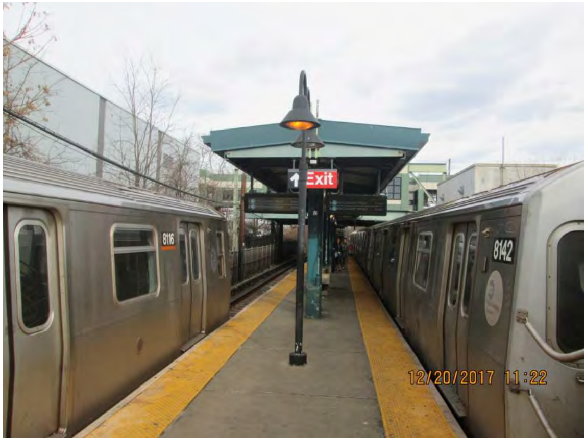
Figure 1– General Platform Condition – East 105th Station
