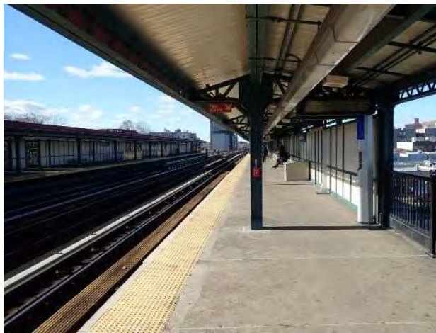
Figure 1 – General Station Condition Castle Avenue Station
