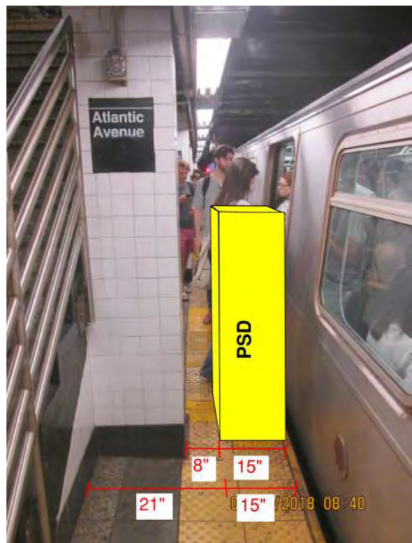
Figure 1 – Non-compliant ADA condition Atlantic Avenue Barclay Center Station
