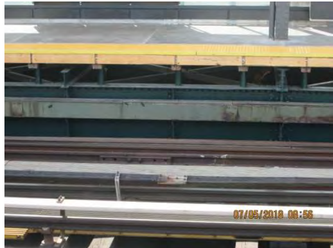
Figure 2 – Precast concrete platforms 36 th Avenue Station
