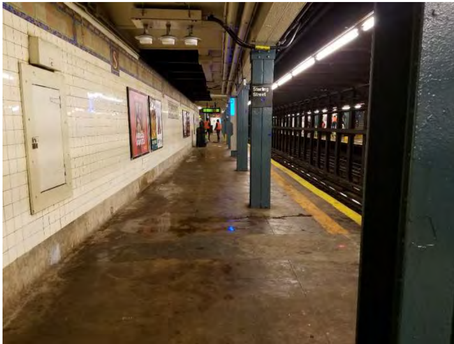
Figure 3 – Typical platform view Sterling Street Station
