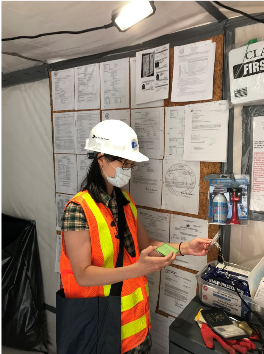
System Safety Specialist Kari Ng inspects the project postings (required paperwork) in the Clean Room of the Personal Decontamination Enclosure System on an asbestos abatement project at East New York Bus Depot.
