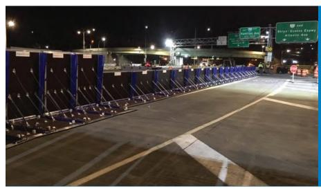
FIGURE 14: RAISED SEAWALL AT GOVERNORS ISLAND VENTILATION BUILDING
