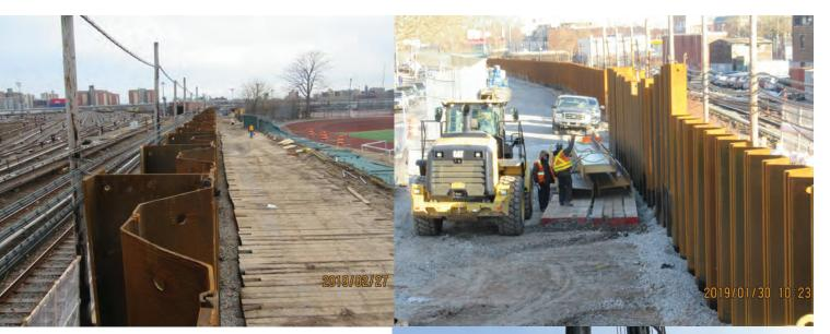
FIGURE 5: INSTALLATION OF THE PERMANENT PERIMETER FLOOD BARRIER AT CONEY ISLAND YARD.
