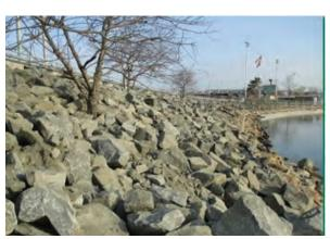
FIGURE 17: RESTORED ABUTMENT AT CROSS BAY BRIDGE
