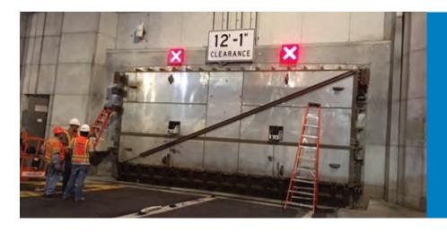
FIGURE 13: PORTAL FLOOD GATE AT HLCT MANHATTAN WEST IN CLOSED POSITION
